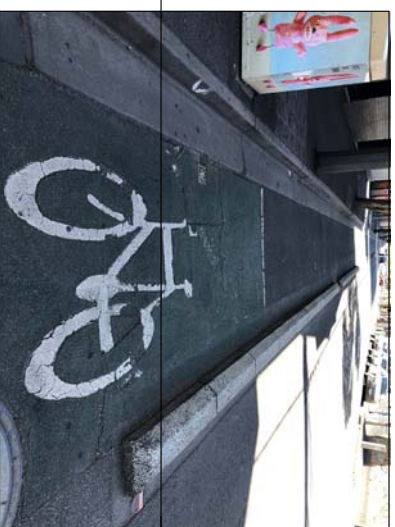
TYPICAL BIKE TRAFFIC KERB SEPARATOR
