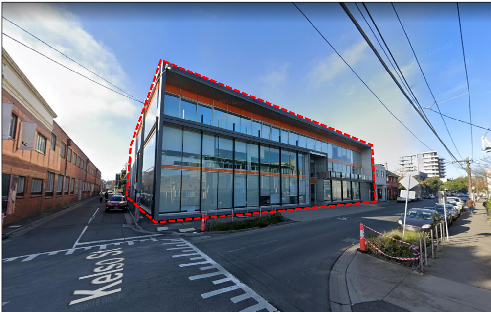
Figure 2 – Subject Site – existing under developed condition. (December, 2019).
