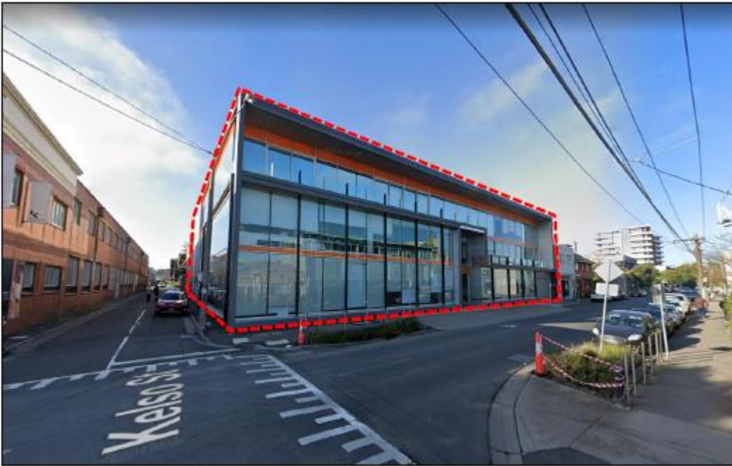
Figure 2 – Subject Site – existing under developed condition. (December, 2019).
