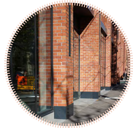
DESIGN BENCHMARK Constructed example of brickwork "Craftworks" 20-30 Mollison St Abbotsford
