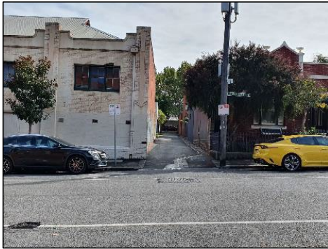
Figure 13: St Crispin Street – View North
