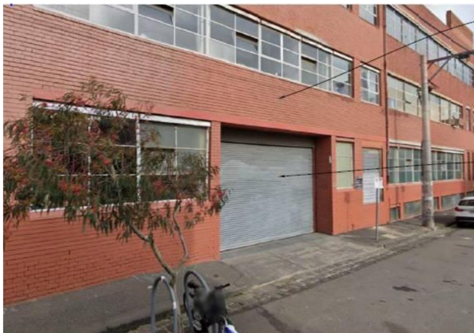
Above: Existing opening
