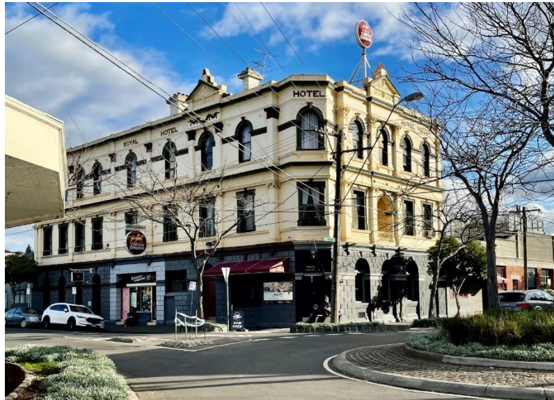
Image 1: The subject site as viewed from the intersection of Spensley and Berry Streets.
