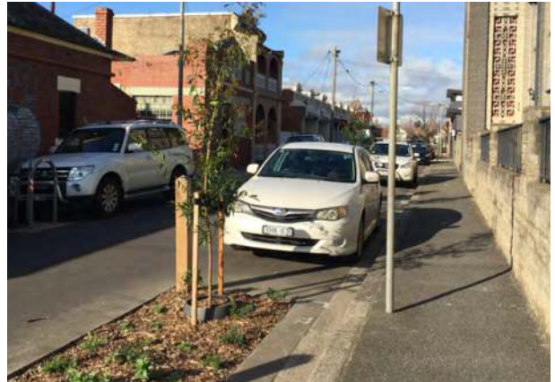
Flush cut garden beds appropriately placed in between car parking bays and protected by corner tree.
