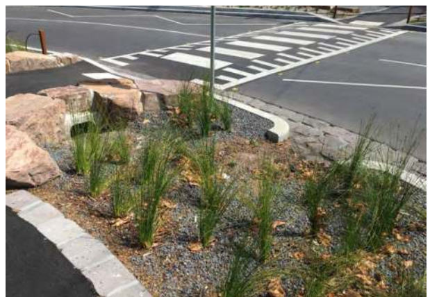
New crossing incorporates WSUD and high quality materials to improve amenity and performance of space.
