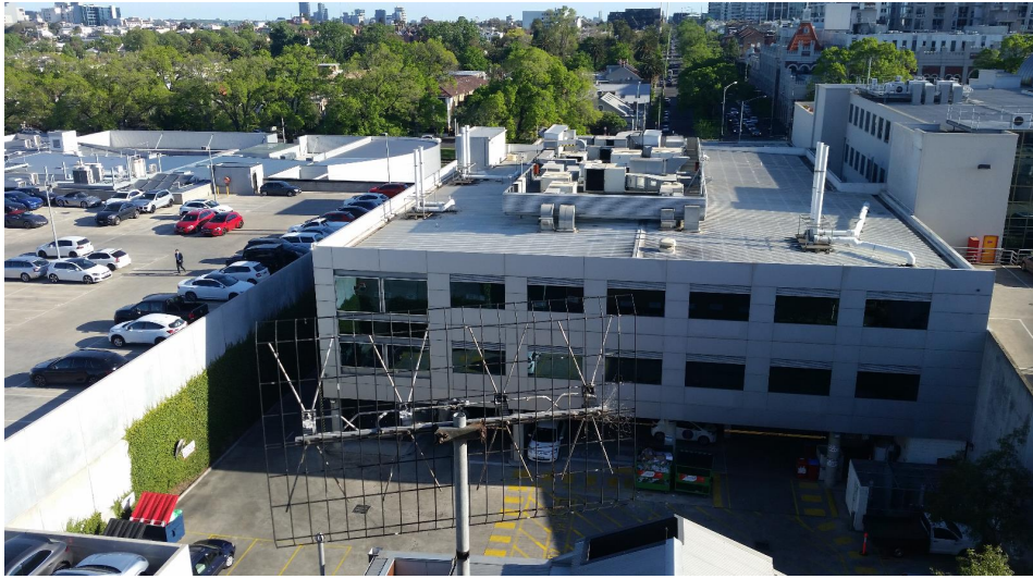
Location 5 – (Roof terrace balcony Brick Stack Vent) View to Melbourne Pathology Building Plant noise not audible above general background level
