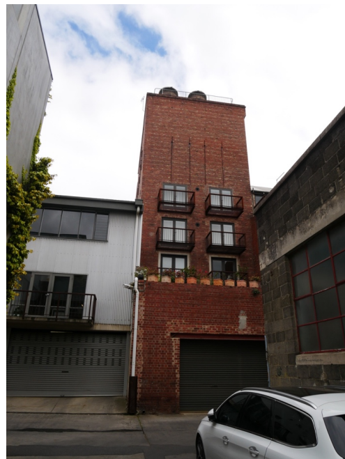
Figure 15. View west along Byron Street
