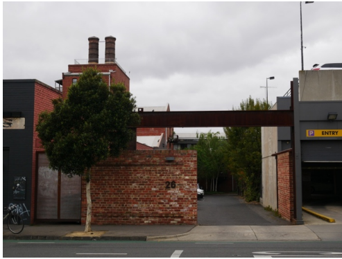
Figure 6. Wellington Street entrance
