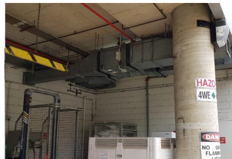
Four exhaust fans within Melbourne Pathology under croft as indicated in area in above photo
