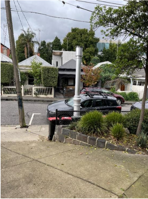
Figure 2: Cubitt St Ramp.
