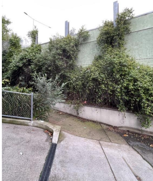
Figure 3: Dover St Entrance
