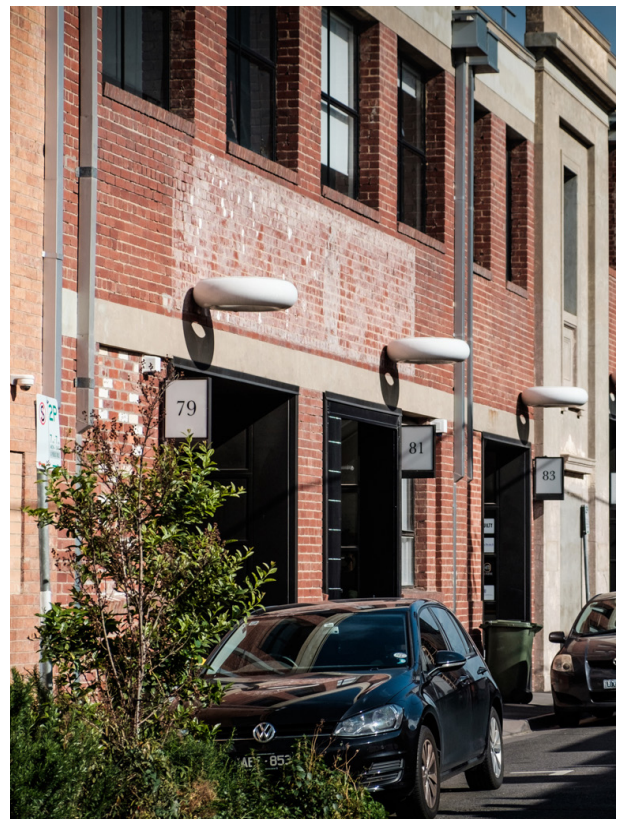
Image 9 - Warehouses converted to commercial tenancies
