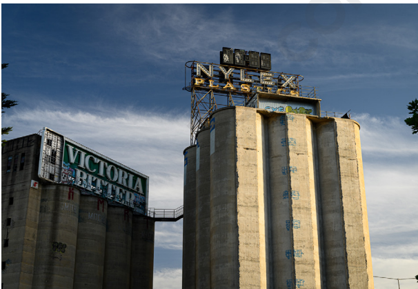
Image 15 - Nylex Sign and Silos at Richmond Maltings
