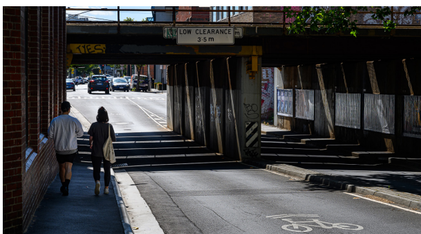
Image 22 - Balmain Street underpass
