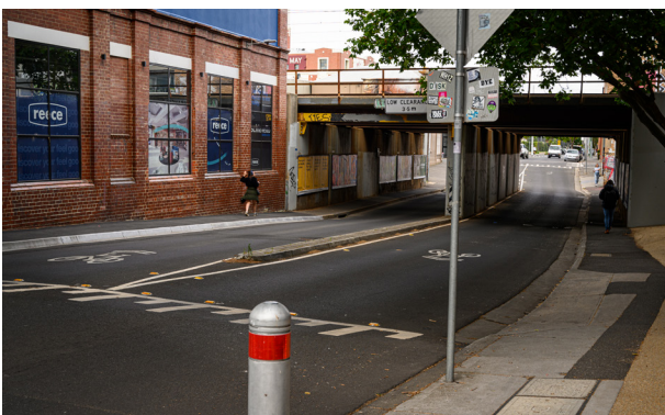
Image 25 - Balmain Street rail underpass
