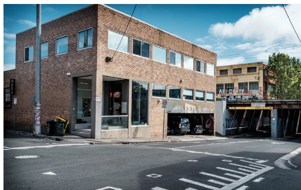
Image 77 - Balmain Street underpass looking west
