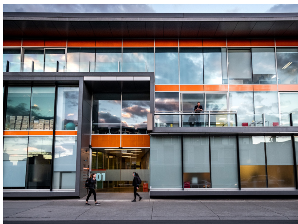
Image 13 - Commercial buildings on Cremorne Street
