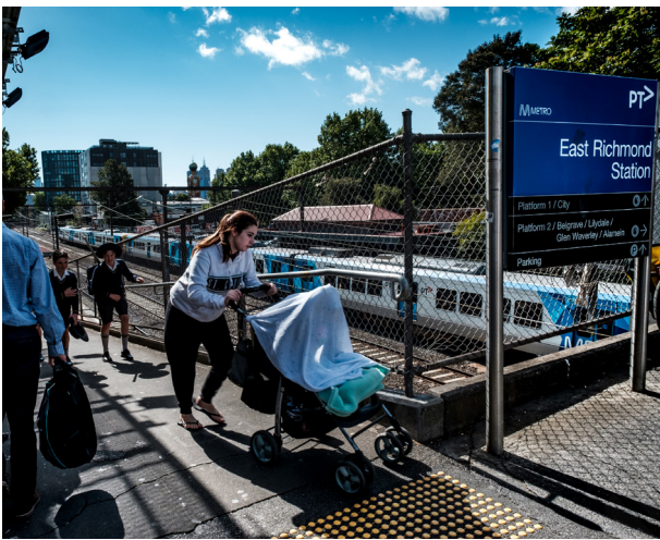
Image 20 - East Richmond Station entrance ramp
