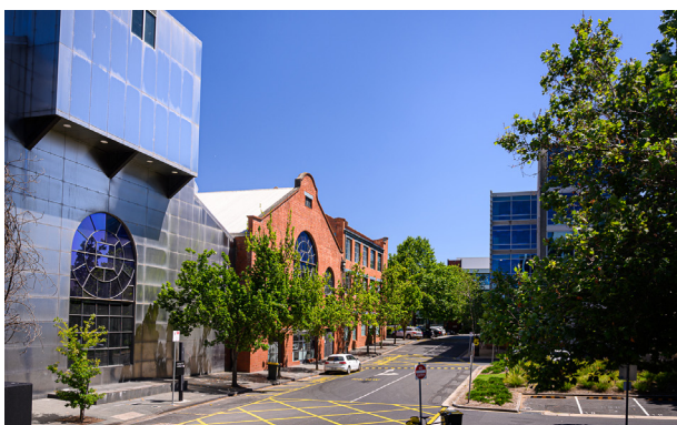
Image 71 - 658 Church Street - Former Power Station
