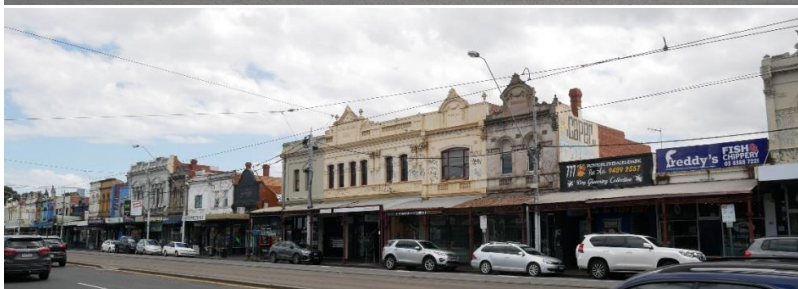
Figure 12. Similar view looking southwest.
