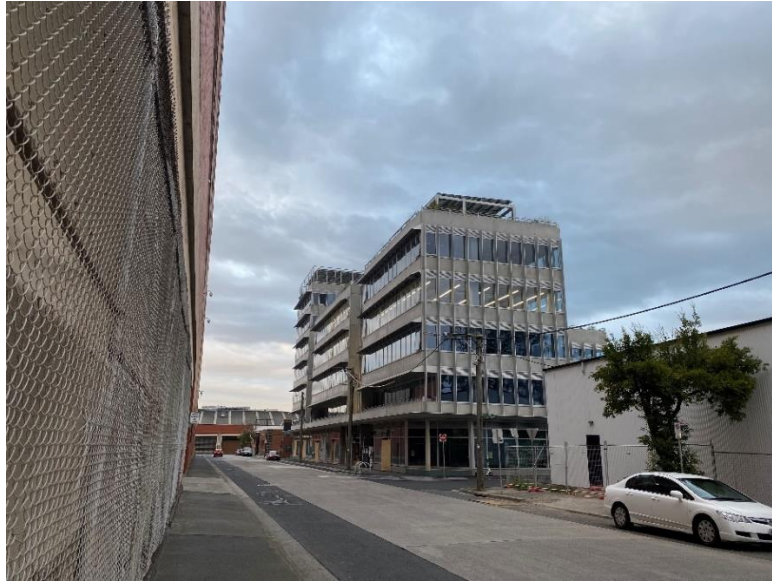
Image – Subject site No. 31-51 Nelson St, Abbotsford - View from west of Nelson Street (Source: Officer inspection – Feb 2024)
