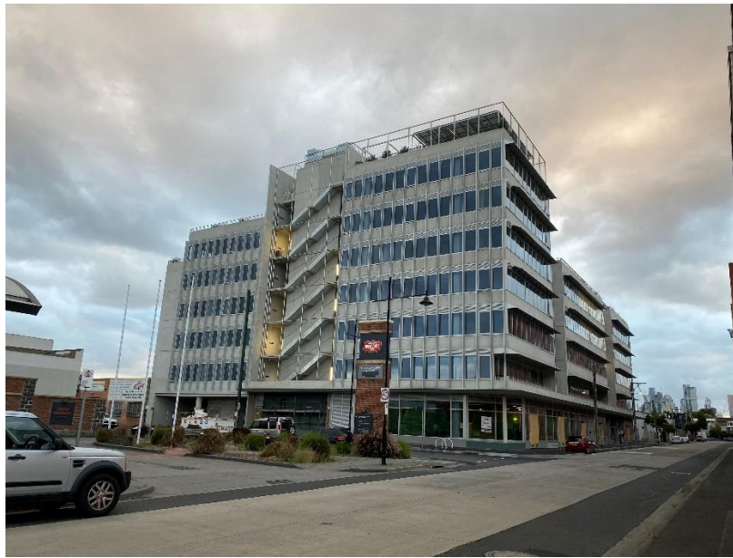
Image – Subject site No. 31-51 Nelson St, Abbotsford - View from east of Nelson Street (Source: Officer inspection – Feb 2024)
