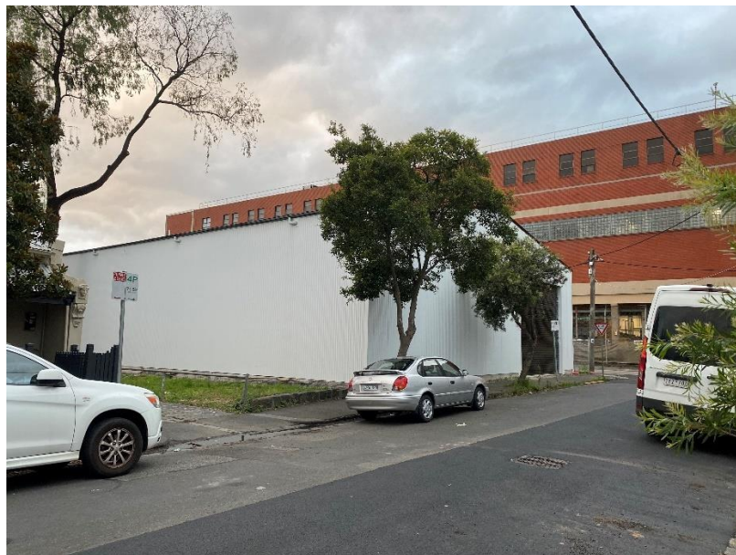
Image – 13-29 Nelson St, Abbotsford - (Source: Officer inspection – Feb 2024)
