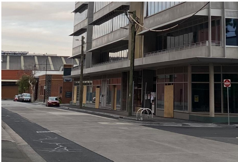
Image – Subject site entry to Nelson Street (Source: Officer inspection – Feb 2024)
