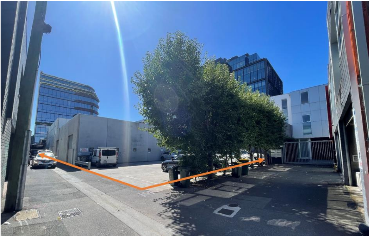
Image 12: the at-grade car park at the rear south-east corner of the site, with Sanders Place to the left and the private driveway and trees of No. 7 Sanders Place to the right (Officer site visit, February 2024)
