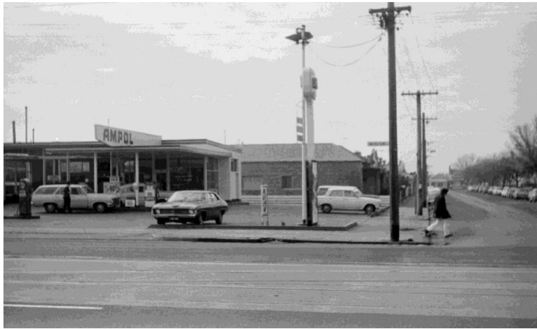
Figure 20. Ampol service station, c. 1970-1974, Committee for Urban Action photographic survey of Fitzroy. Source: State Library of Victoria
