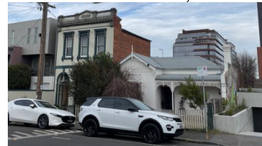
Brighton Street dwellings – east of the subject site
