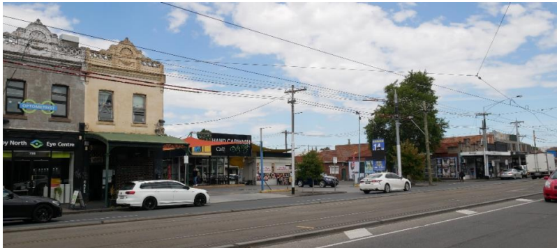
Figure 14. Looking southeast from the west side of Nicholson Street towards the subject site.
