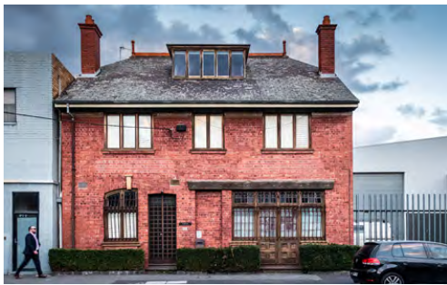
Image 67 - Former Yarra Hotel Cremorne Street
