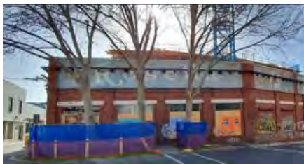
Figure 52. Current development site north of Balmain Street, Building 1. Source: Trethowan Architecture.
