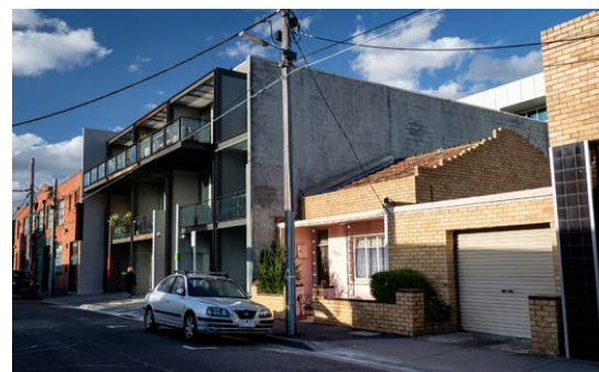
Image 37. An industrial-style commercial building alongside a single storey building with a residential typology.
