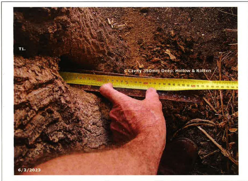
T1: Bole Cavity at Ground Level. Hollow & Rotten.
