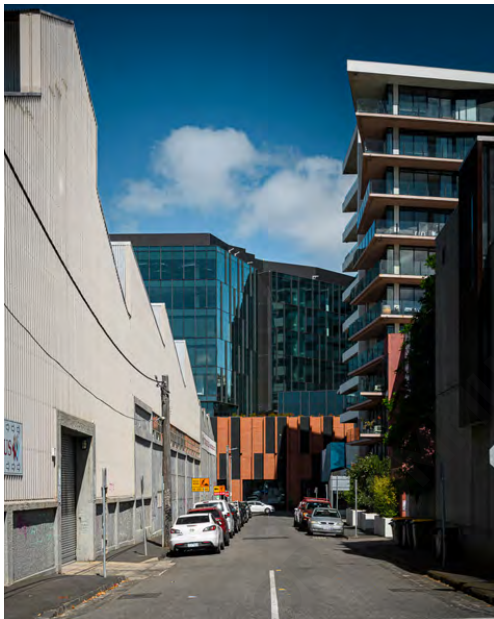
Image 83 - Bent Street existing warehouse
