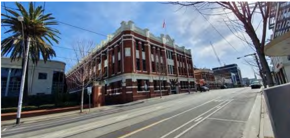
Figure 44. View of Bryant and May facade from the southeast, Church Street. Source: Trethowan Architecture.
