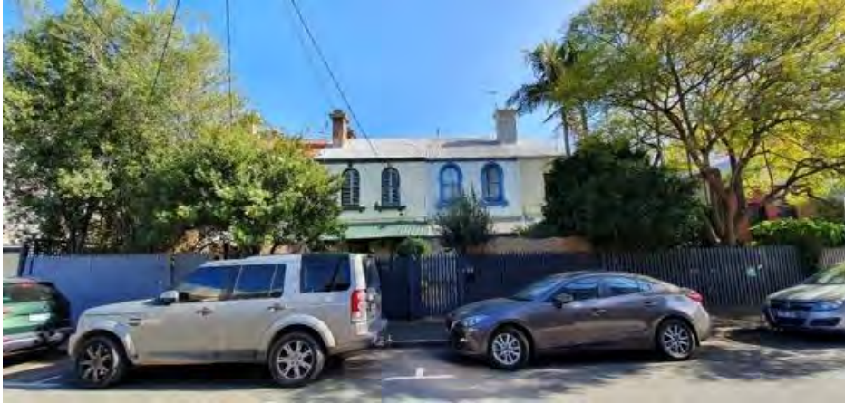
Figure 33. 30-38 Dover Street. Source: Trethowan Architecture.
