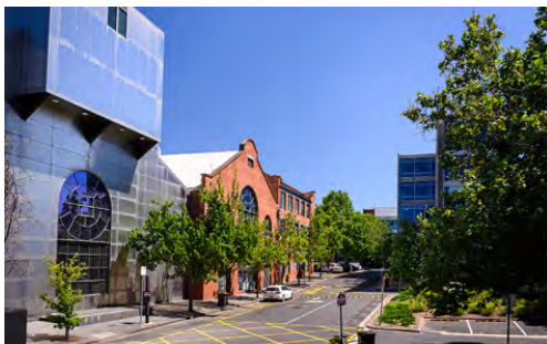
Image 71 - 658 Church Street - Former Power Station
