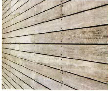
Timber Decking - Greyed Off
