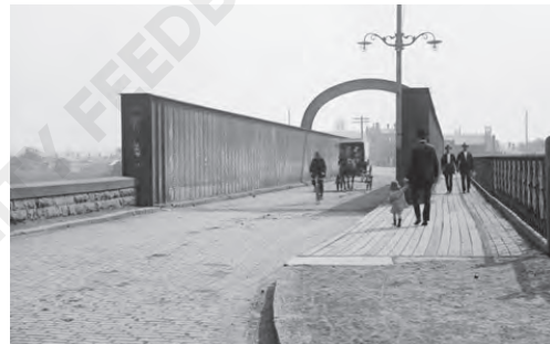
Image 4 - Church Street bridge (1914)
