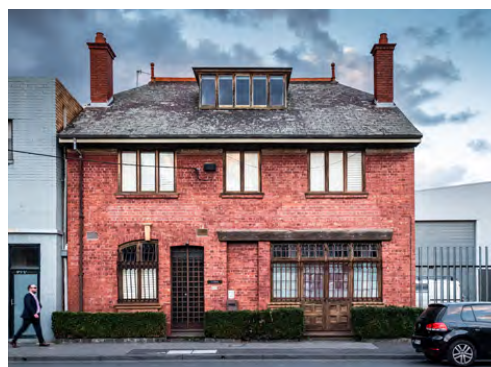
Image 76 - Former Yarra Hotel Cremorne Street
