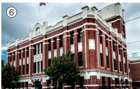
Image 27. Bryant and May building as viewed from Church Street.
