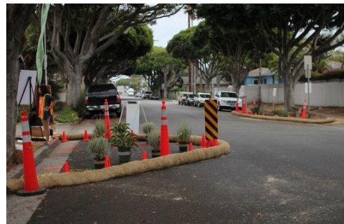
Figure 4.4 – Pinch point trial on a local street using sandbags to create the kerb build-out
