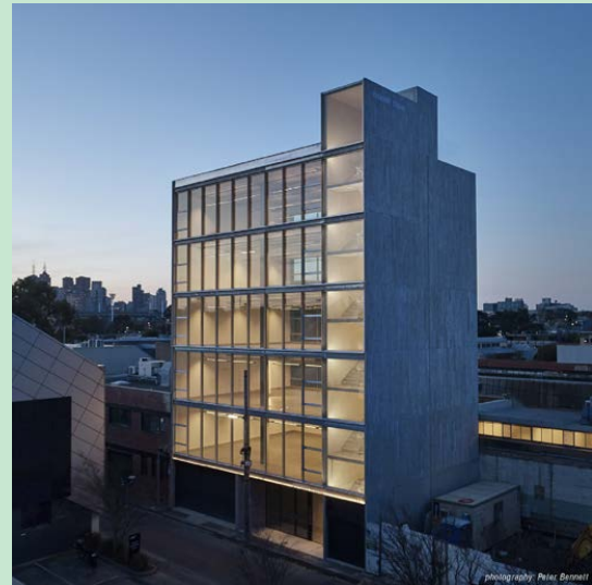
Figure 18. Elevated view of Cremorne Studios, photographed by Peter Bennett. Source: Layan Architecture.
