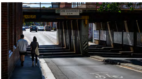
Image 22 - Balmain Street underpass
