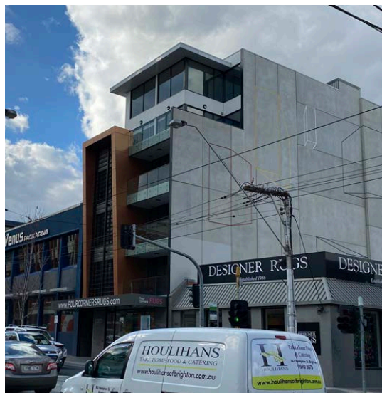
Figure 31. Buildings of between 1 and 6 storeys along Church Street.
