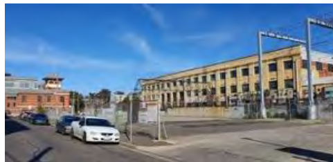
Figure 53. Rosella Factory and Power Station on either side of the railway line, looking southwest. Source: Trethowan Architecture.
