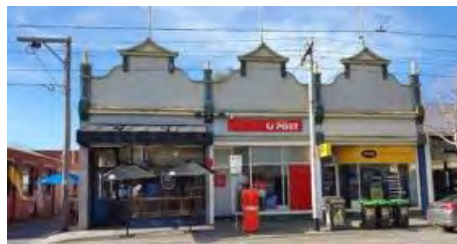
Figure 40. 533-537 Church Street. Source: Trethowan Architecture.
