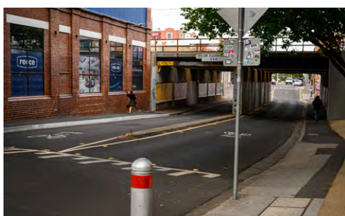
Image 25 - Balmain Street rail underpass
