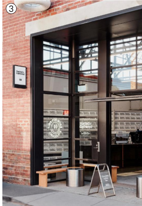
Image 18. Good example of an inset building entrance with integrated seating on Gwynne Street.
