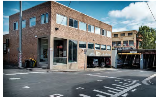
Image 77 - Balmain Street underpass looking west
