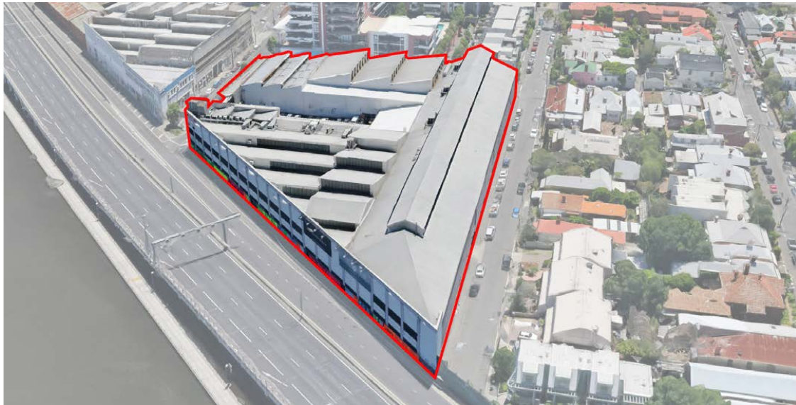
Figure 93. 167 Cremorne Street aerial
