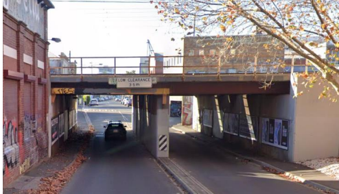
Figure 4.6 – Existing Balmain Street Underpass
