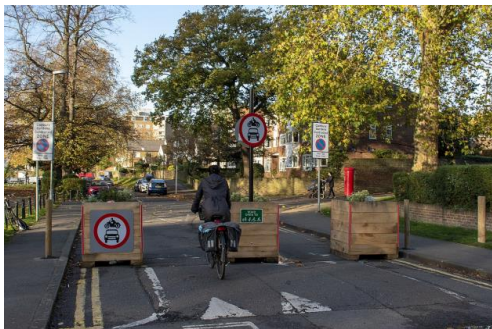
Figure 4.3 – Modal filter trial with pole-mounted signage anchored in planter boxes
