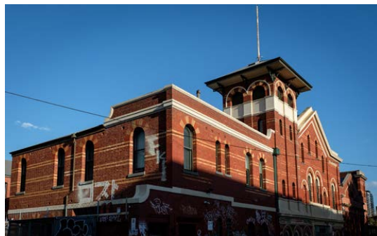
Image 9. A view of the Richmond Power Station on Green Street.
