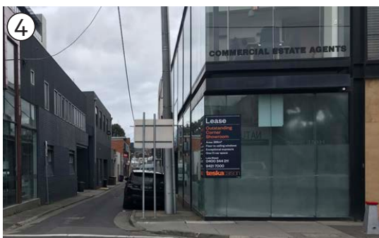
Image 19. Poor example of ground floor design on Church Street with floor to ceiling glazing and limited architectural detailing.
