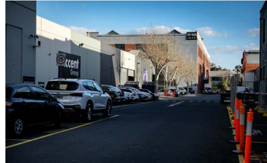
Image 47. Existing buildings within the Rosella Complex looking south along Palmer Parade.
