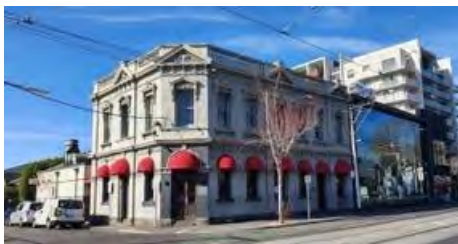
Figure 39. 619 Church Street. Source: Trethowan Architecture.
