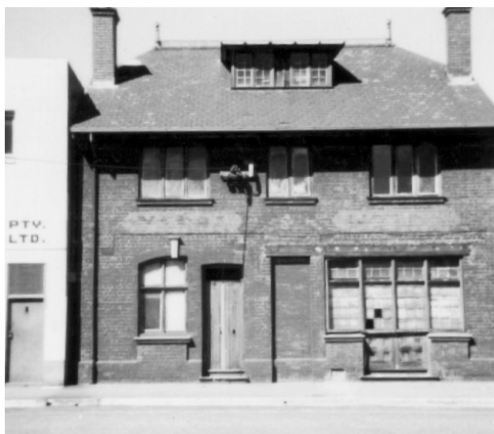
Image 5 - Former Yarra Hotel (Cremorne Street)
