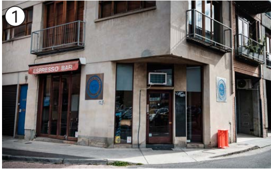
Image 16. Example of a chamfered building corner at the intersection of Kelso Street which has the benefit of creating additional public space at the entrance to the building and at the intersection.
