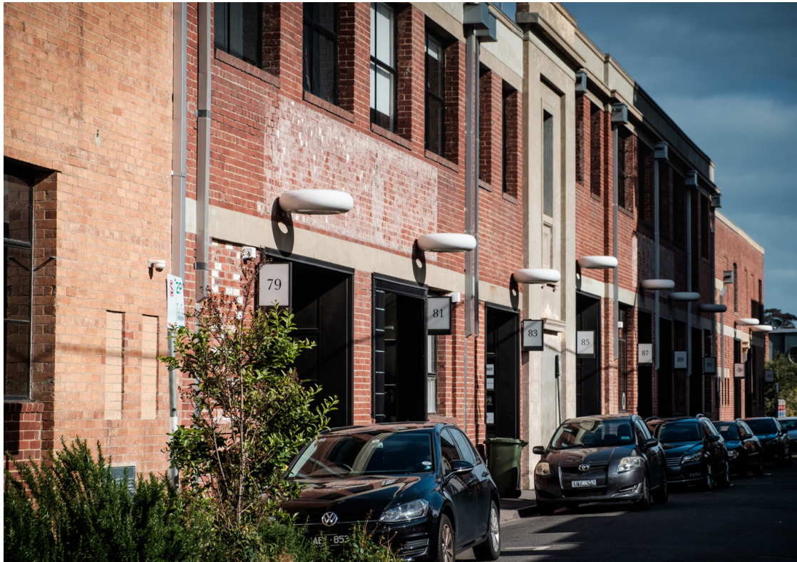
Image 1. Typical industrial buildings found in Cremorne.
