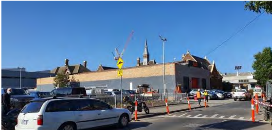
Figure 21. View from the north, note warehouse abutting the former state school building. Source: Trethowan Architecture.
