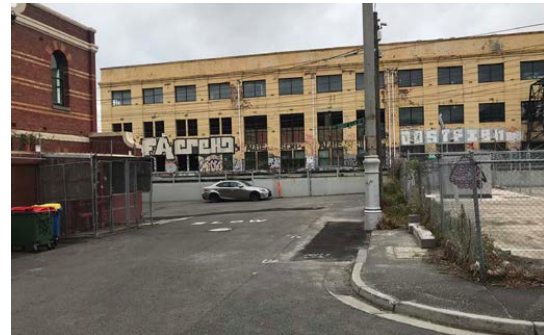
Image 35. Looking across the railway line towards the Rosella Complex from the intersection of Electric Street and Oddy's Lane. Richmond Power Station to the left.
