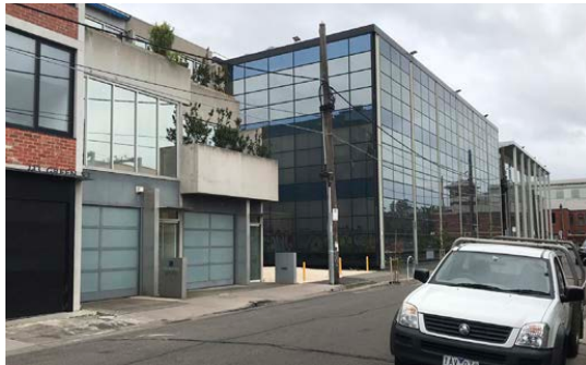
Image 34. Looking south along Green Street at a mixed typology of buildings.
