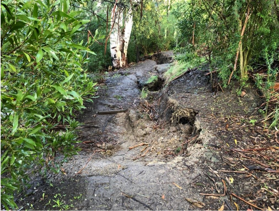
Tree T1 on and related bank slump 12 August 2019
