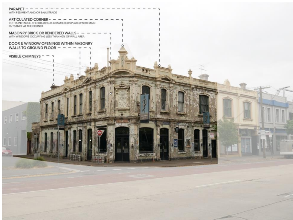
Figure 36: Corner hotel / commercial building (Prince Patrick Hotel, corner Victoria Parade and Rokeby Street, HO138)
