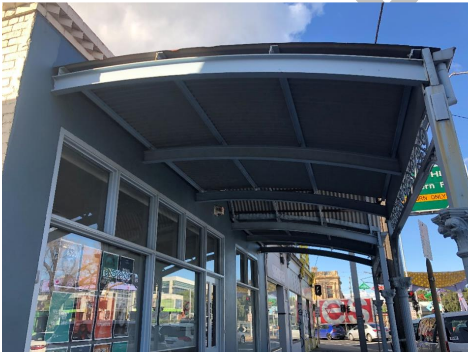
Figure 7. Looking east to the canopy at 211-213, showing later steel structure above cast iron verandah posts.
