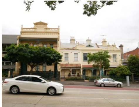
Figure 22: (left ) Intersection of Victoria Parade and Smith Street looking northeast
