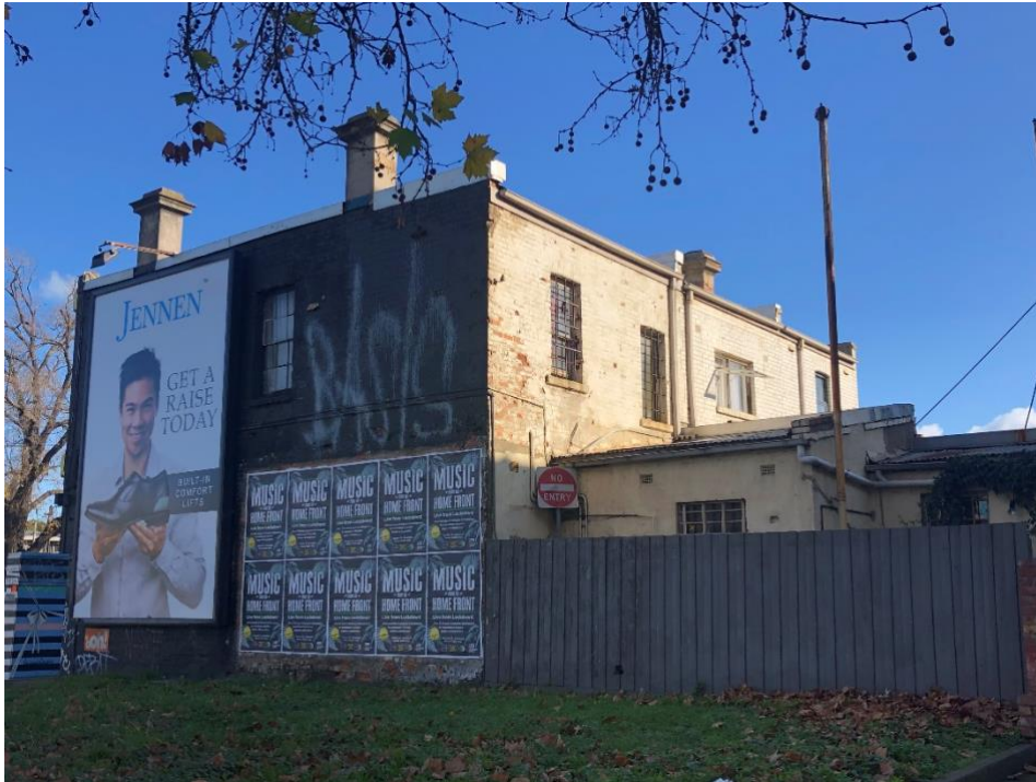
Figure 8. Looking southwest to the rear of 215-219 Victoria Parade, showing extant chimneys to the east elevation and single-storey outbuildings (at right).
