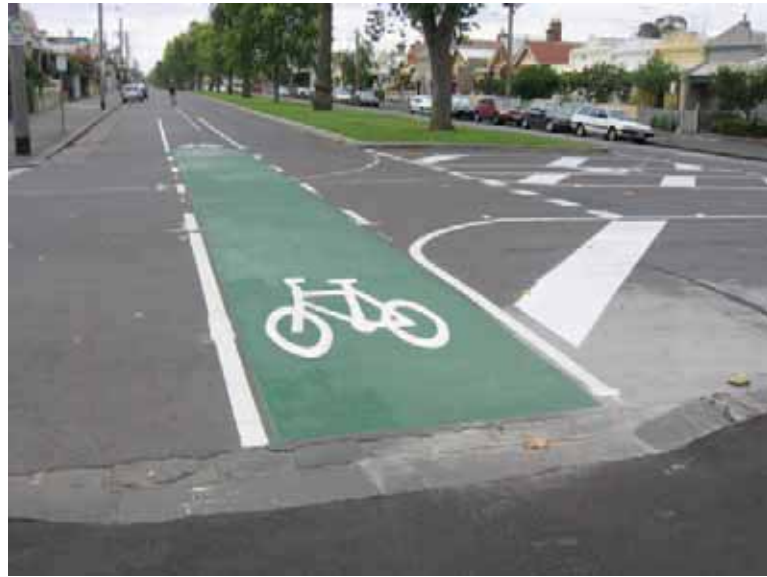
Figure 5.1.1 (a) Canning Street, North Carlton
