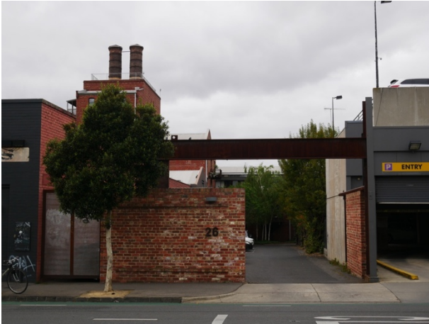
Figure 6. Wellington Street entrance
