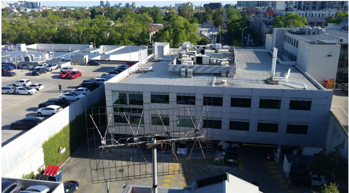
Location 5 – (Roof terrace balcony Brick Stack Vent) View to Melbourne Pathology Building Plant noise not audible above general background level
