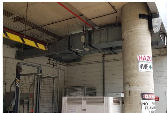
Four exhaust fans within Melbourne Pathology under croft as indicated in area in above photo
