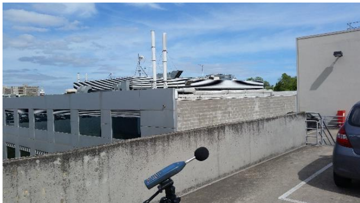
Measurement location 3 - Melbourne Ppathology roof plant
