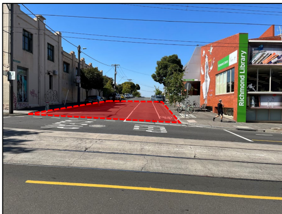
Figure 1: Charlotte Street – View East from Church Street
