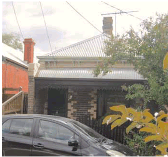
Figure 2 58 Stafford Street, Abbotsford (identified as a contributory building in the extended HO313 precinct)
