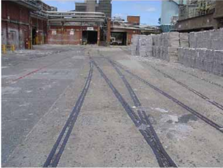
Remnants of railway sidings
