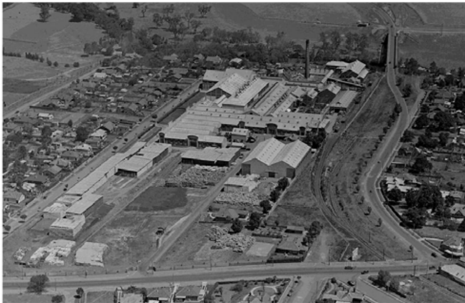
Figure 8 c. 1936 Airspy oblique aerial showing additional buildings along eastern boundary (Latrobe Avenue) and double gabled building along railway siding. Note Chandler Highway open to cars. North is at the bottom of the image. Source: Airspy, State Library of Victoria
