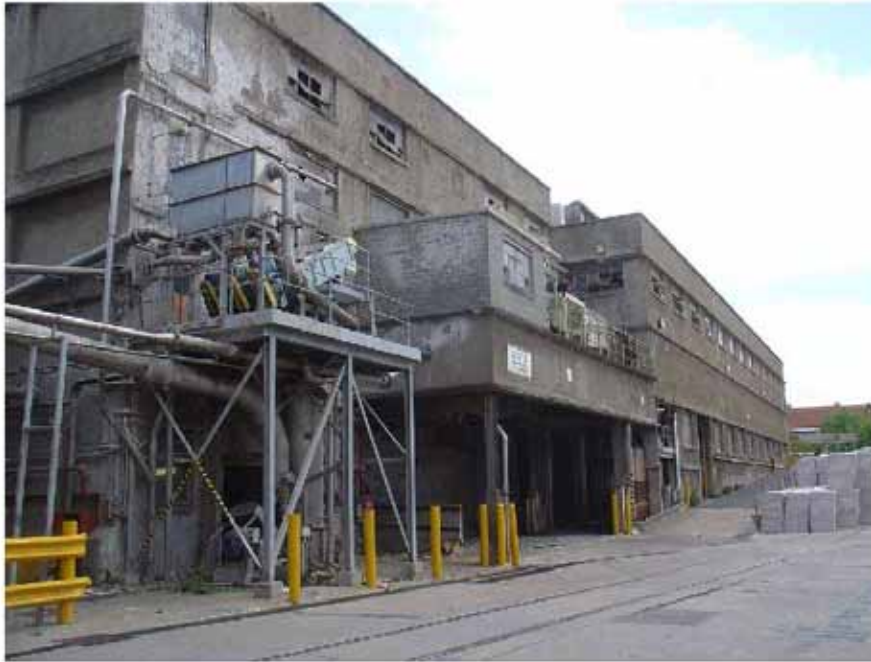
Rear of Chandler Highway Building
