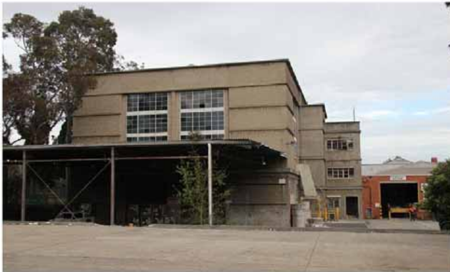
Figure 2 The north end of the F5/ FRC building showing the unfinished outer skin.
