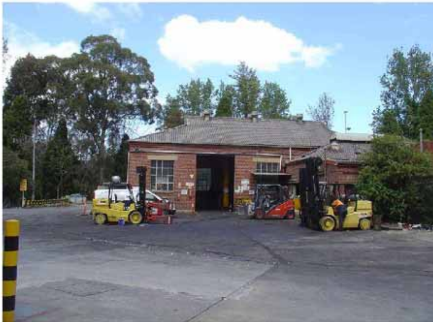
Garage and Switchyard (probable original power house)
