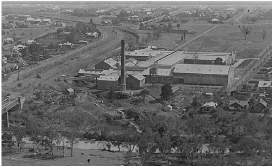
Figure 6 1920s Airspy oblique aerial of mill, with rail bridge and Yarra River in foreground. Source: State Library of Victoria.
