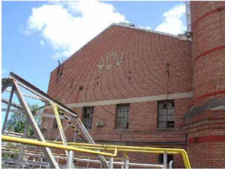
North wall of original boiler house and chimney
