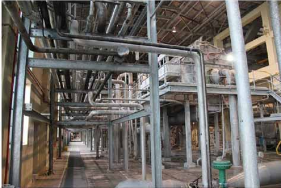
Figure 3 Interior view within the F5/ FRC building looking south
