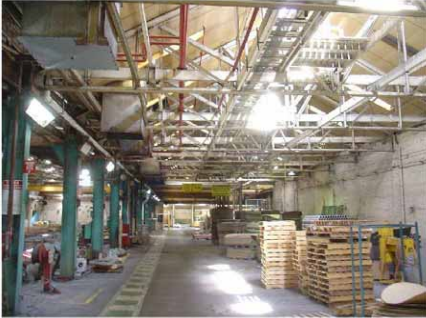
Timber trussed section in South Mill Building, probably c 1919.
