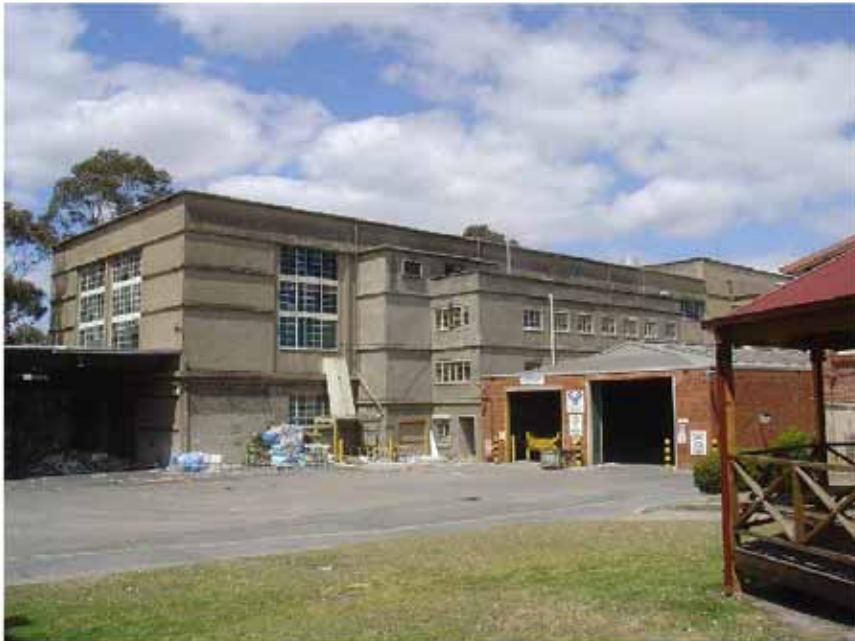
West side of Recycling Centre
