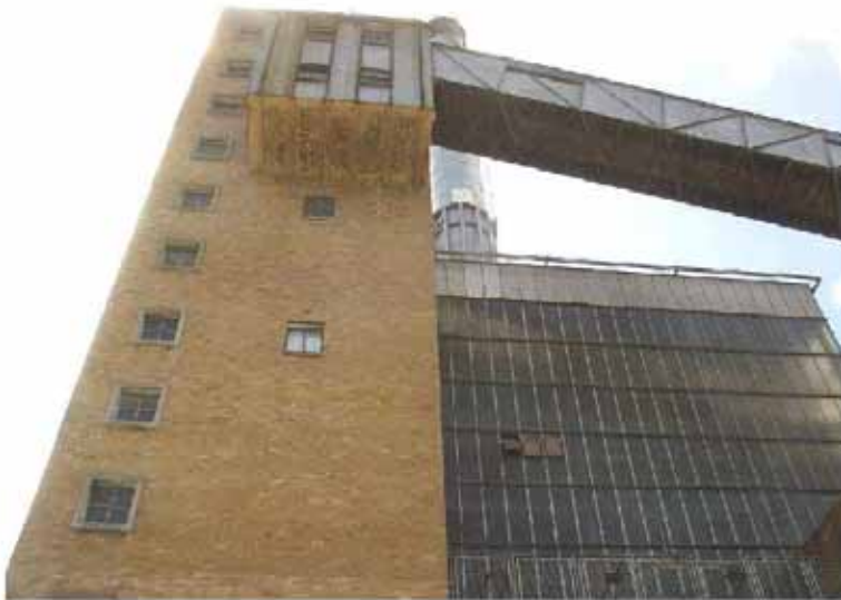
Boiler House showing coal elevator
