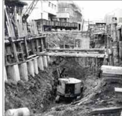
Figure 19 Coal Tippler construction 1952 Source: Source: Contamination Plan , GHD, 2003, Appendix C
