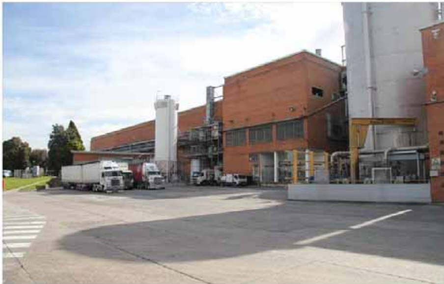
Figure 4 Internal view of the south side of the F6 building
