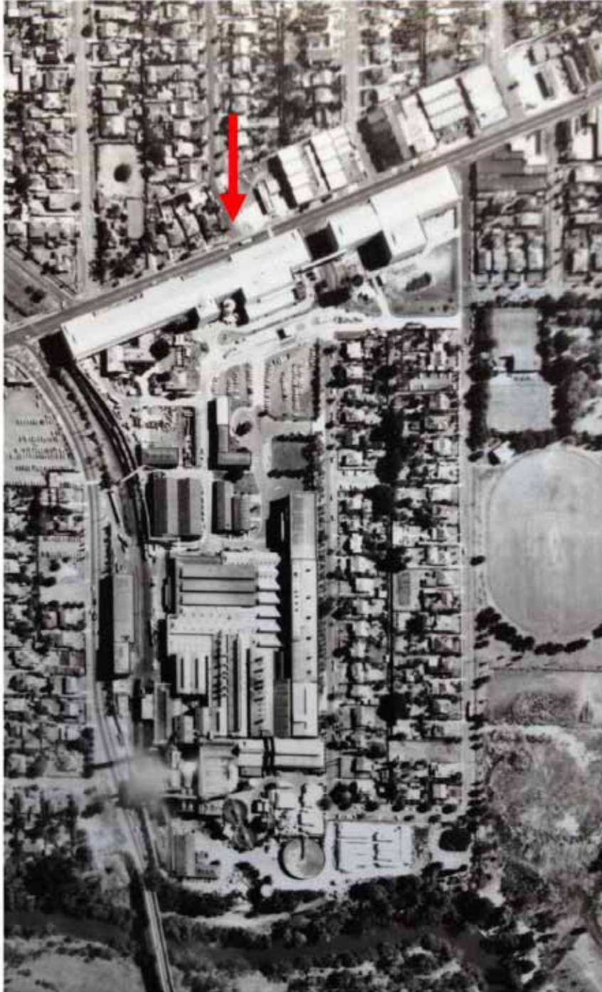
Figure 14 1968 aerial image showing the newly constructed No. 6 Machine buildings along Heidelberg Road. Source: Laverton Aerials, Land Victoria.
