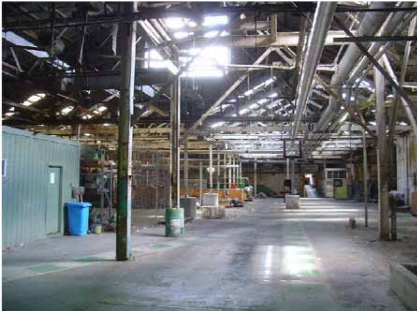
Steel truss roofed section of South Mill – c later 1920s.
