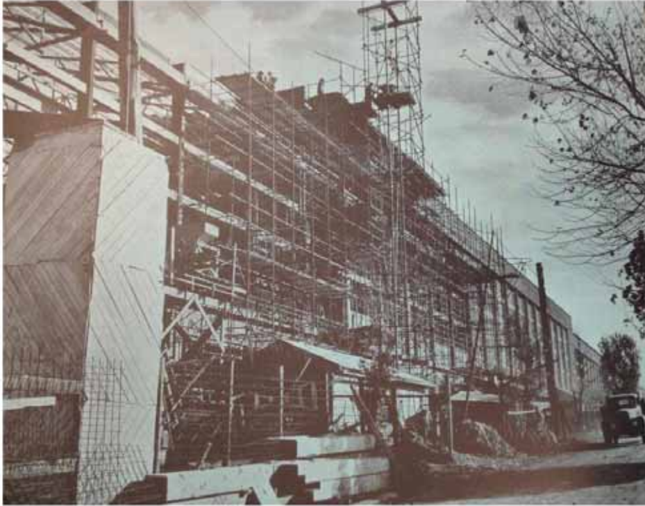
Figure 10 No. 5 Building during construction, c. 1950. Source: APM Annual Report, 1952, Amcor archives.
