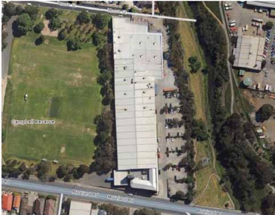
Figure 24 Recent aerial of the former Spicers Paper Mills complex, Coburg. Source: Nearmap.
