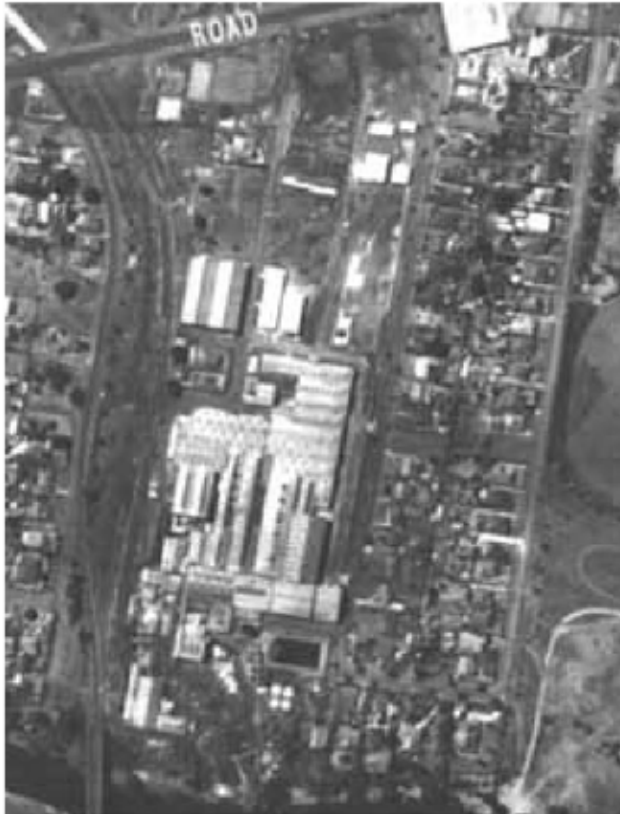
Aerial view showing extent of site and railway sidings c 1945, Melbourne University Library
