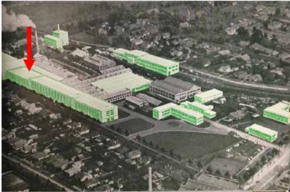
Figure 11 Expansion of Fairfield Mill site, 1950. No. 5 building indicated. Source: APM Annual Report, Amcor archives.
