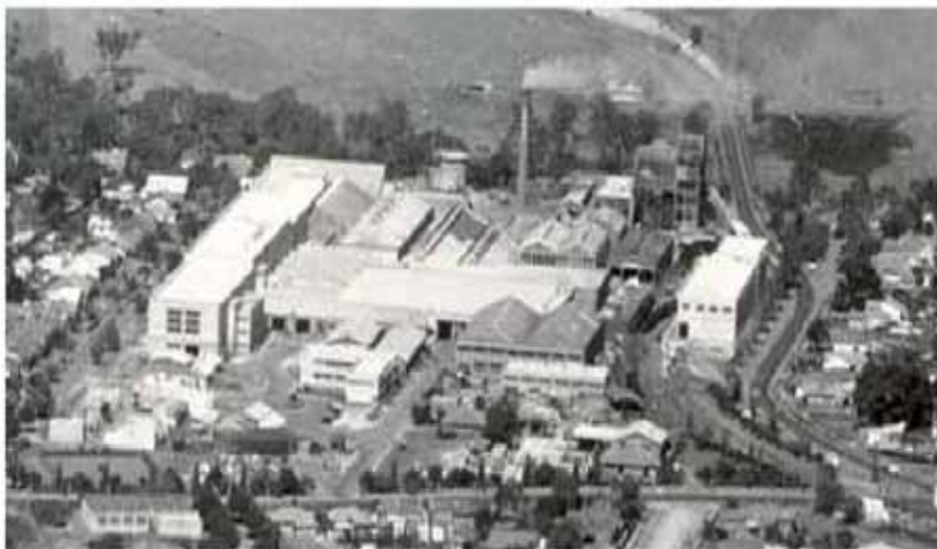
Aerial View c1950s, – note new boiler house under construction, .Darebin Historical Encyclopaedia
