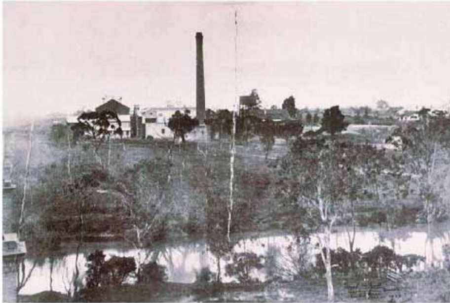
View from rail bridge shortly after construction of Paper Mill Darebin Historical Encyclopaedia
