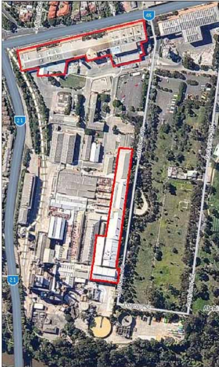
Figure 7 The F6 (northernmost) and FRC (easternmost) buildings. It is proposed to remove part of the roof structures within the red lines.
