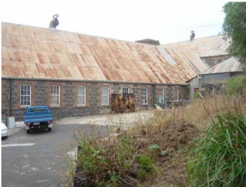
Figure 26 Barwon Paper Mills Complex, Fyansford.
