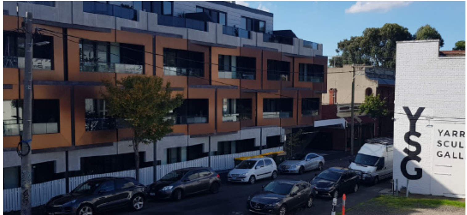
Existing apartment development - 114 Vere Street
