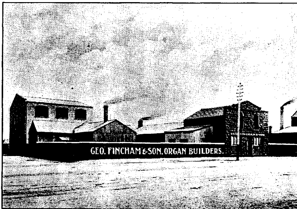
Figure 32 George Fincham & Sons premises, Richmond, c.1903. Source: The Cyclopedia of Victoria
