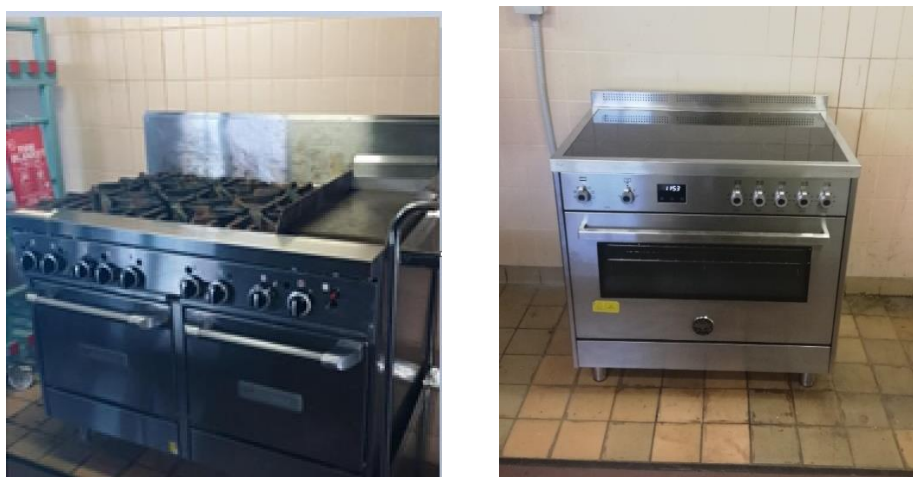
Figure 13 - Example of an action towards going all electric at our smaller sites - replacement of a gas stove to electric induction at the Richmond Senior Citizens Centre (April 2021)
