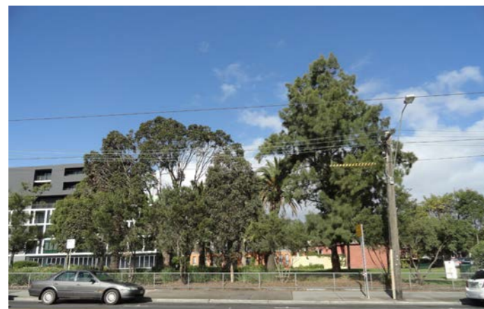
Williams Reserve: Existing Conditions
