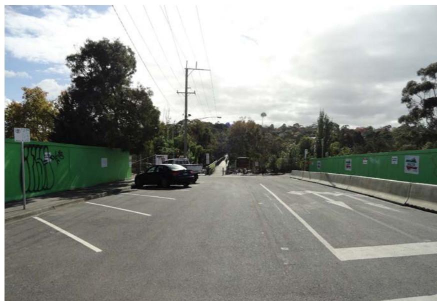
Walmer Street: Existing Conditions
