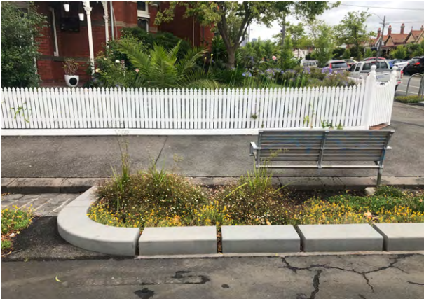
New garden bed in the road space includes slotted kerbing to help capture runoff.
