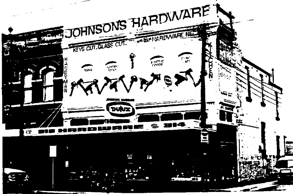
Fig. 4.71 314, 316 Bridge Rd., 1984. Replacement of the shopfronts, the verandah and the defacing signs have detracted from the original appearance.
