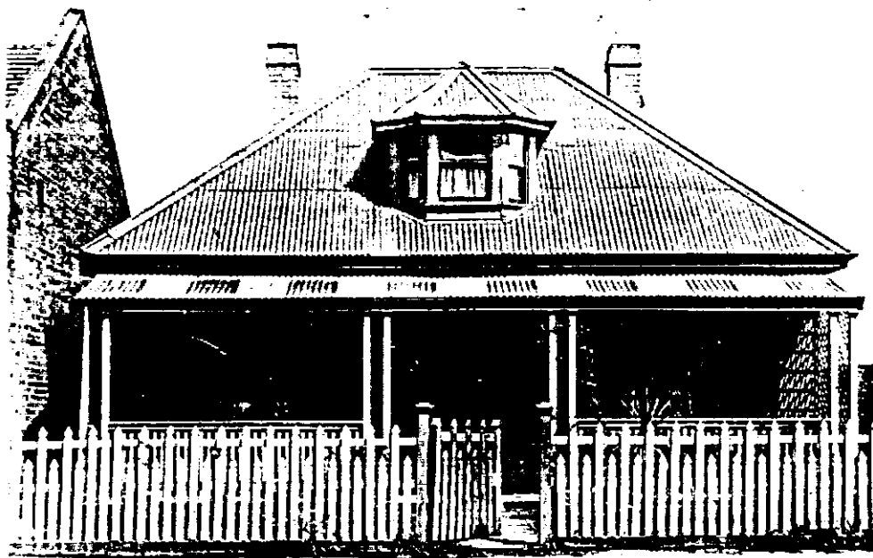
Fig. 6.13 1840's Prefabricated House, formerly on the site of St. Ignatius, Church Street
