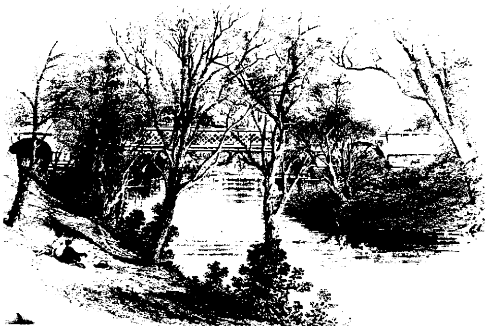
Fig. 6.83 The riverbank and Hawthorn railway bridge, 1862
