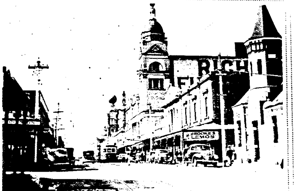
Fig. 6.59 Swan Street looking east, 1940's
