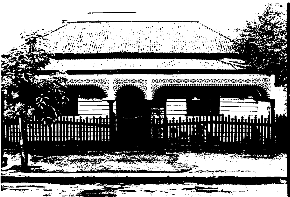
Fig. 4.51 Victorian fence, 41 Shelley St.
