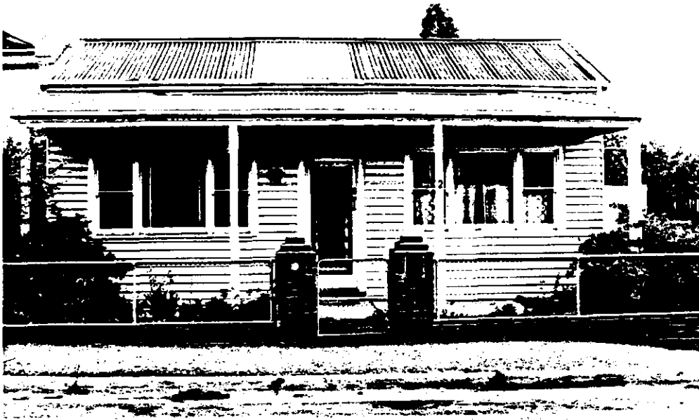
Fig. 4.41 Unsuitable Windows and Doors detract from original character of cottage.
