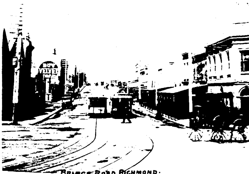
Fig. 6.42 Bridge Road looking east from Punt Road, 1890's
