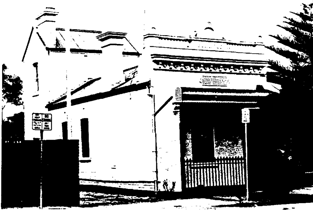
Fig. 4.26 VISIBLE REAR ADDITION DEFINITION 185 Burnley St.
