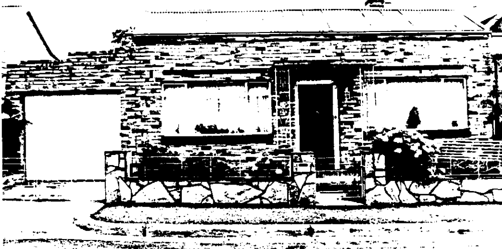
Fig. 4.39 Inappropriate cladding on a Victorian cottage.
