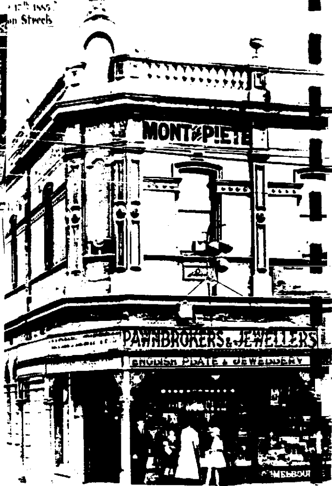
Fig. 4.73 Cast Iron Verandah on late Victorian Shop, 138 Swan Street.
