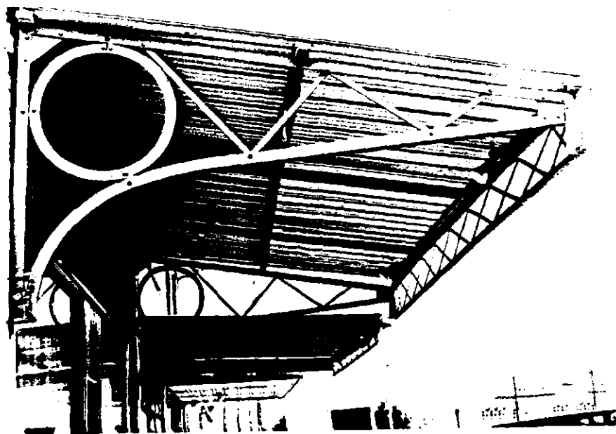
Fig. 4.83 Edwardian Cantilever Brackets, 144 Stawell St.
