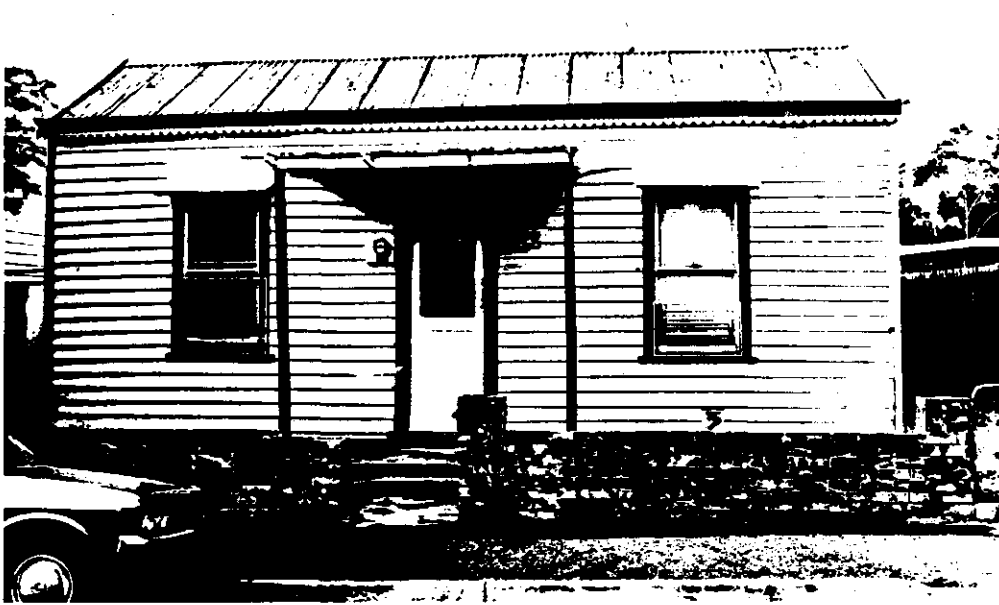
Fig. 4.45 Unsuitable verandah detracts from cottage's character
