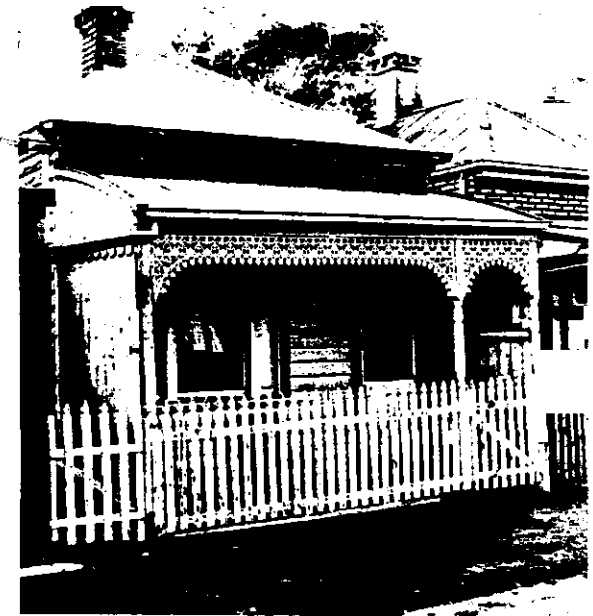
Fig. 4.9 Typical late Victorian Cottage, 87 Stawell St.
