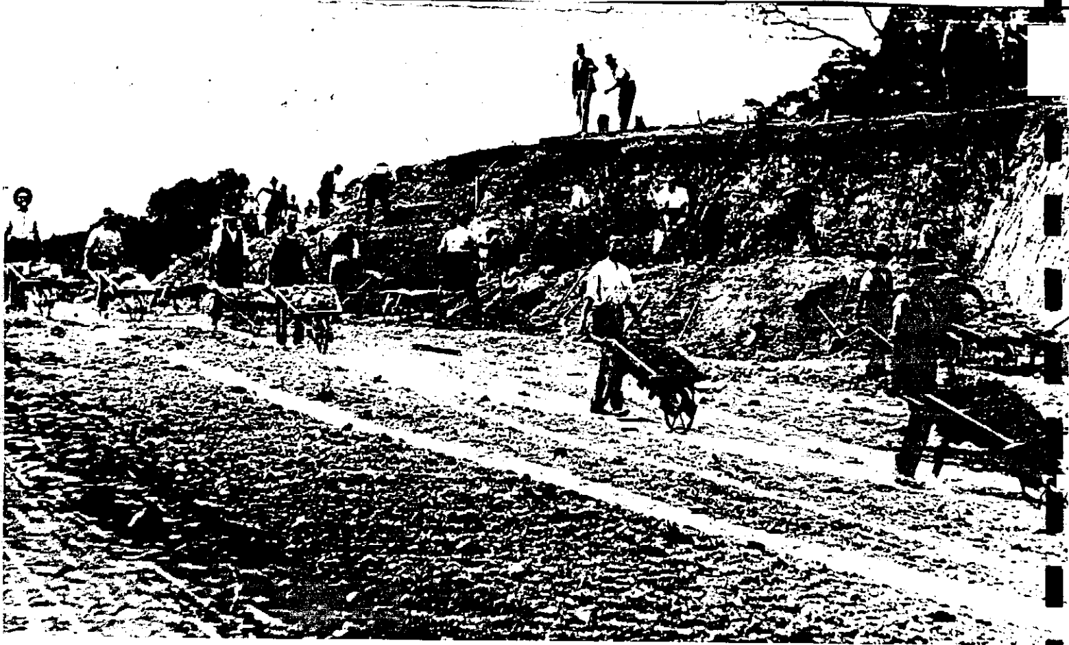
Fig. 6.93 'Sustenance' workers constructing the Yarra Boulevard, c. 1932
