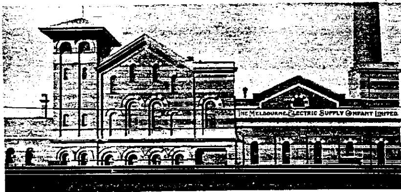
Front Elevation c. 1913. (The Story of Richmond Power Station, unpublished notes held by the S.E.C.)
