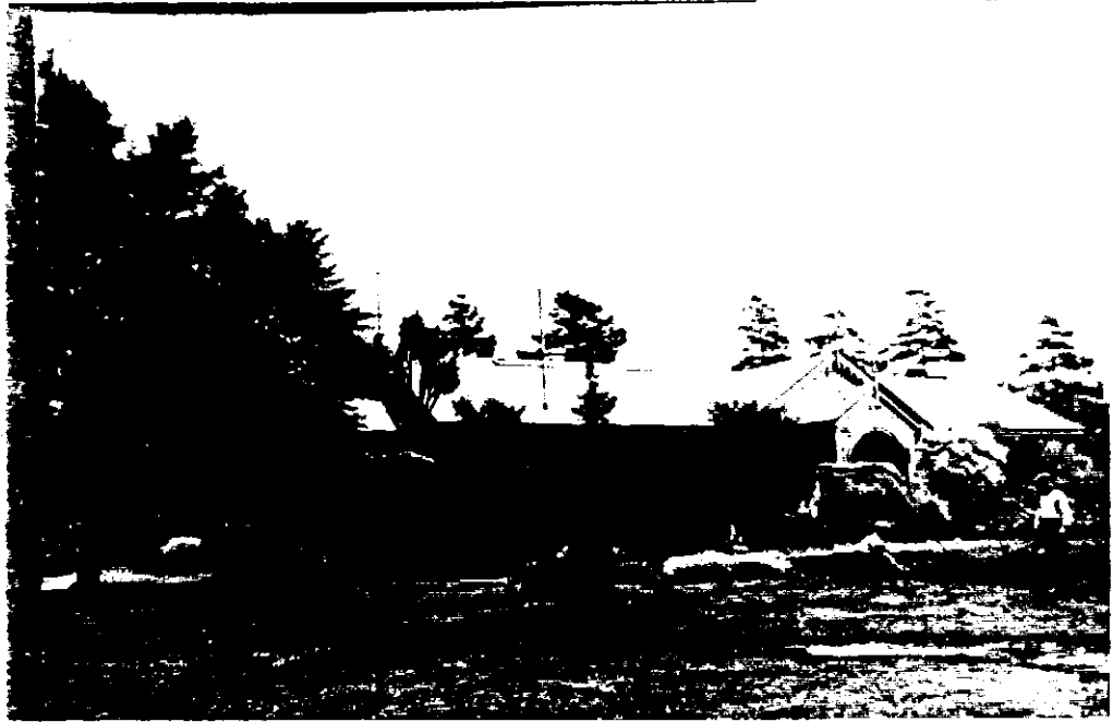
Fig. 6.84 Horticultural Society of Victoria's exhibition pavilion, c. 1890 (demolished)
