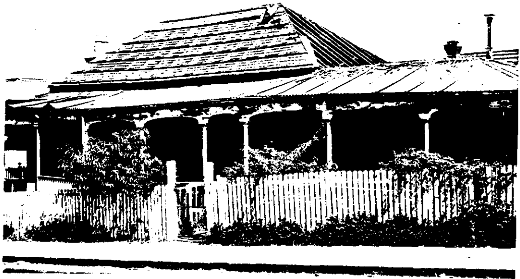
Fig. 6.5 Alexander McCrae's prefabricated timber house, cnr. Sherwood and Rotherwood Streets, during demolition, 1970's
