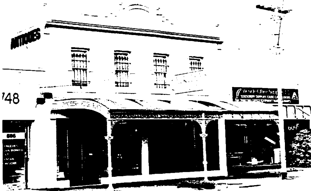
Fig. 4.78 Reconstructed Verandah 597, 599 Bridge Rd.
