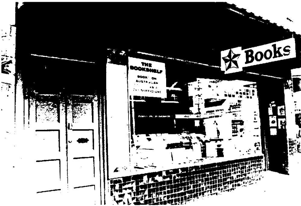
Fig. 4.97 Inter War Shopfront, 116 Bridge Rd.
