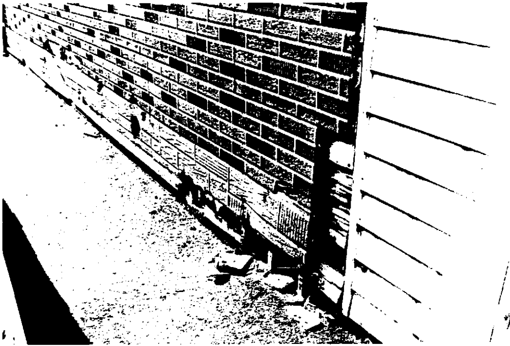
Fig. 4.38 Fake claddings often worsen existing problems.
