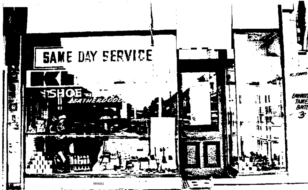
Fig. 4.92 Brass Edwardian Shopfront, 334 Bridge Rd.
