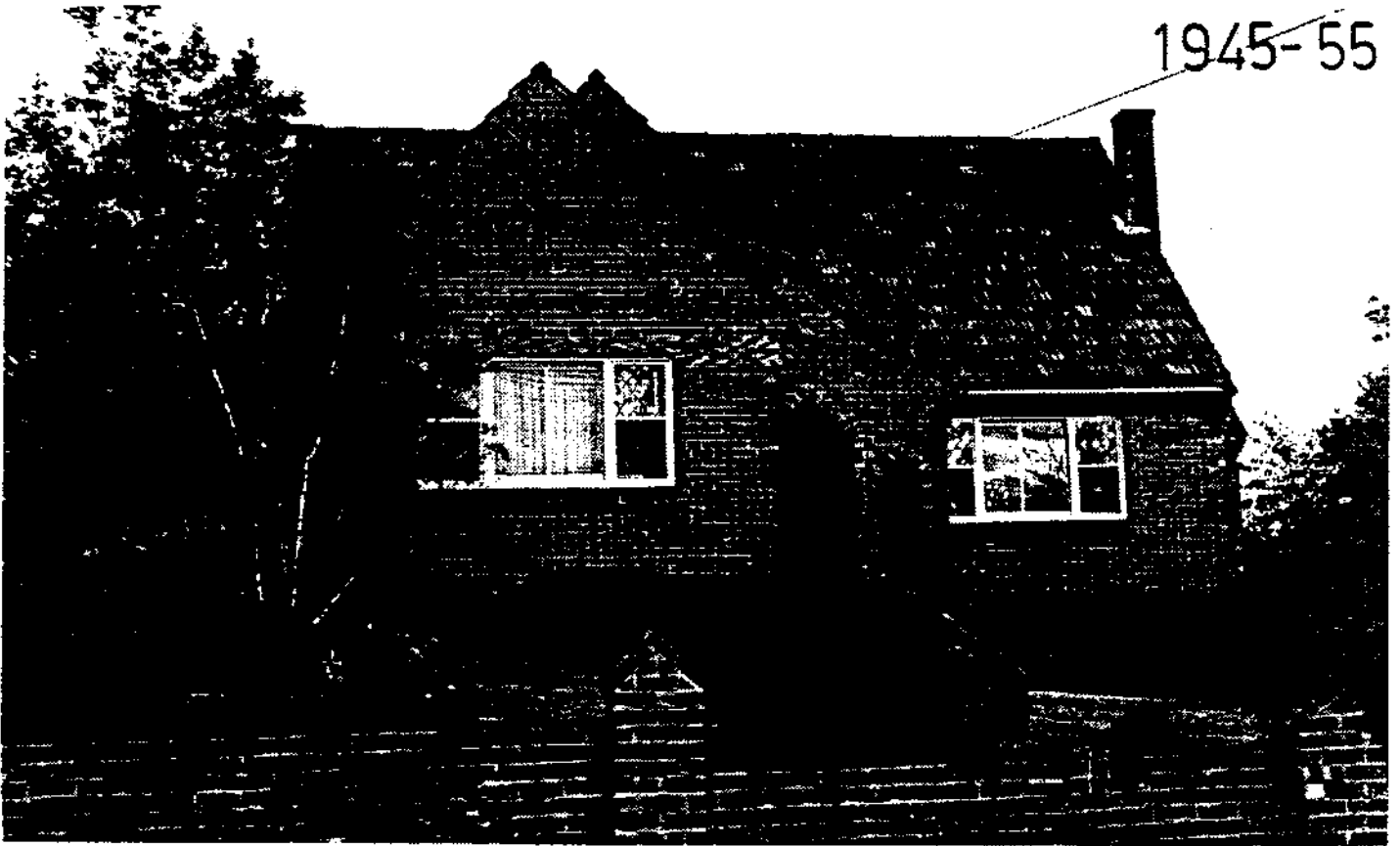
House, 115 Fyffe St, c1954 : the Tudor revival is evident with the gabled front, pointed arch openings and the fence to match. Again the wrought iron is evident and has spread to use as balustrading. Few flowering plants and neatly clipped hedges and topary are typical.
