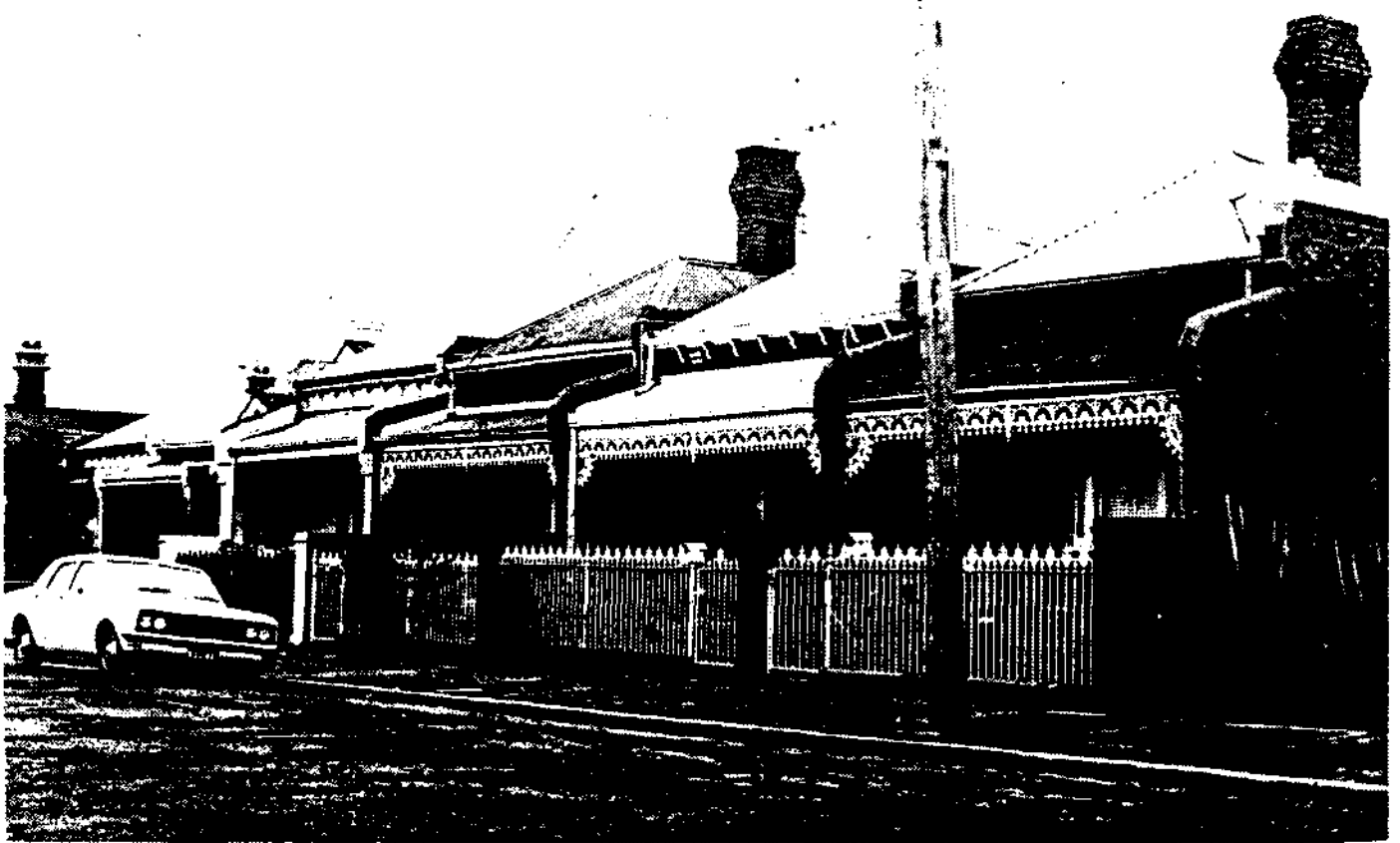
Rowhouses, 43-9 Charles St, c1900: one of few examples of a cast and wrought iron fence in Northcote, here placed on the typical chamfered edge basalt plinth and set between brick dividing walls.
