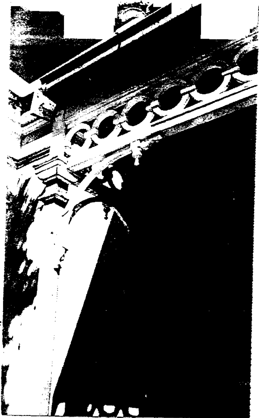
Verandah detail of 46 Bastings Street: indicates a similar tonal variation of paint colouring to 47 Cunningham St. This may have also been the case with Mayville.
