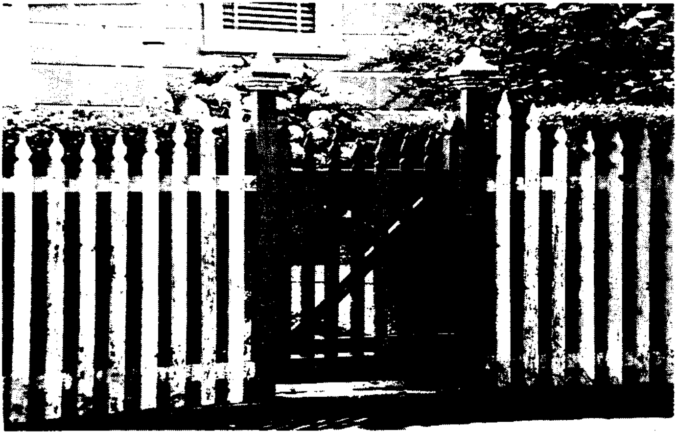
Detail, 39 Christmas St: spade-head pickets (c 70x20) spaced c35, height c +1200, posts 100x100, rail c45x80, plinth c100x40.
