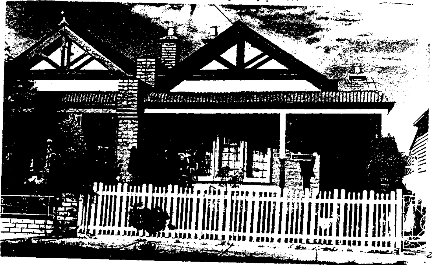
House, 24-6 Bridge St., c1910: pickets alternate as round versus square head which was to become more typical as was the two heights of picket.
