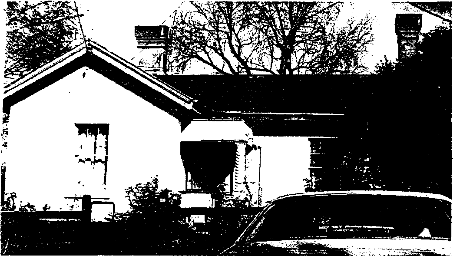
FORMER NORTHCOTE POLICE STATION, 24 WALKER STREET
