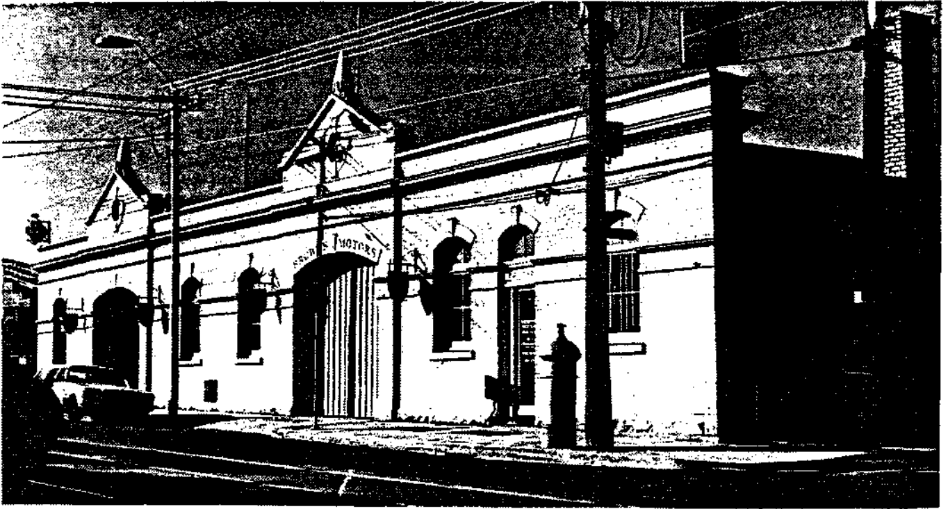
FORMER CABLE TRAM ENGINE HOUSE, 626 HIGH STREET
