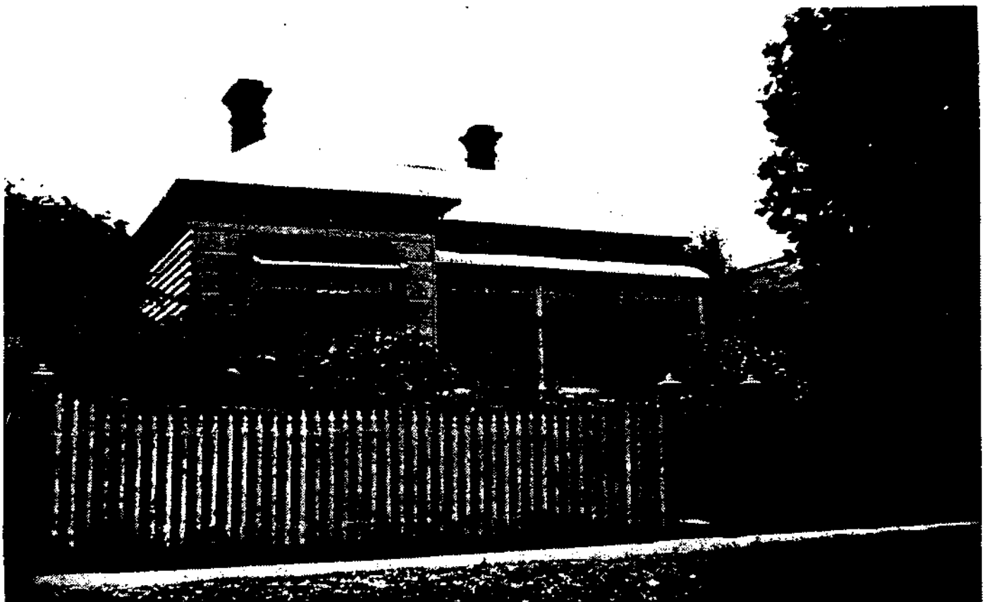
House, 39 Christmas St., c1905, intact fence and planting to front garden also possible remnant of original colour scheme. Refer detail.
