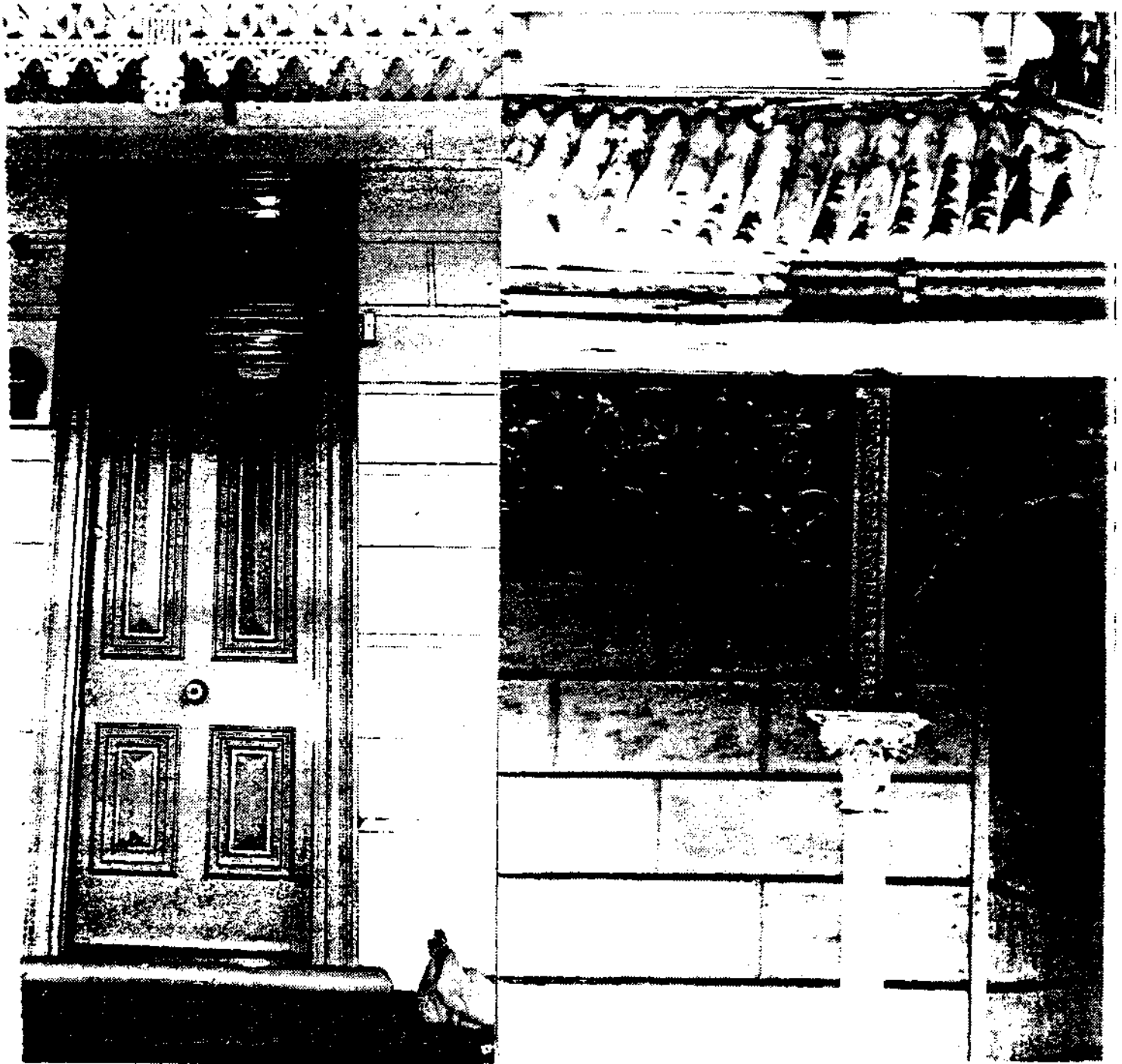
Detail, 175 Gillies Street (1906): note pressed metal ogee-profile gutter and clip, earlier ogee gutter did not have the rolled edge and were fixed with gutter spikes.
