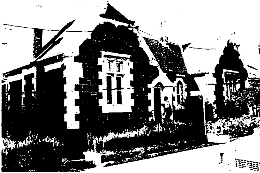
Secretary's Office, formerly Association or Founders Cottage, 12 Coppin Avenue, Constructed 1870, Architect: George Johnson
