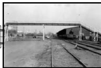
Footbridge within Edinburgh Gardens
