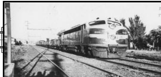
Amess Street Crossing.
