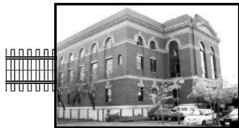
North Fitzroy Electricity Substation built 1912
