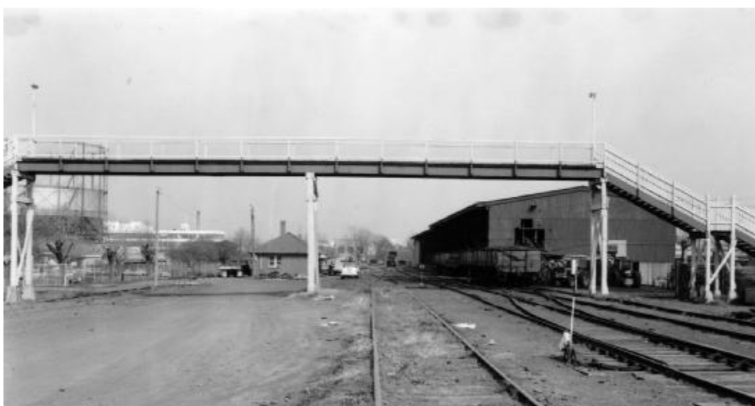
Figure 8 Footbridge across railway line at Fitzroy (Edinburgh Gardens) Source: Victorian Railways Collection, Public Record Office, c.1970s.
