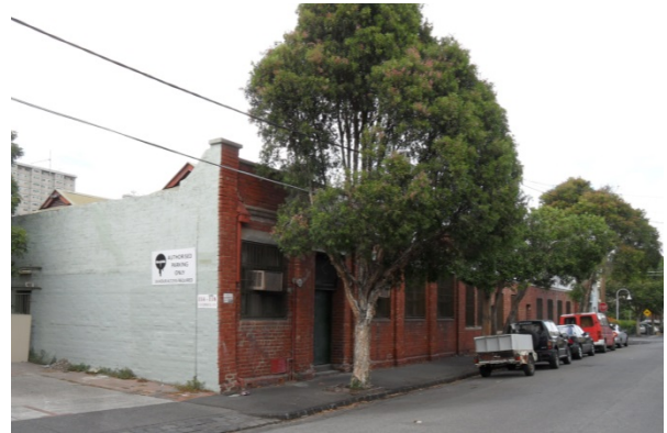
Factory at 114 Campbell Street, 2015.
