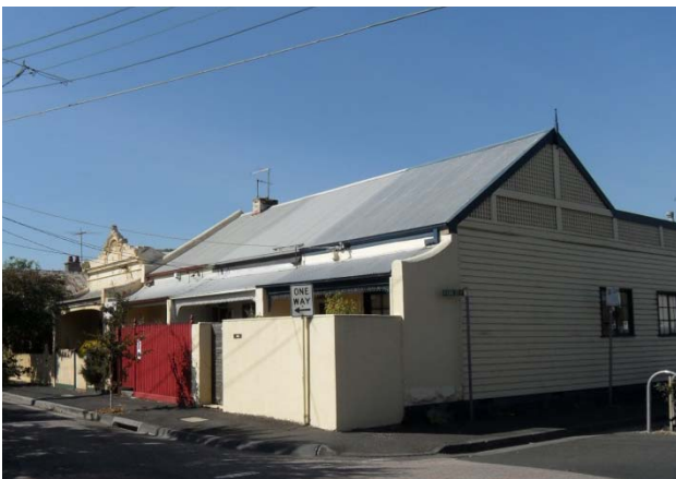
57-63 Stafford Street, looking east, 2015.
