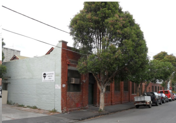
Factory on east side of Campbell Street, looking south.
