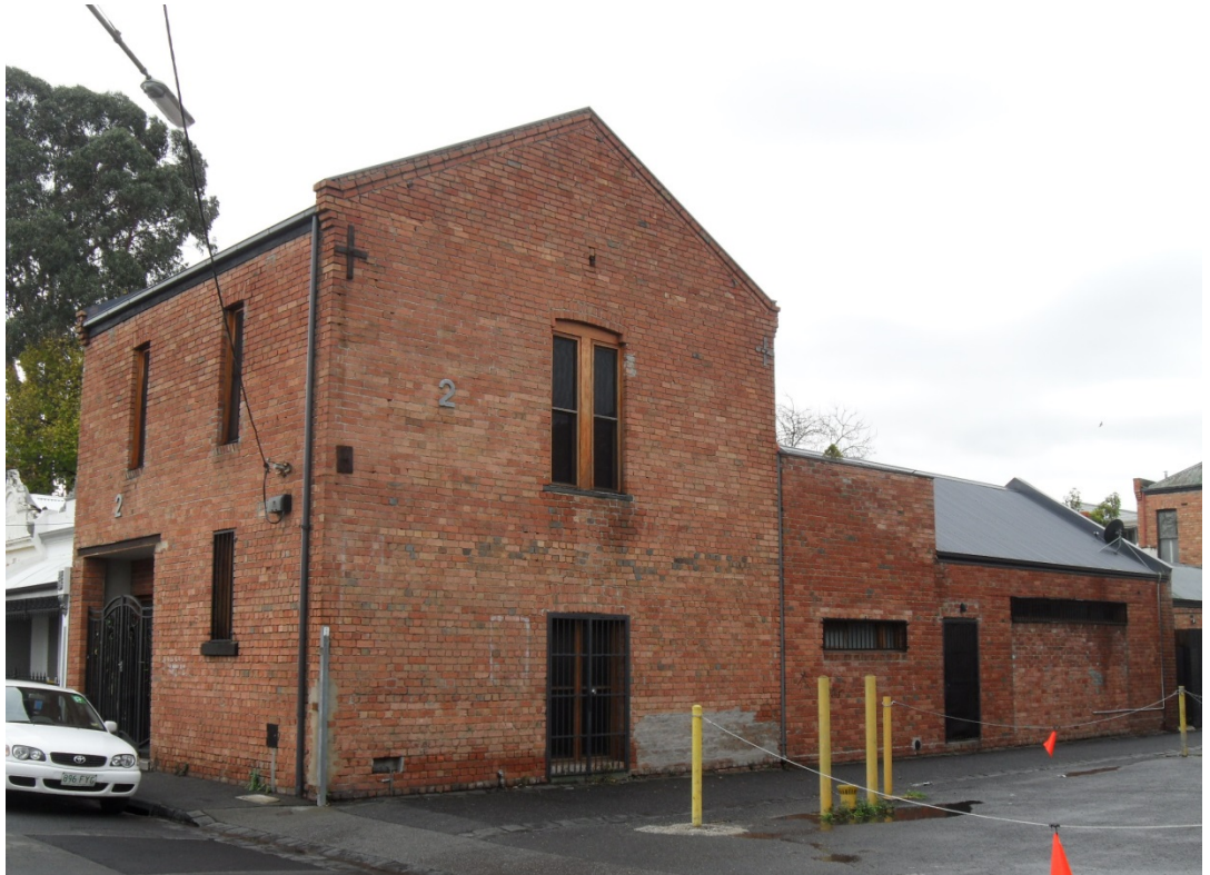
Former stables at 2 James Street, Abbotsford
