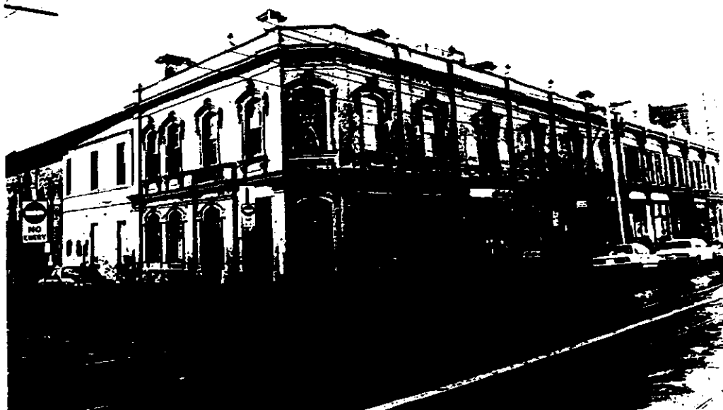
Figure 24 A recent view of the shops adjoining the Gertrude Hotel in Gertrude Street, which were built to take advantage of the consolidation of the street as one of Fitzroy's most important shopping strips.*
