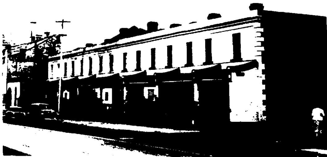
Figure 41 Glass Terrace * at 64-78 Gertrude Street, was constructed in the late 1850s by Hugh Glass. Reproduced from Fitzroy: Melbourne's First Suburb.
