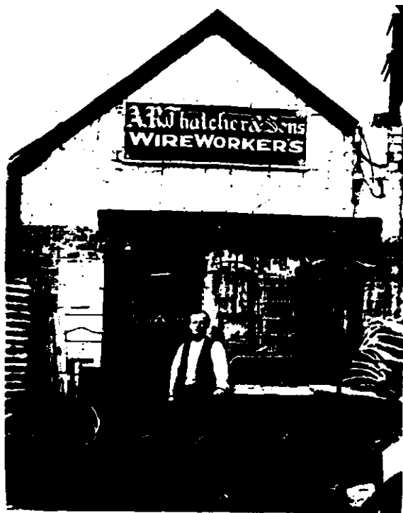
Figure 37 Small works such as A R Thatcher's wireworks in Kerr Street were not looked upon with much favour in the Land Values Research Group study. Thatcher's works are pictured in about 1925. + Reproduced from Fitzroy: Melbourne's First Suburb.
