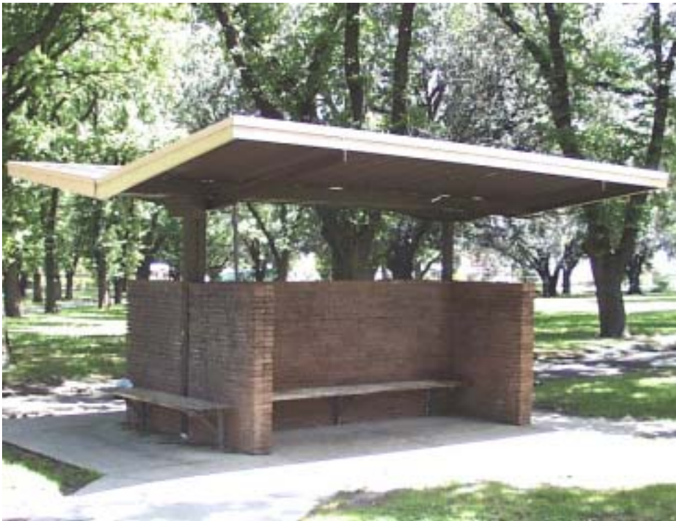
Figure 56 The existing shelter
