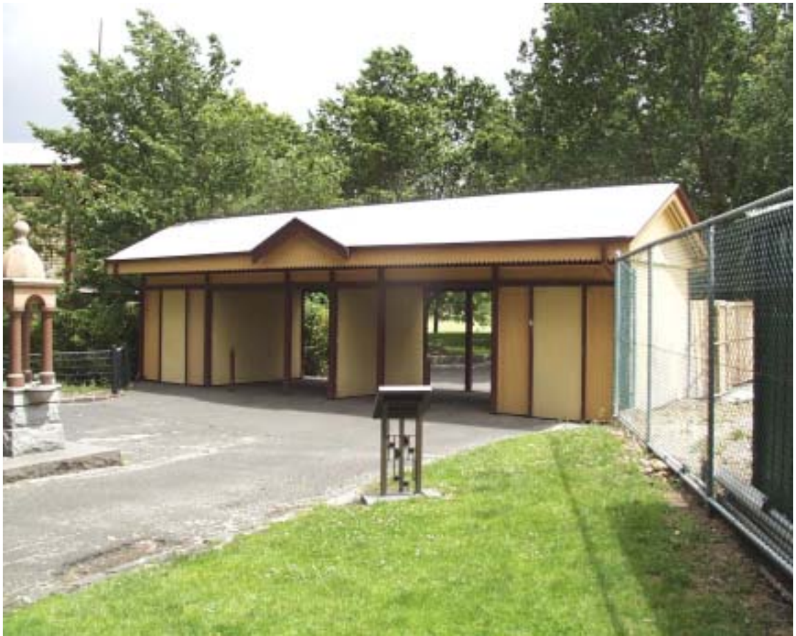
Figure 28 Timber entrance pavilion, viewed from the north-east
