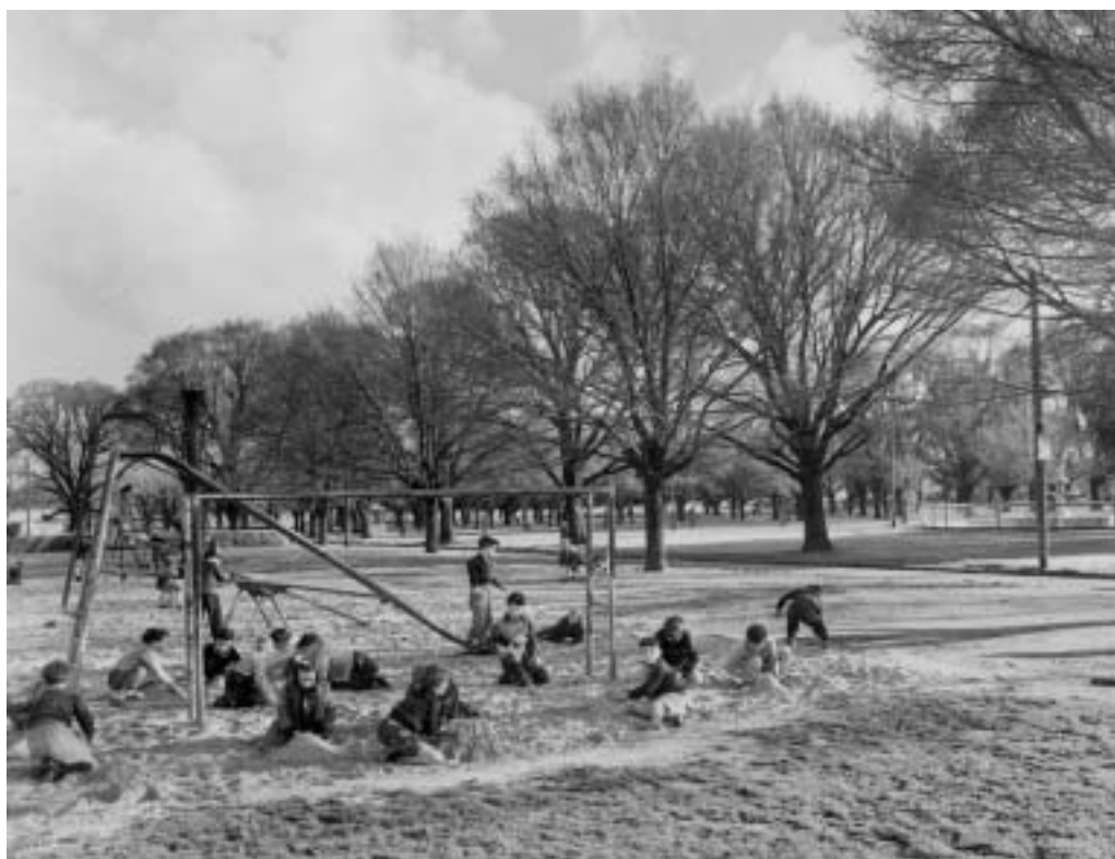
Figure 51 Playground in the Edinburgh Gardens, sited opposite the primary school, 1965. Note the fountain in the background behind the power pole. Source: Fitzroy Local History Collection
