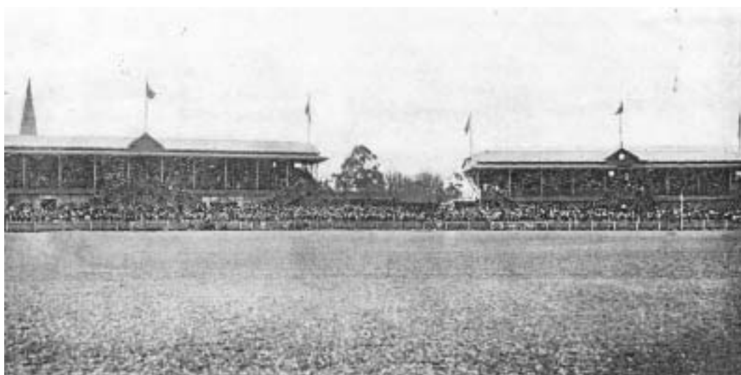
Figure 22 View of the 1905 grandstand (left) and the existing 1888 grandstand (right), c.1913
