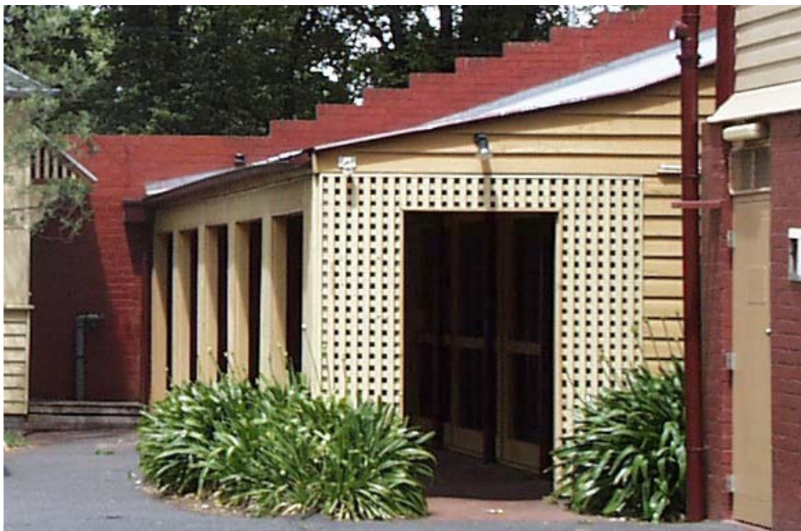
Figure 29 Community Hall (right)
