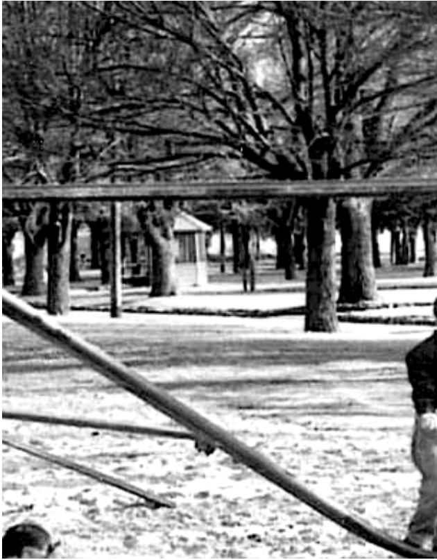
Figure 55 Detail of a 1965 photograph of the Gardens showing the original timber gazebo. Source: Fitzroy Local History Collection
