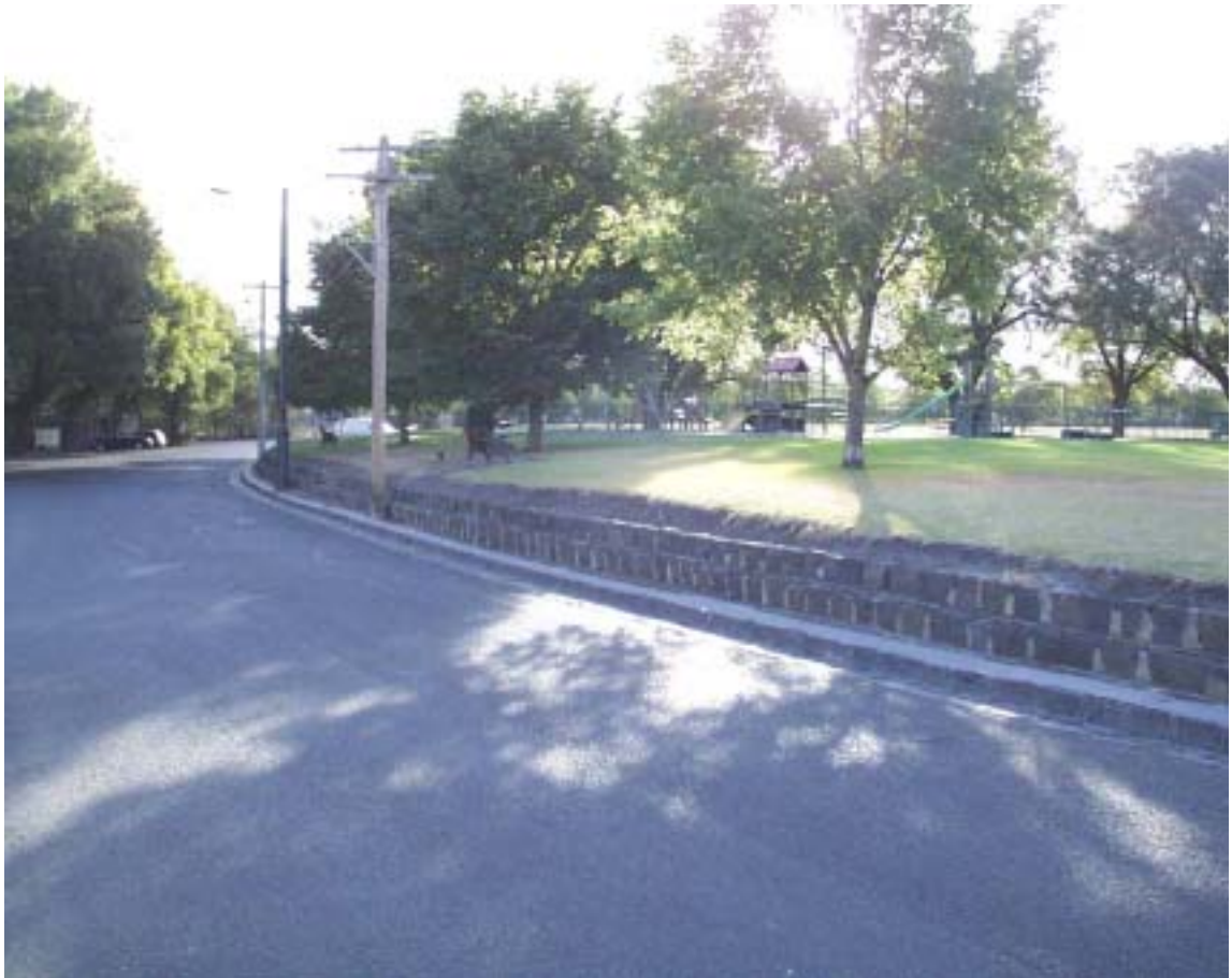
Figure 61 Bluestone retaining wall along Alfred Crescent
