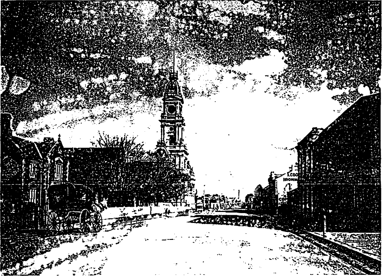
Fig. 3.26 Hoddle Street, outside the town hall, built in 1887, and showing the St. Phillip's vicarage and church (demolished).
