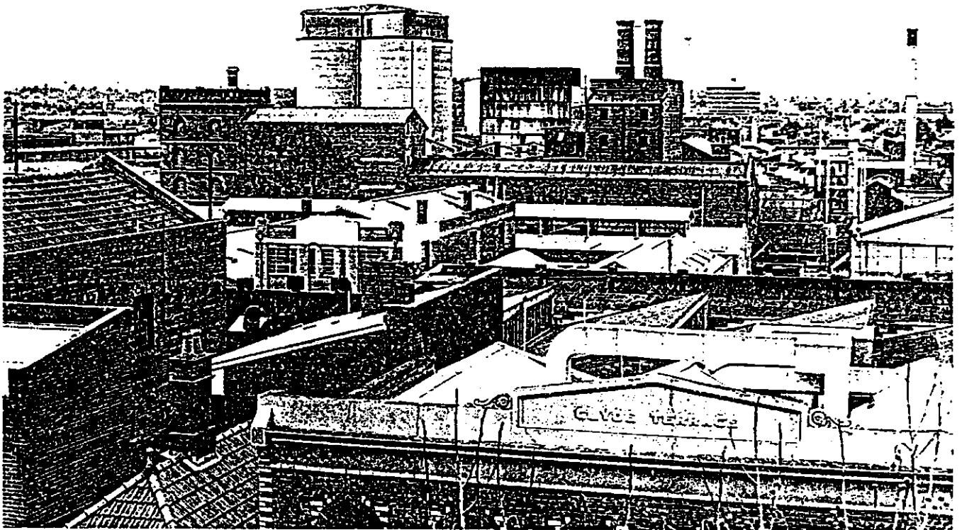
Fig. 3.10 Roof tops of the Collingwood Slope, 1987, looking east from Cambridge Street to Thomas Aitken's Northumberland Street distillery, built in 1862.
