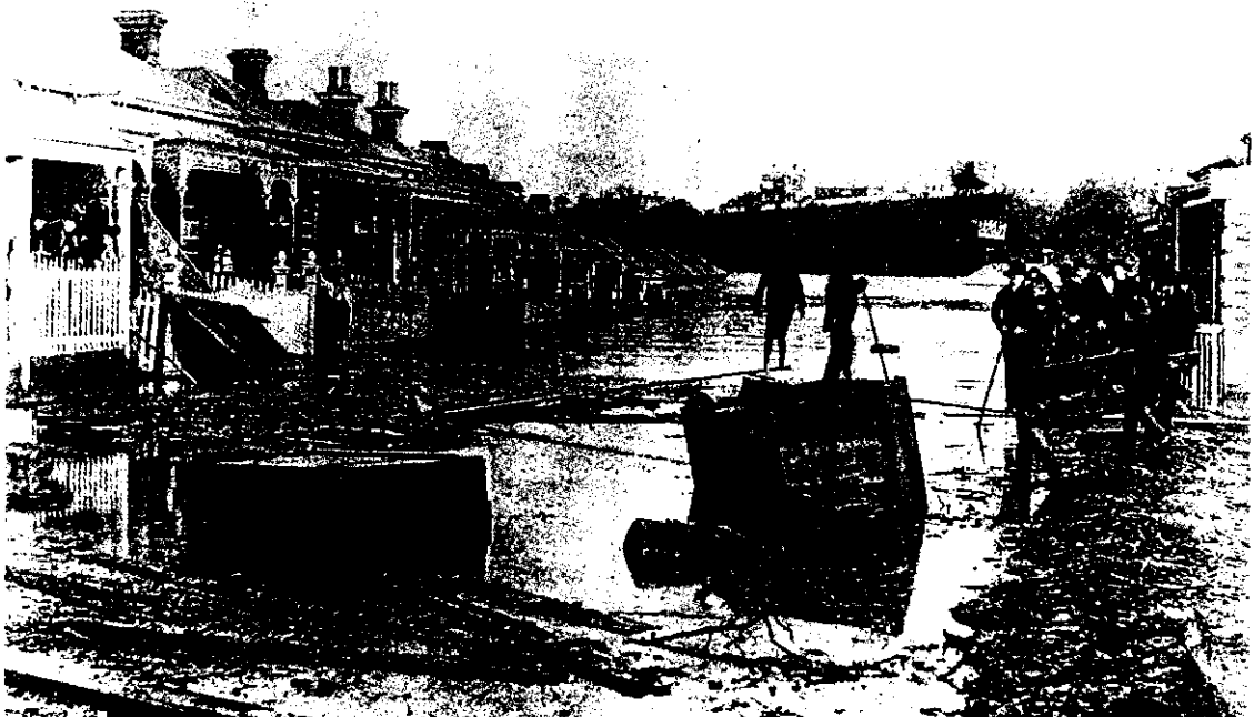
Figure 54 Flooding in Richmond, 1891. Source: Victoria Illustrated, 1834-1984
