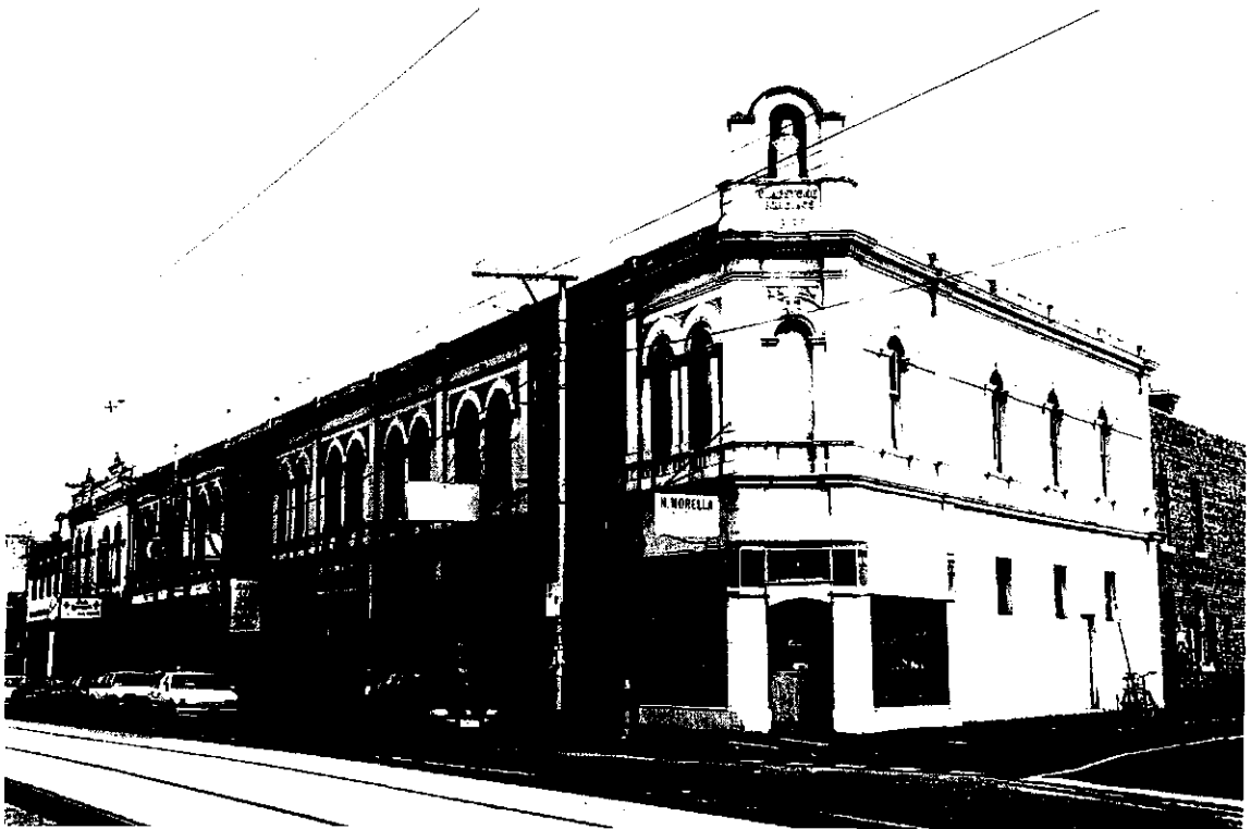
Figure 61 Gladstone Buildings, 169-187 St Georges Road, North Fitzroy
