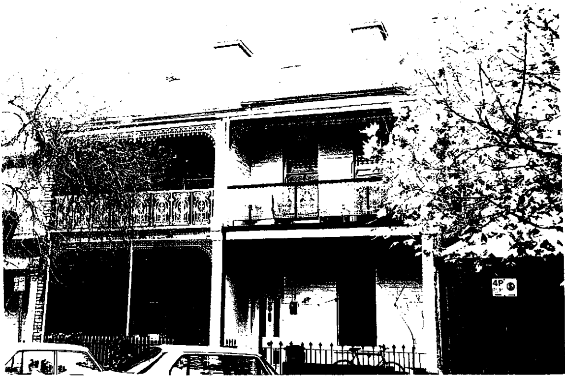
Figure 81 Typical double-storey terraces, 65-67 Westgarth Street, Fitzroy
