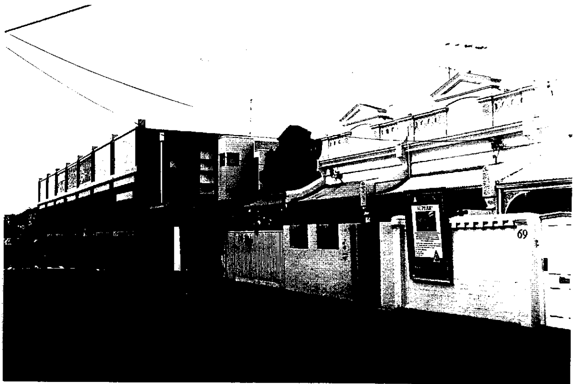
Figure 33 East side Mary Street, Richmond: workers' cottages and converted warehouse
