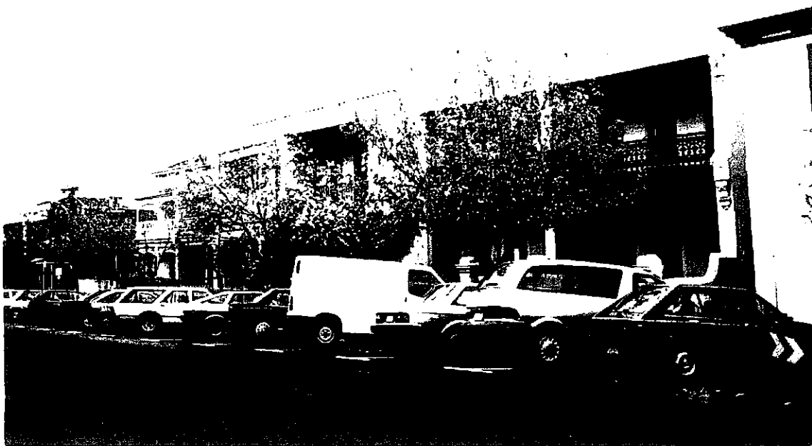
Figure 95 North side Erin Street, Richmond, looking west: note Taragona (1883)
