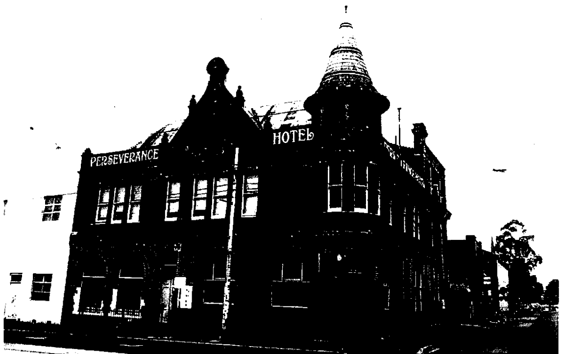
Figure 12 Perseverance Hotel, 196 Brunswick Street, Fitzroy
