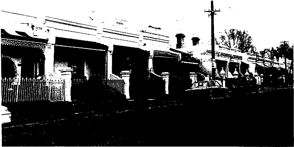
Figure 53 Ornate terraces, West side Station Street, North Carlton
