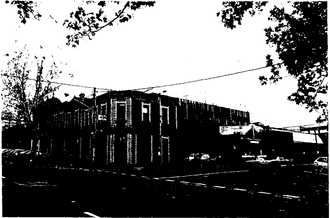
Figure 29 Barnard's Buildings, 28-32 Peel Street, Collingwood, with Foy & Gibson's landmark Wool Sorting and Scouring building in the background.
