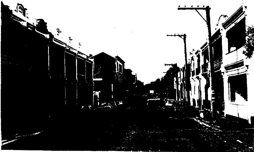
Figure 83 Streetscape, King William Street, looking east
