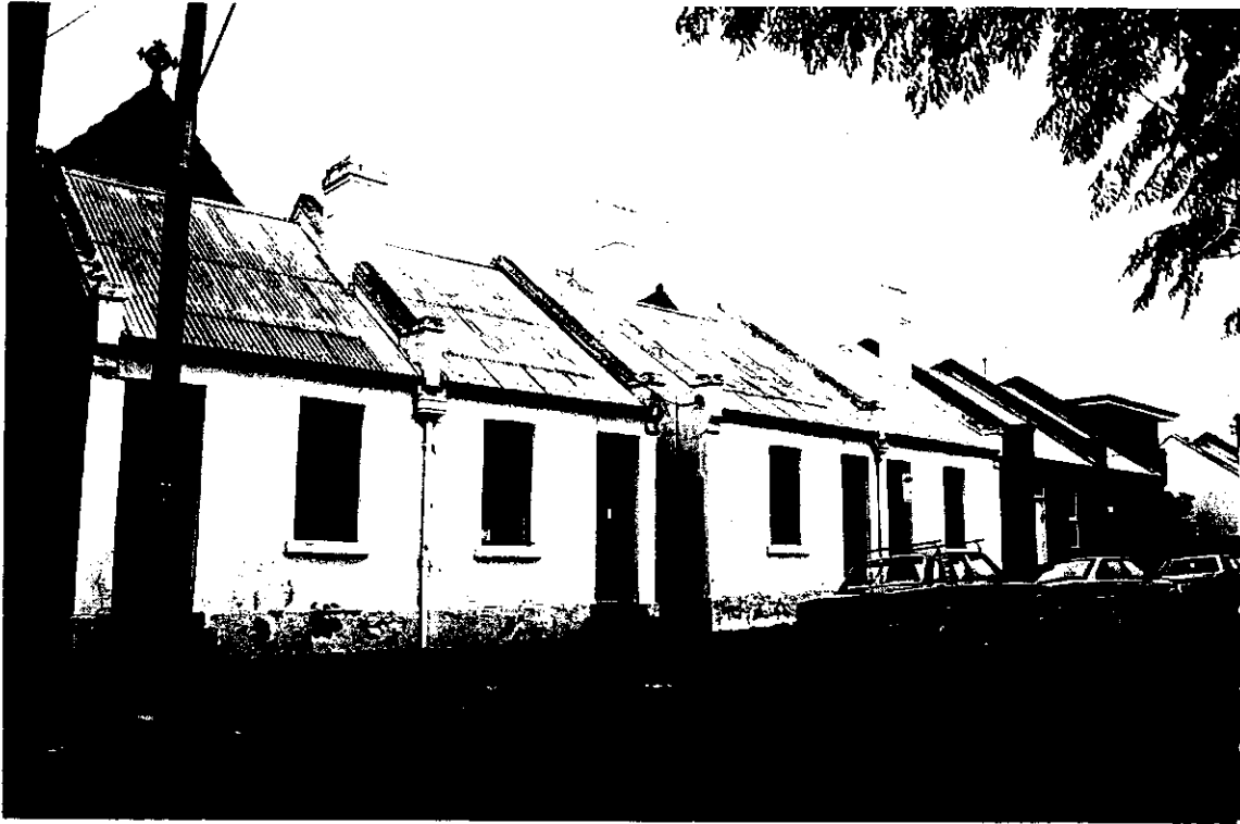
Figure 82 Semi-detached brick cottages, 183-191 Moor Street, Fitzroy
