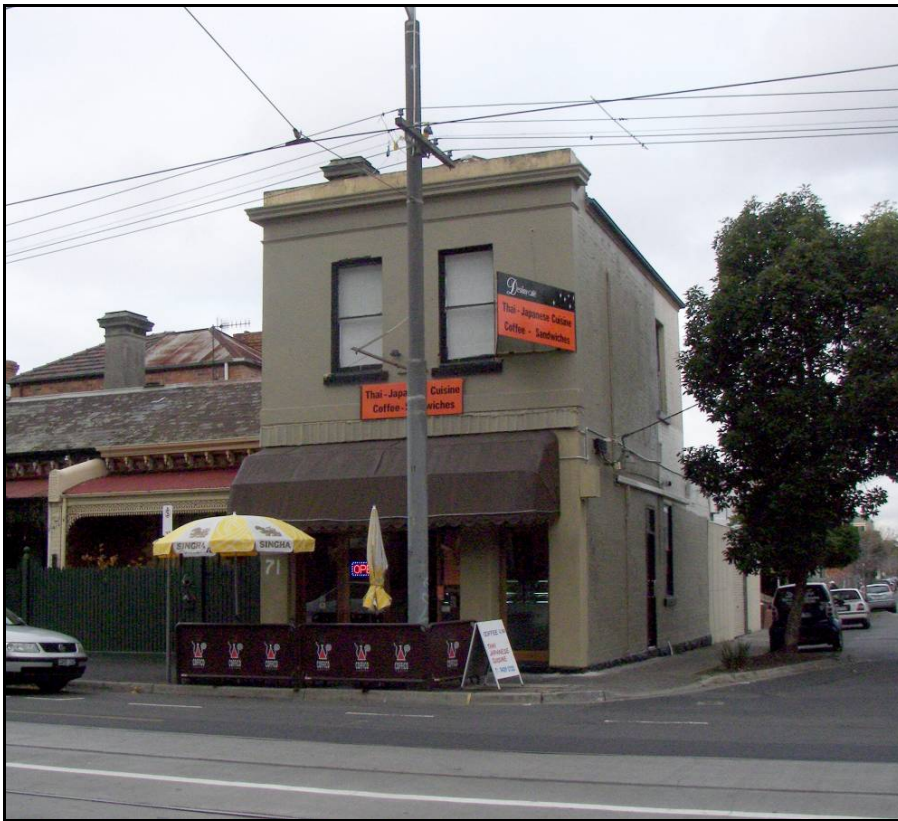
Figure 32 Shop & residence part of row
