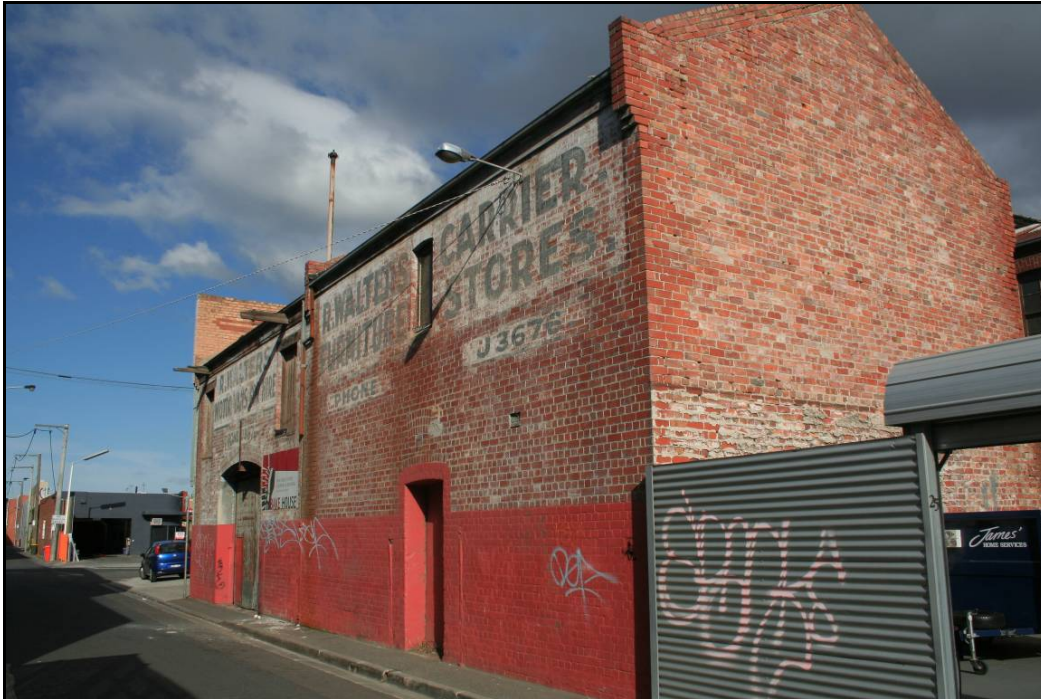
Figure 40 Rear lane stable and store
