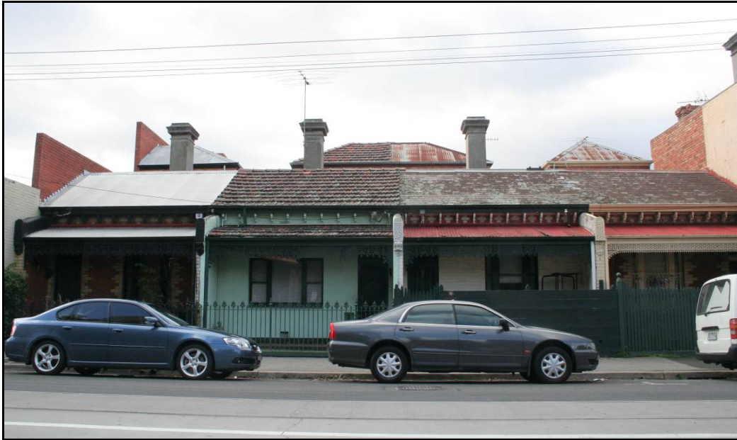
Figure 33 Row house part of row
