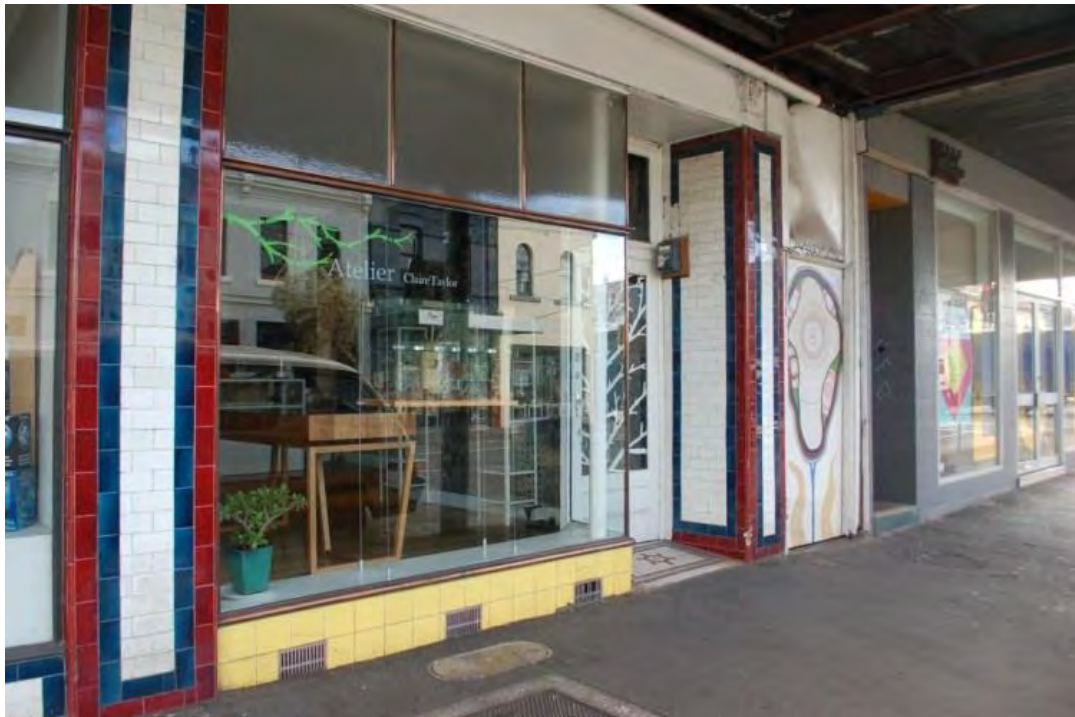
The shopfront of No. 73 Smith Street. Proposed grading: Individually significant.
