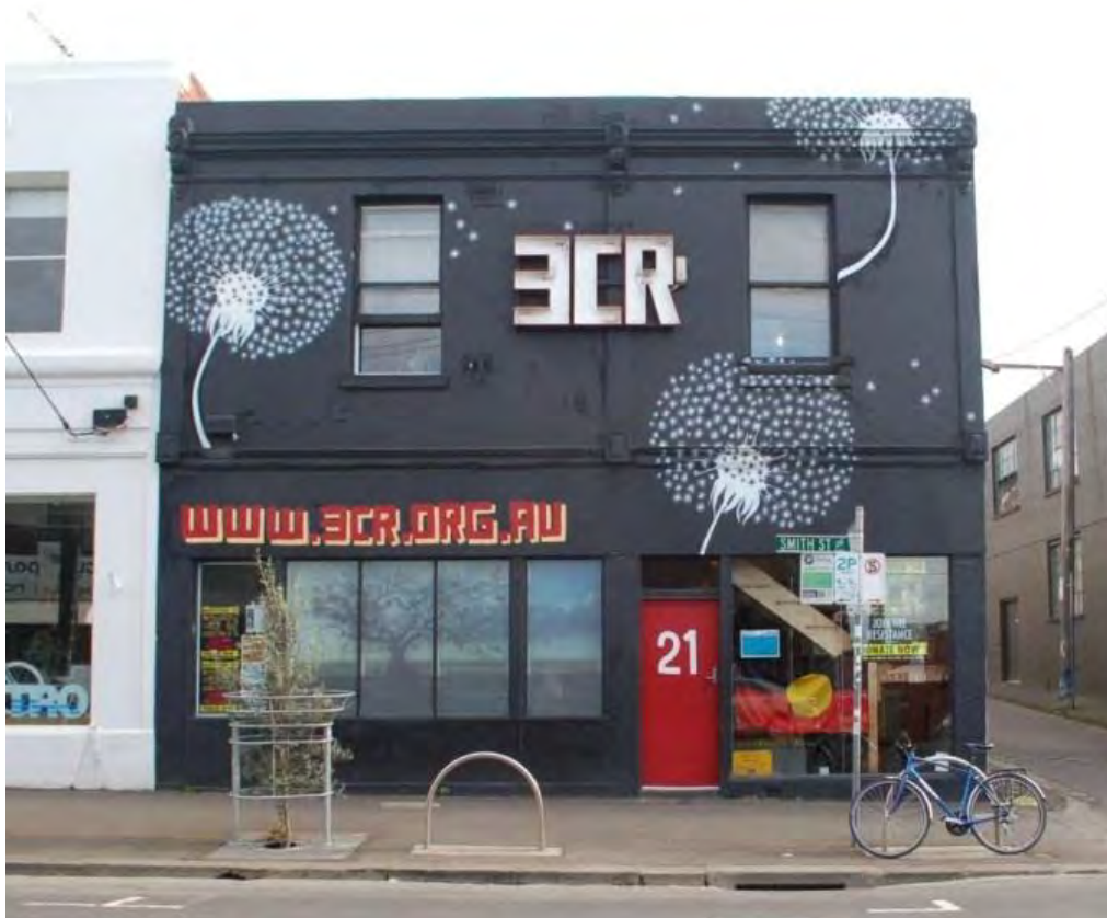
No. 21 Smith Street, Fitzroy (incorporating No. 19). Proposed grading: Contributory.
