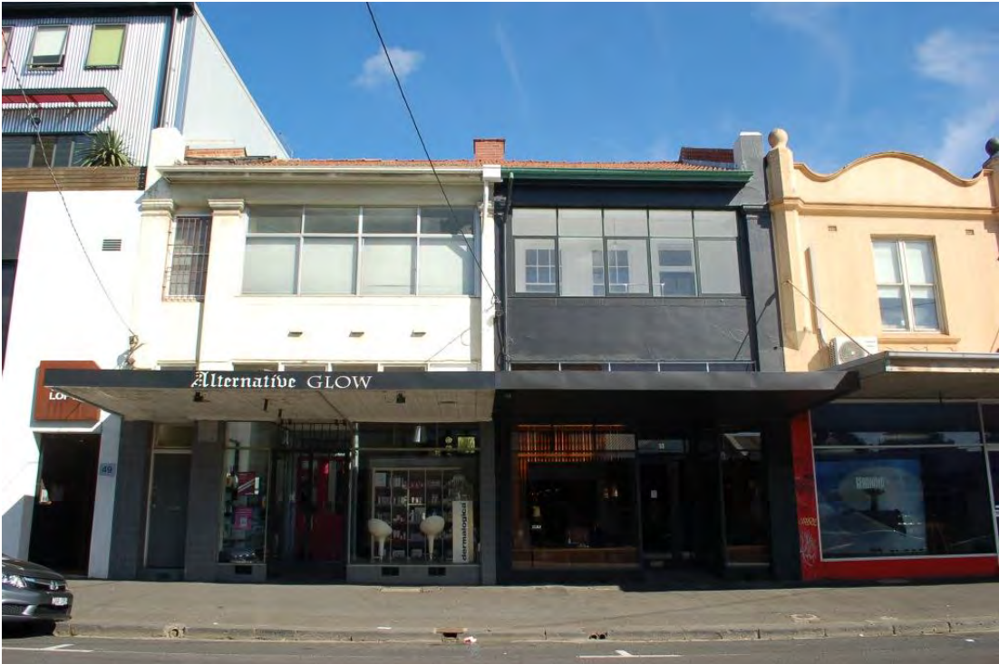
Nos. 51 - 53 Smith Street, Fitzroy (left to right). Proposed grading: Individually significant.
