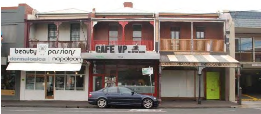
No. 6 Smith Street, Collingwood (right), forms part of a group of three identical shop houses. Proposed grading: Contributory.
