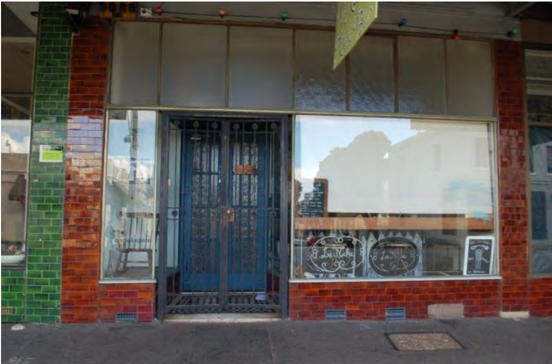
The shopfront of No. 67 Smith Street. Proposed grading: Individually significant.
