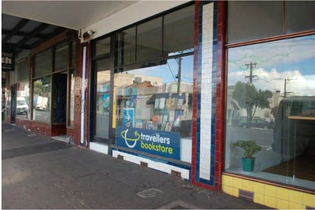
The shopfronts of Nos. 69 (brown tiles) and 71 Smith Street (white tiles). Proposed gradings: Individually significant.
