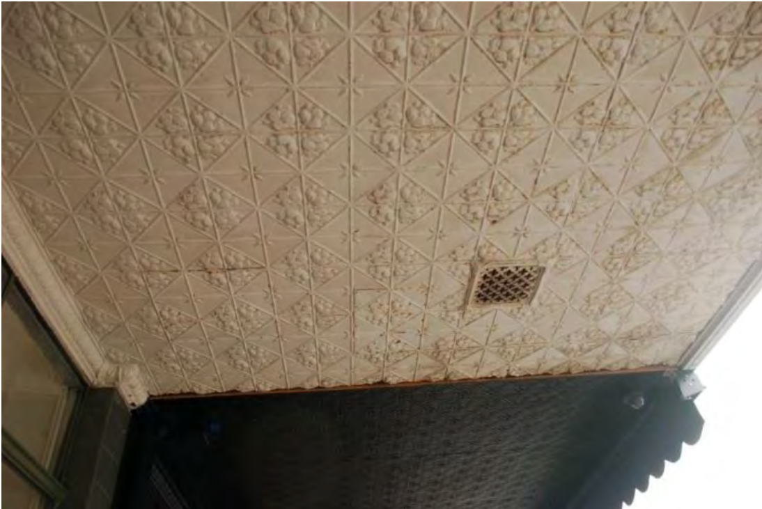
Nos. 51 - 53 Smith Street, Fitzroy. Pressed metal soffit to shop canopies. Proposed grading: Individually significant.
