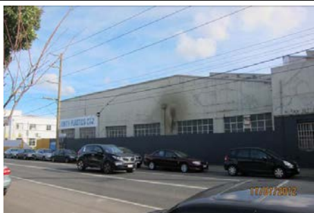
Figure 3. View from Burnley Street of number 198— factory of concrete construction built c.1950 (not included in heritage overlay)
