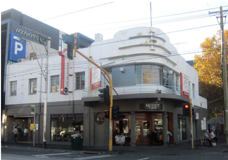
323- 325 Victoria Street, Abbotsford; view of the south-east corner of the building.
