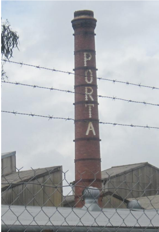
Detail of chimney stack.
