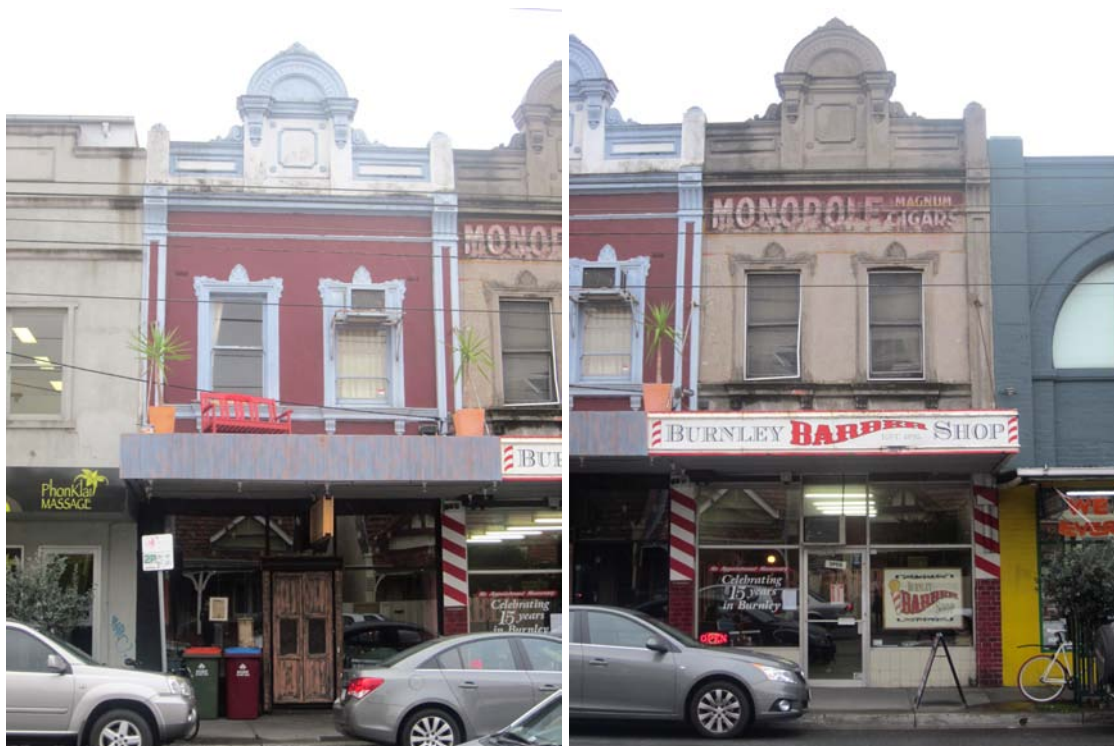
No. 413 Swan Street at left, and no. 415 Swan Street at right.
