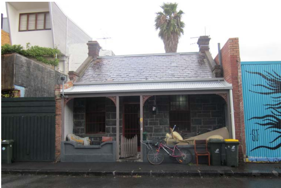
Front (north) facade of 4 Henry Street showing the irregular stone patterning.
