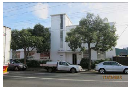
Figure 4. The south-east portion of 198 Burnley Street (formerly 240 Burnley Street) – former offices for Australian General Electric Company built between 1945-1948 (not included in heritage overlay)
