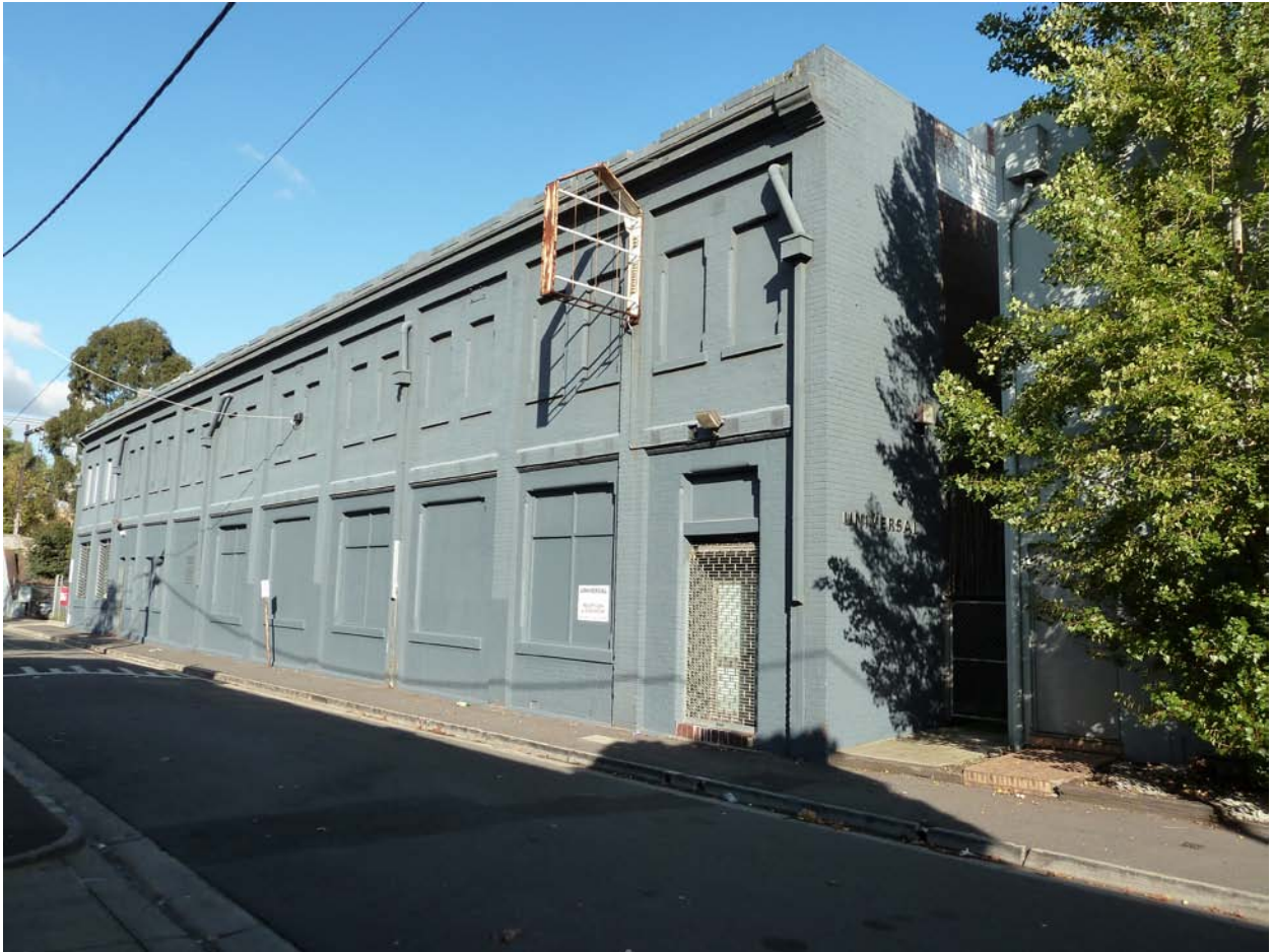
View of the south façade, looking east down Stafford Street.
