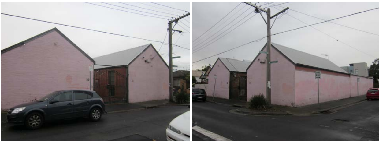
Left to right: View of the south elevation looking north east across Farmer Street; view of the east elevation looking north along Cutter Street.
