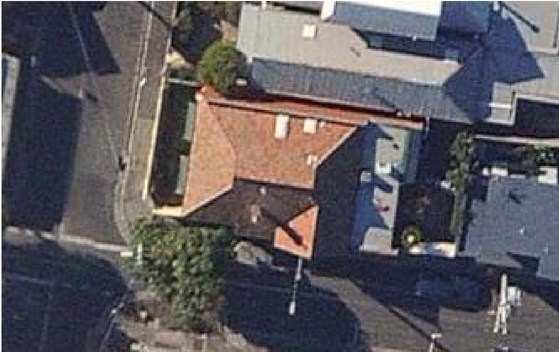
Recent aerial image, showing 89 Neptune Street.
