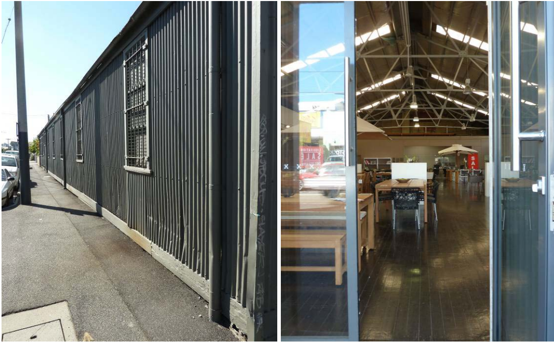
From left: West elevation to Duke Street; interior view of the Drill Hall showing the timber flooring.
