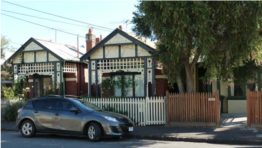
No. 164, 162 and 160 Lord Street showing the overpainted brick facade to No. 160.
