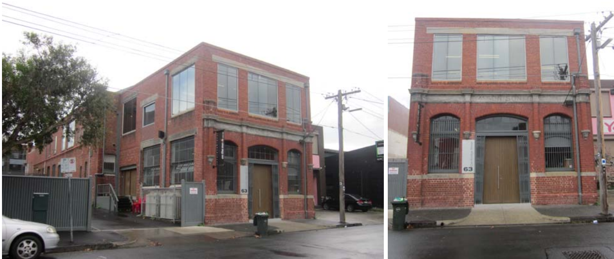
Left to right: Views of 63 Cambridge Street, Collingwood, showing the altered east façade.
