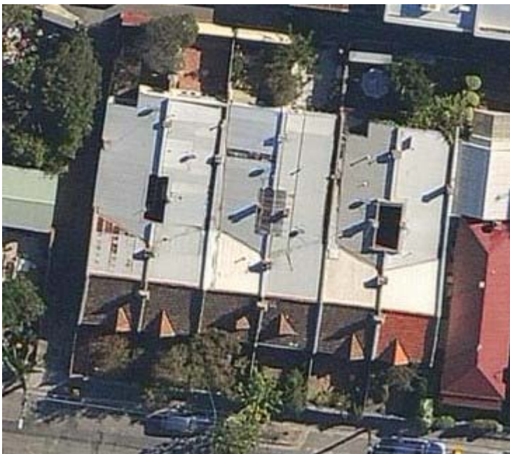
Recent aerial photograph of the properties, showing the floating gables to the central pair of dwellings, and gablets to the outer pair.
