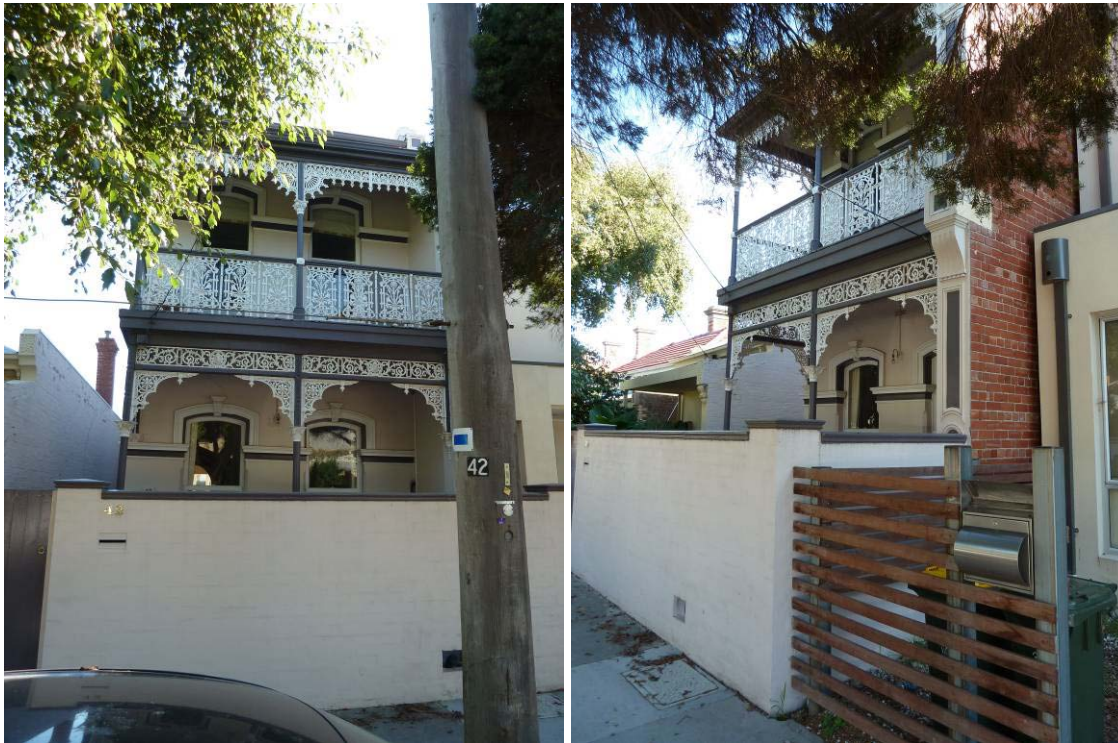
Left: 42 Edinburgh Street front façade. Right: View of the façade looking south-west showing the exposed brick work to the north elevation.
