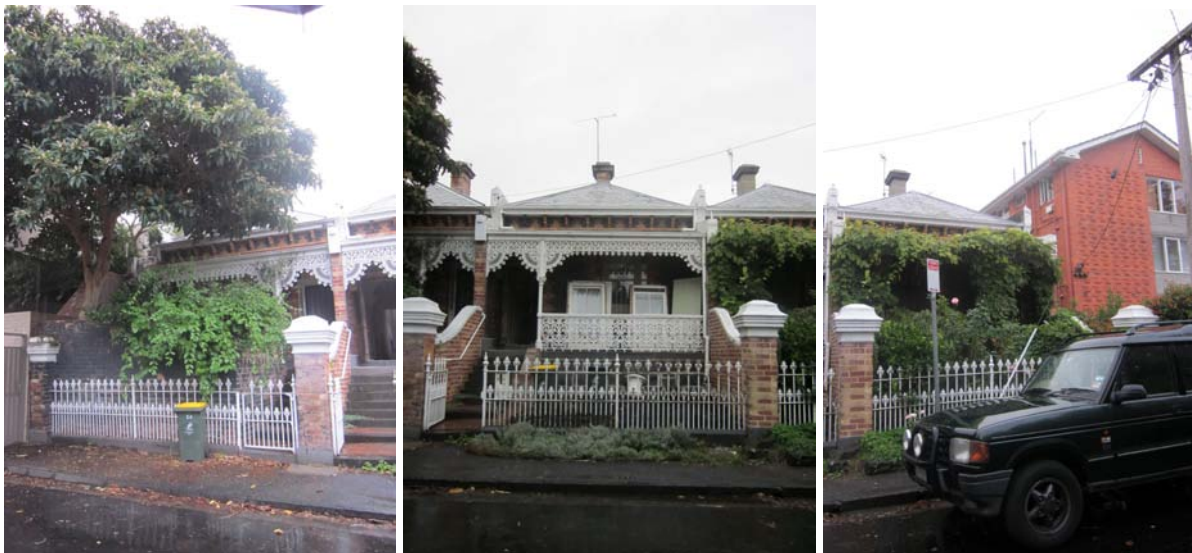
From left: 26 Park Avenue, 24 Park Avenue, 22 Park Avenue.
