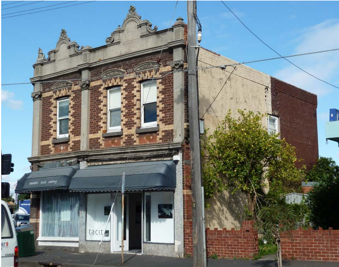
View of north façade and west wall of nos 323- 325 Johnston Street.
