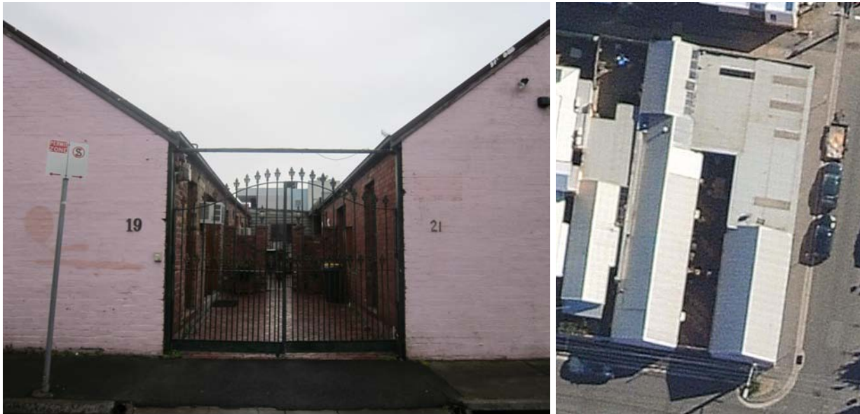
Left to right: No.19-21 Farmer Street front (south) elevation showing the gated front entry; recent aerial photograph of the site showing the separate gable roof forms facing Farmer Street (bottom of image).
