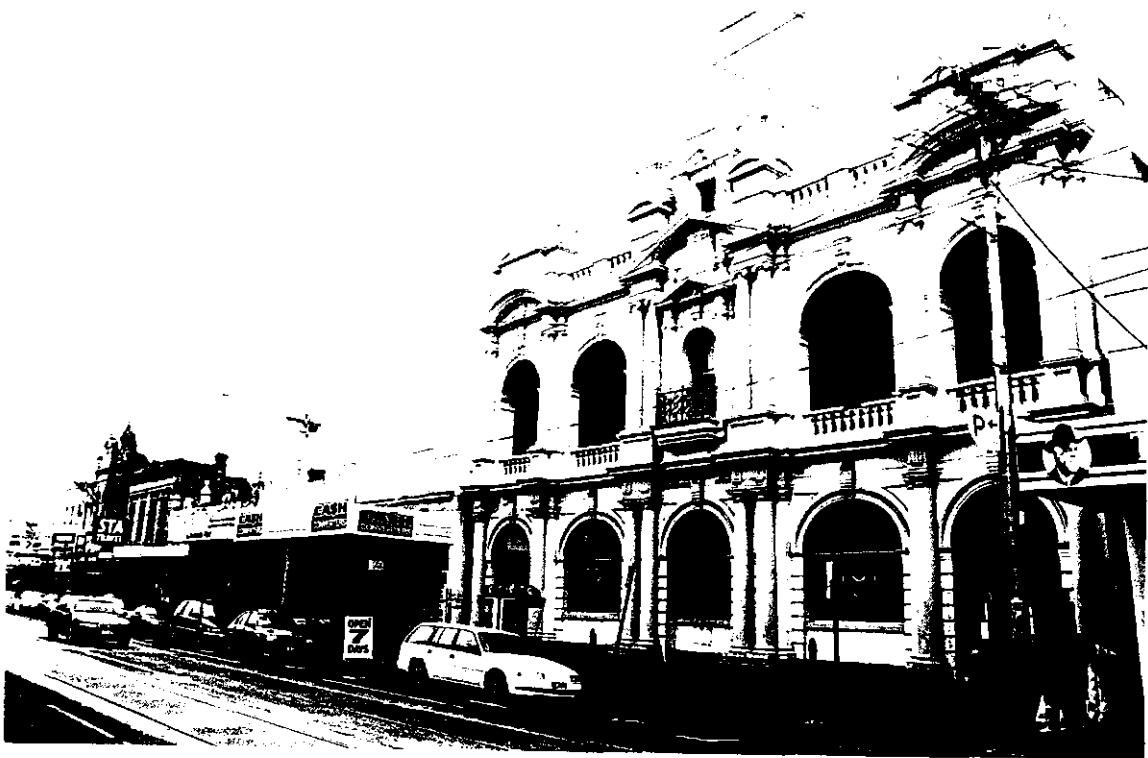
Figure 78 East side Smith Street, Collingwood, with the former Collingwood Post Office in the foreground
