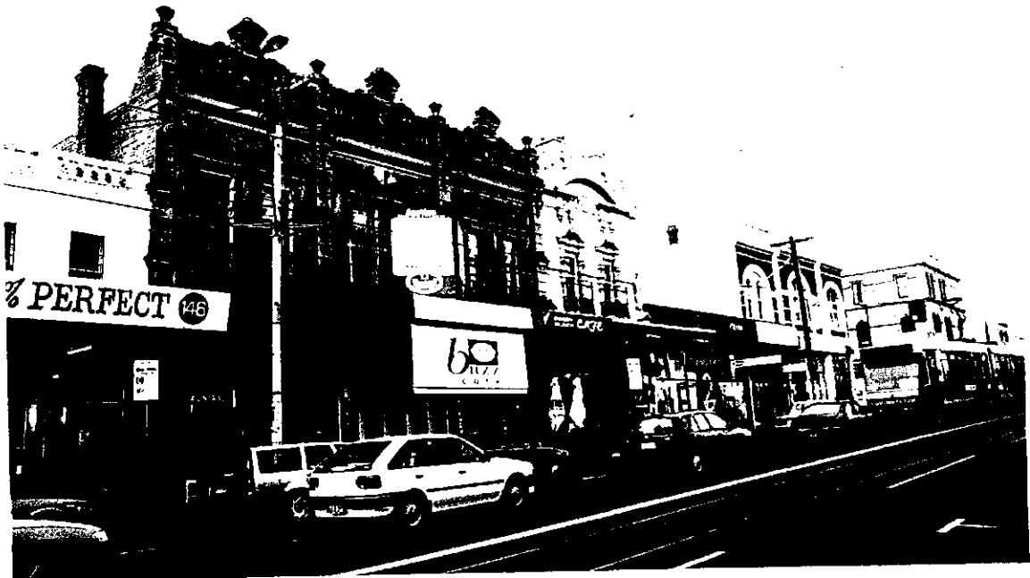
Figure 8 South side Bridge Road, Richmond, looking west
