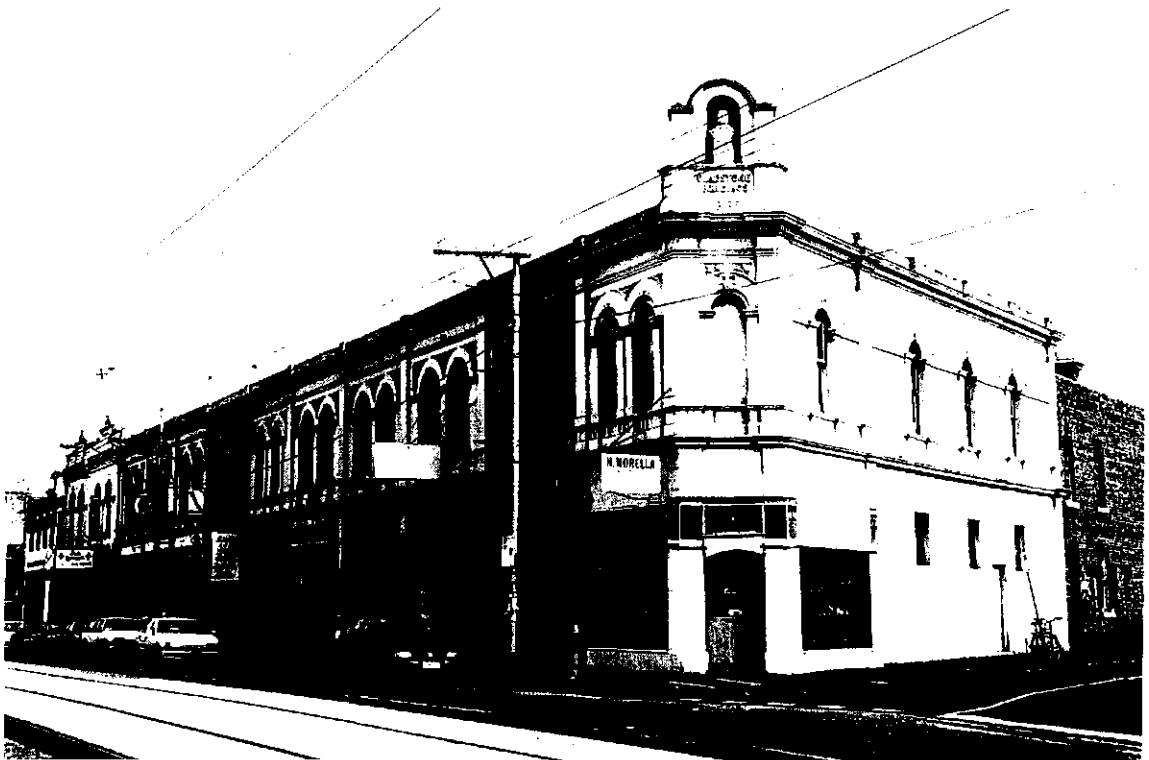
Figure 61 Gladstone Buildings, 169-187 St Georges Road, North Fitzroy
