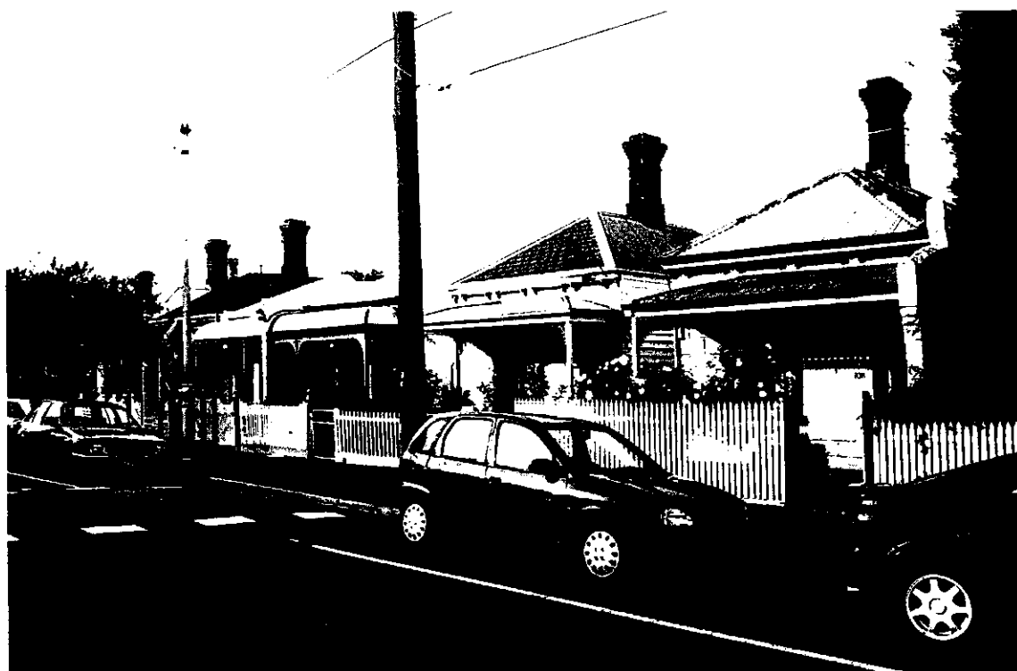
Figure 51 Workers' Cottages, south side Buckingham Street, Richmond
