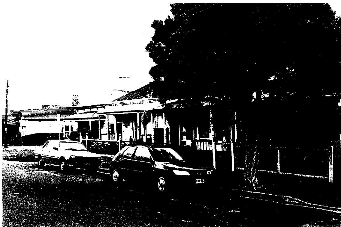
Figure 2 Typical modest timber cottages, 274-280 Mary Street, Richmond
