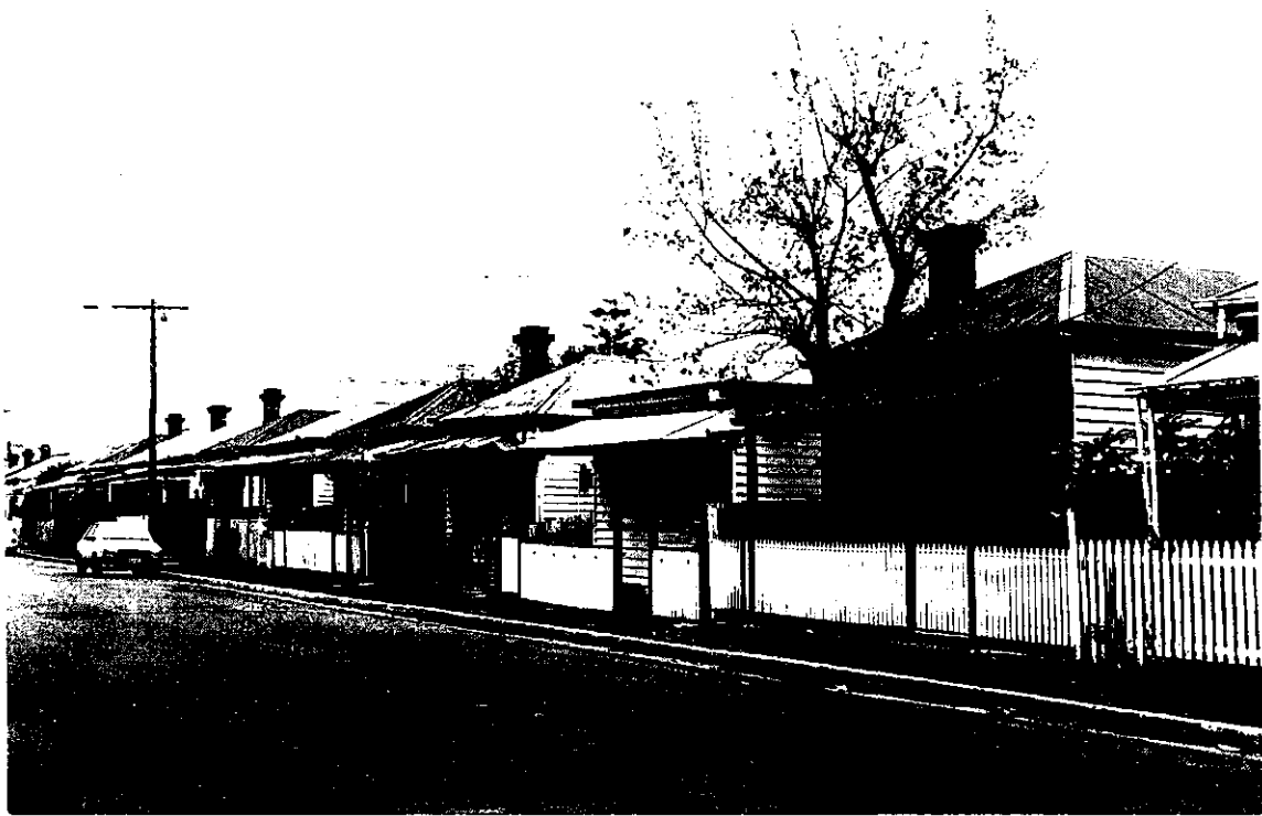
Figure 14 Timber cottages, west side Campbell Street, Collingwood
