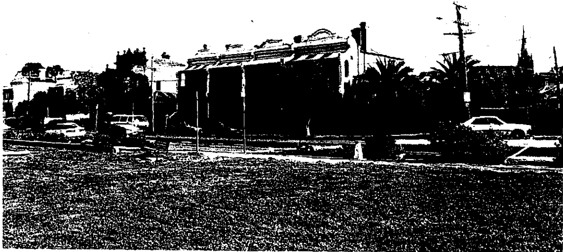
Figure 26 West side Gold Street from the Darling Gardens, Clifton Hill: the spire of St John's is visible in the background
