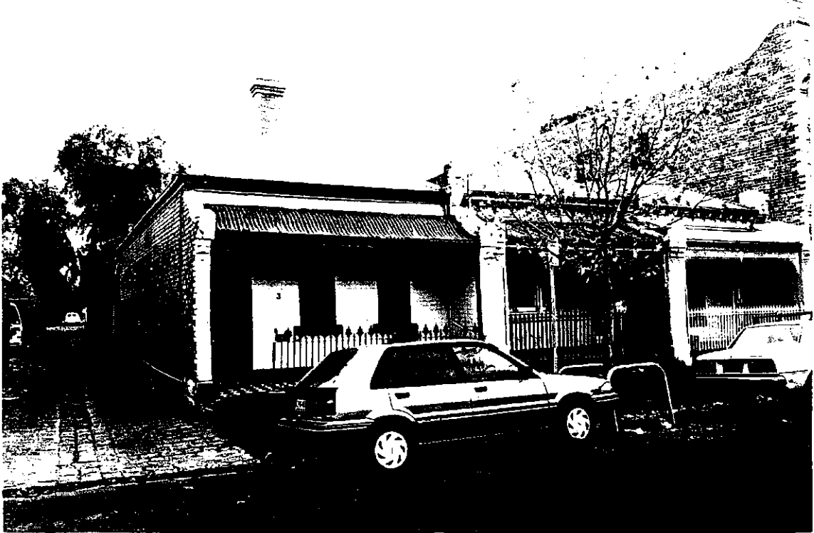
Figure 58 Typical modest Victorian brick terraces, 3-5 Birkenhead Street, North Fitzroy
