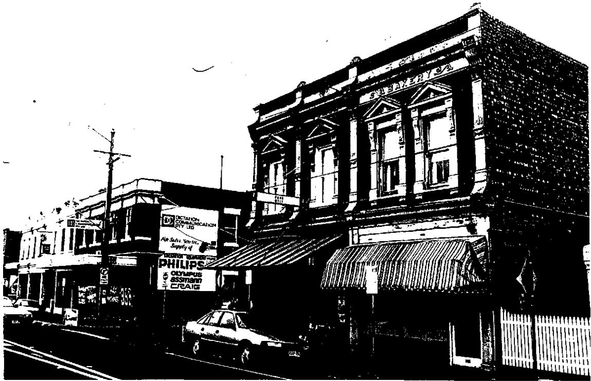
Figure 60 Victorian shops, 98-114 Scotchmer Street, North Fitzroy, with the former Ennis Tymon Bakery in the foreground
