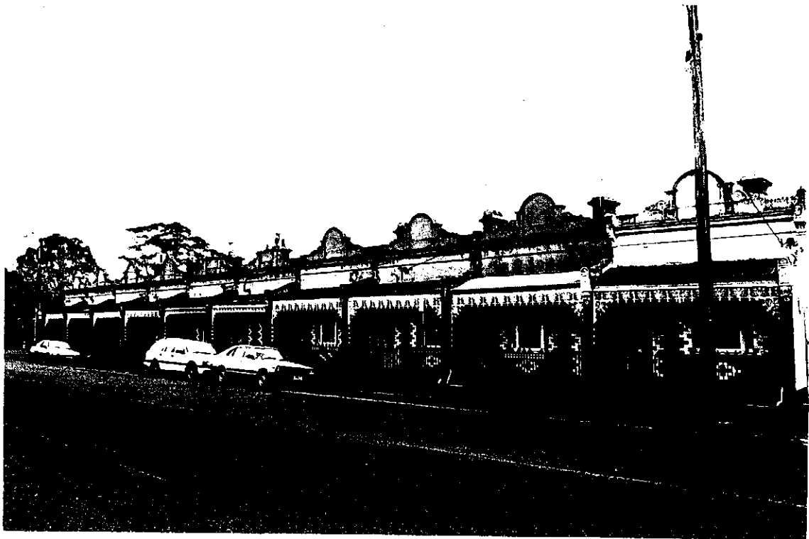
Figure 67 Terraces, 100-118 Paterson Street, North Carlton
