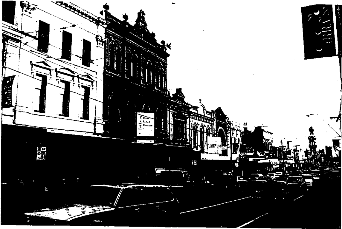
Figure 85 North side Swan Street, looking towards Church Street
