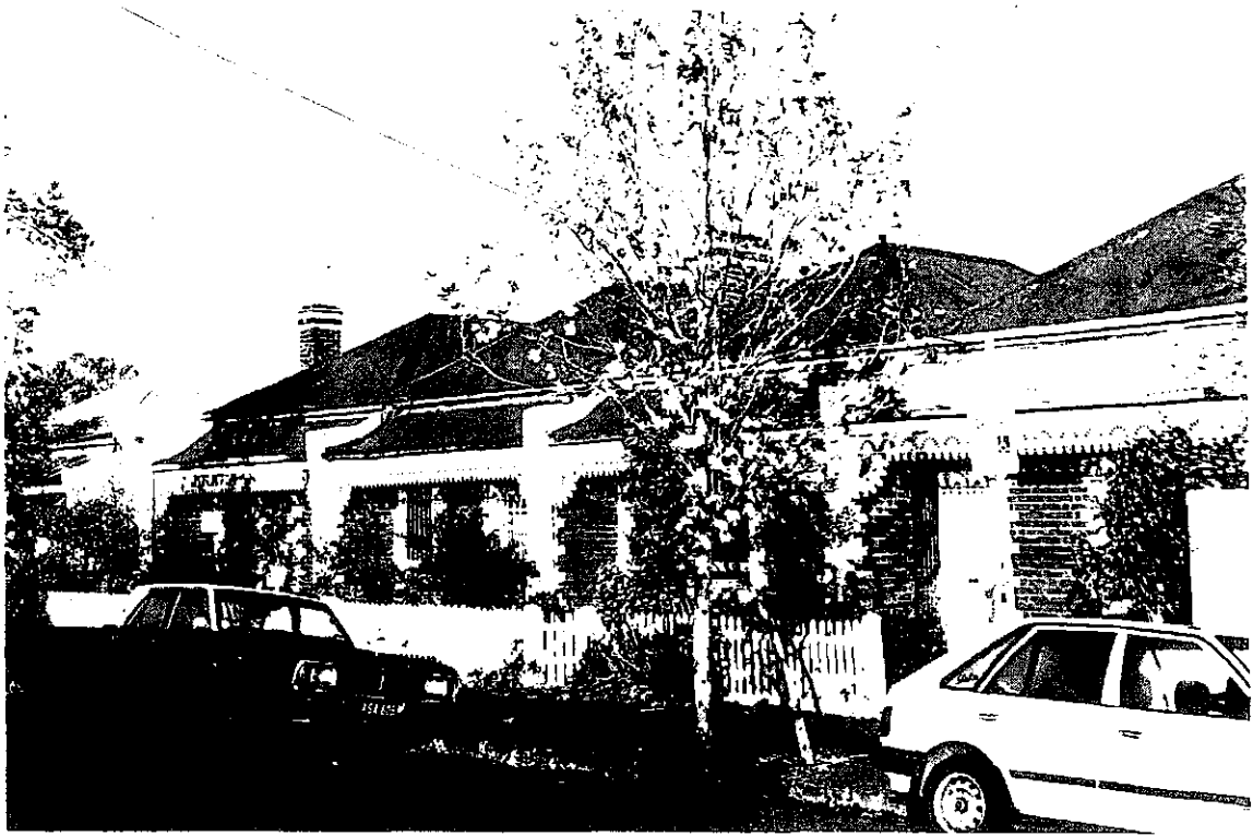
Figure 98 Bichromatic terraces, west side William Street, Abbotsford, looking south
