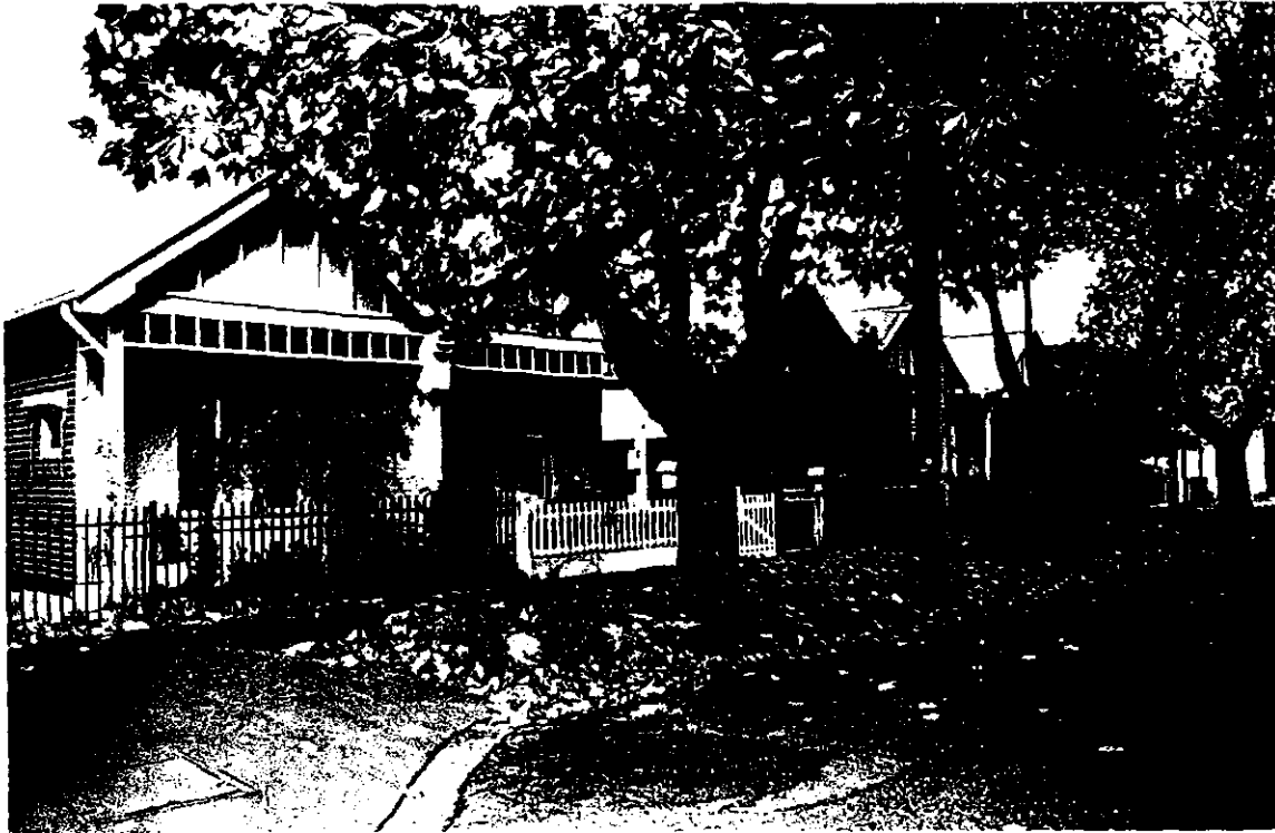
Figure 5 Edwardian cottages, 2-16 Moore Street, Richmond
