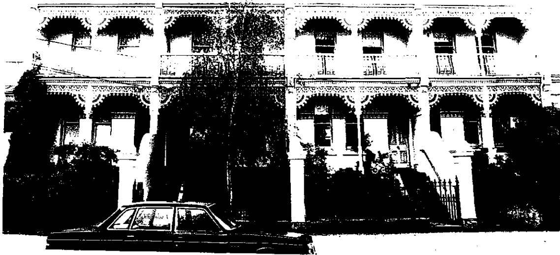
Figure 55 St Edmonds Terrace, 789-795 Drummond Street, North Carlton: note intact front fences and bluestone steps
