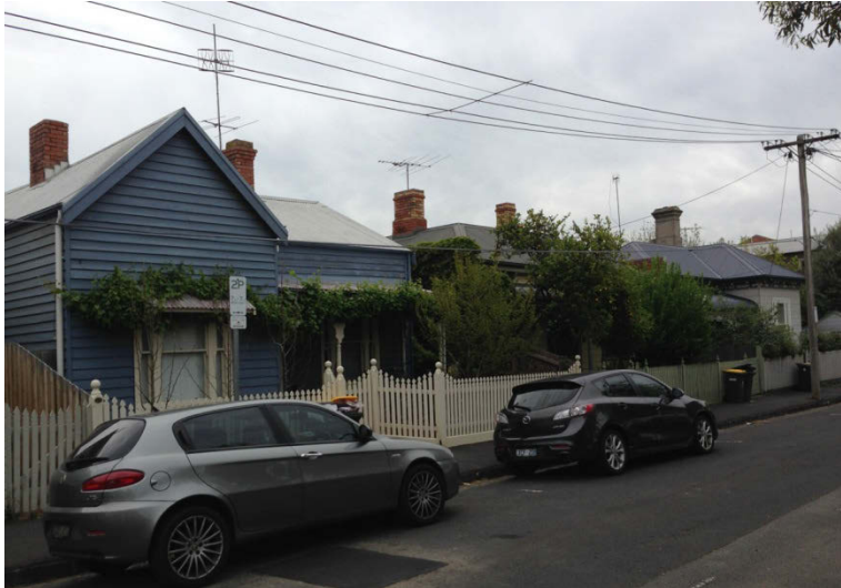
Bellevue Street, south side looking west showing late Victorian timber houses
