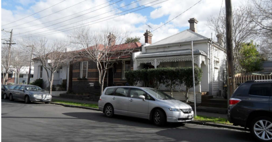
Late Victorian and Federation houses at 32-36 Charles Street (Recommended for inclusion in HO319)
