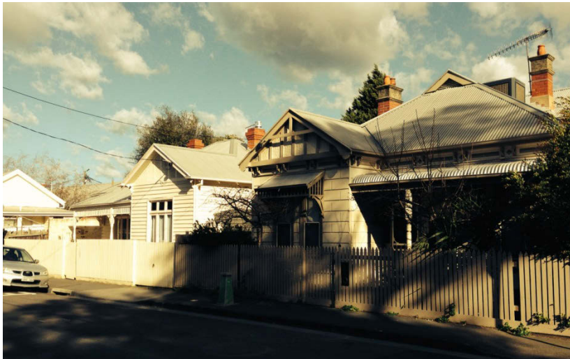
Asymmetrical Edwardian timber houses at nos. 26 & 28 Stawell Street
