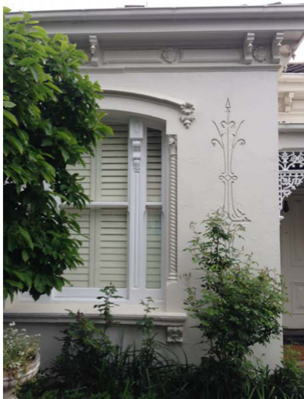
12 Newry Street detail showing incised and moulded decoration to the projecting bay (at right)
