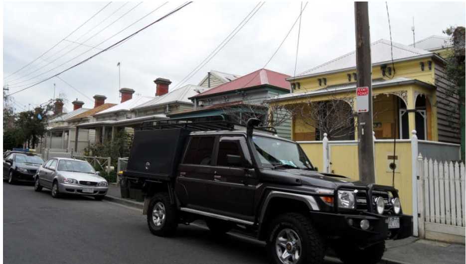
Timber cottages, 22-30 Neptune Street
