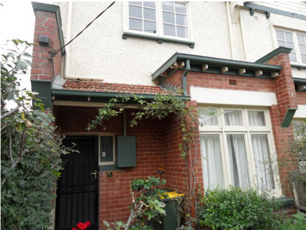
Detail of 5 Brougham Street showing entrance and bay window (below)
