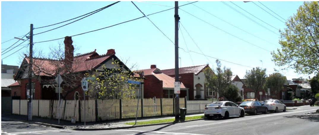
Edwardian and interwar houses, west side between Abinger and Sheedy streets
