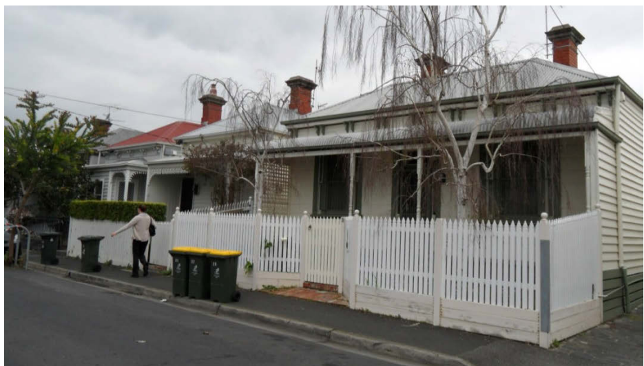
Timber cottages and house, 27-31 Fraser Street
