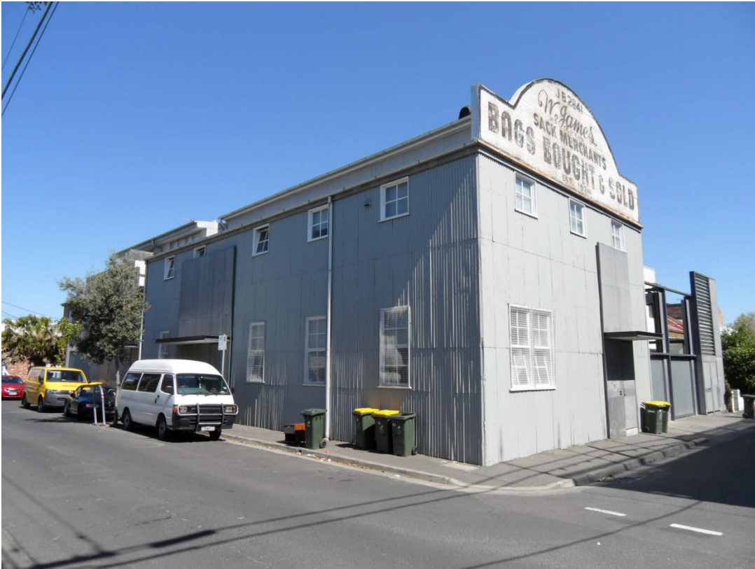
Former W. James & Co. Sack Merchants factory
