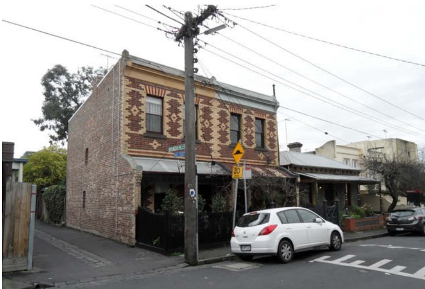
Two storey bi-chrome brick houses at 23 & 25, and house 27 Abinger Street
