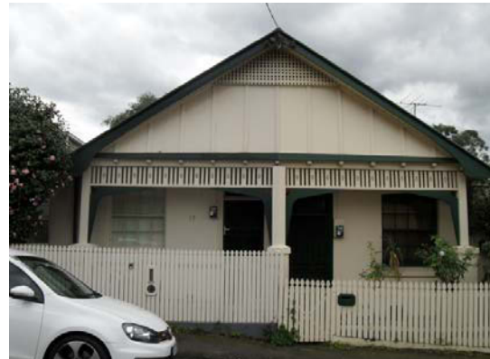
17-19 Brougham Street: At left is currently outside HO319; at right is within HO319
