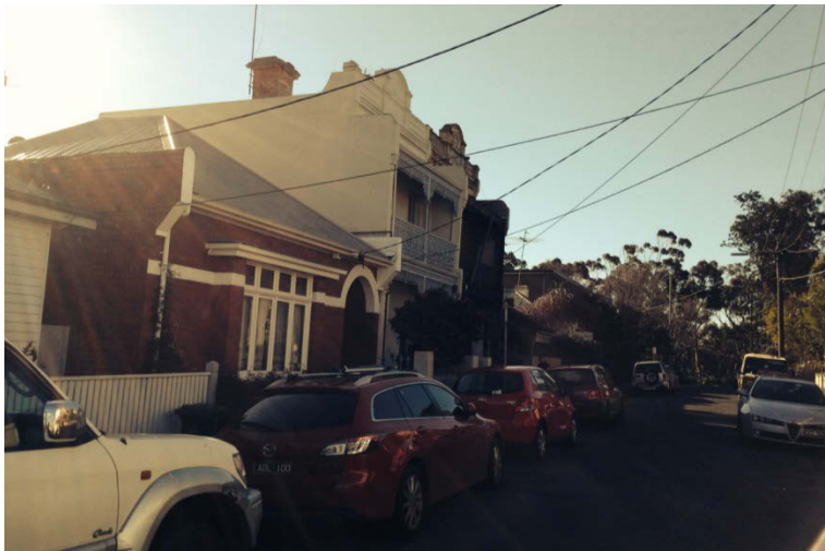
North side of Park Street, looking east, showing the Edwardian house at no. 3 and the double storey late Victorian terrace pair at nos. 5 & 7
