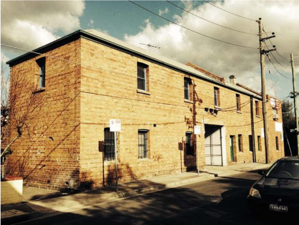
Glasshouse Street elevation looking west (above)
