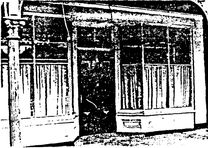
A typical Victorian shopfront with 'lamb's tongue' ogee profile mullions, solayed entry and heavily moulded stallboard.
