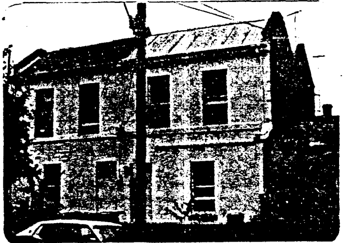
Two storey terrace house with austere detailing. Exposed gable roofs were commonly found on early Victorian residences as was simple fenestration with few decorative mouldings.
