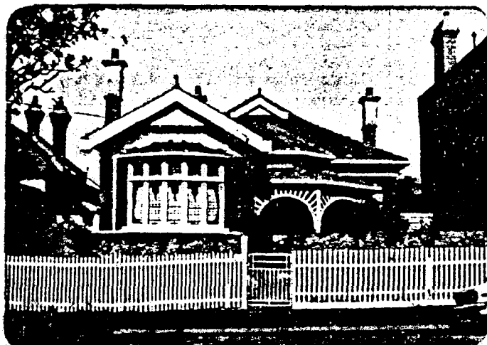
A prominent bow window with leaded glass casements of art nouveau pattern is the feature of this house in Princes Hill. Other typical Edwardian features are the 'sunburst' timber decoration, terra cotta tile roof and clipped privet hedge.
