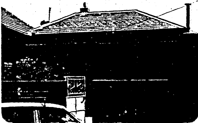
Sadly, most new high masonry walls are badly designed and often poorly executed. Apart from their detraction from the visual qualities of the houses, they detract from the overall streetscape. These three examples demonstrate particular problems; bluestone piers used in a manner entirely foreign to their original use; hollow besser blocks creating a completely inappropriate texture, and materials which clash with the body of the building; and bland brickwork with no articulation and insufficient capping.
