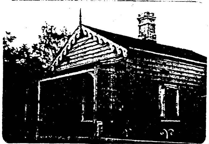
largely confined to institutional buildings. The timber cottage is one of relatively few surviving from the early period. The decorated barge boards drew on Gothic revival precedents and the weatherboards had a typical beaded edge profile.
