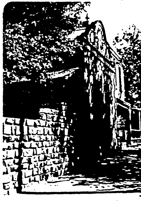
Sadly, most new high masonry walls are badly designed and often poorly executed. Apart from their detraction from the visual qualities of the houses, they detract from the overall streetscape. These three examples demonstrate particular problems; bluestone piers used in a manner entirely foreign to their original use; hollow besser blocks creating a completely inappropriate texture, and materials which clash with the body of the building; and bland brickwork with no articulation and insufficient capping.
