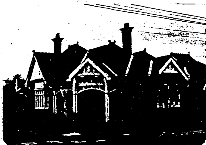
The picturesque arrangement of hips and gables characterise the Federation style of architecture, popular during the Edwardian period. This interest in complex roof forms is highlighted by the use of slate with contrasting terra cotta ridge capping. The use of timber verandah columns and brackets contrasts with the late Victorian predilection for cast iron components.
