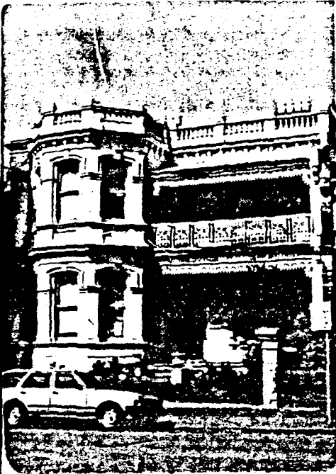
In Princes Hill and South Carlton several larger residences are located, interspersed with rows of much smaller terraces. This example has typical 'boom style' elements such as a large front bay window, heavily modelled surfaces, balustraded parapet and cast iron decoration.
