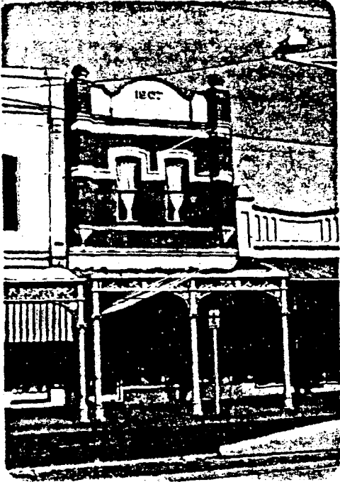
One of several Edwardian shops in North Carlton, this facade has typical red brickwork with contrasting cement render, octagonal brick piers and a simple curved parapet. The cast iron post supported veranda, popular with Victorian shops, was still widely used during the Edwardian period lending a unifying element to shopping areas.
