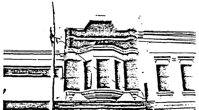
One of Lygon streets few Edwardian shops, this facade has a typical bay window, octagonal piers and simple geometric cement mouldings. The red brickwork is particularly characteristic of this period.
