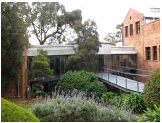
**Figure 2.** The north-west elevation of the 1911 building (right) with its gabled third-storey, the 1984 glazed walkway and the modified 1920s brick office building (left).
