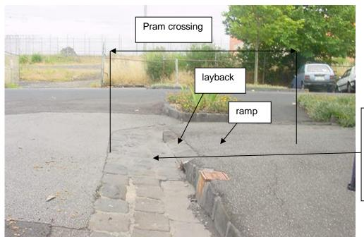
When bluestone pitcher channels at pram crossings are reconstructed the pitchers in front of the pram crossing will be cut in half and laid smooth side up.
