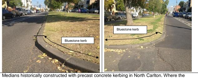
Medians historically constructed with precast concrete kerbing in North Carlton. Where the existing precast concrete end radials are damaged they will be replaced with concrete. If the end radials are bluestone, they will be replaced with bluestone.
