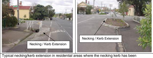
constructed to match the street bluestone kerb and channel.
