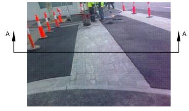
TYPICAL SAWN BLUSTONE PAVERS PAVING AT TRAFFIC MANAGEMENT DEVICE.
