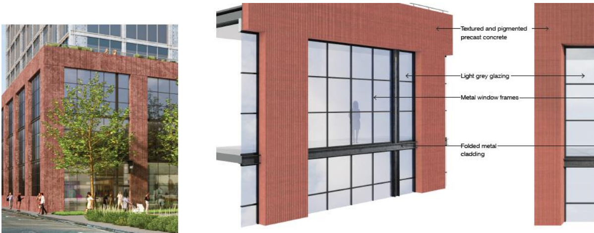
Figure 20: Building D (Chestnut workplace) streetwall detail Source: Denton Corker Marshall
