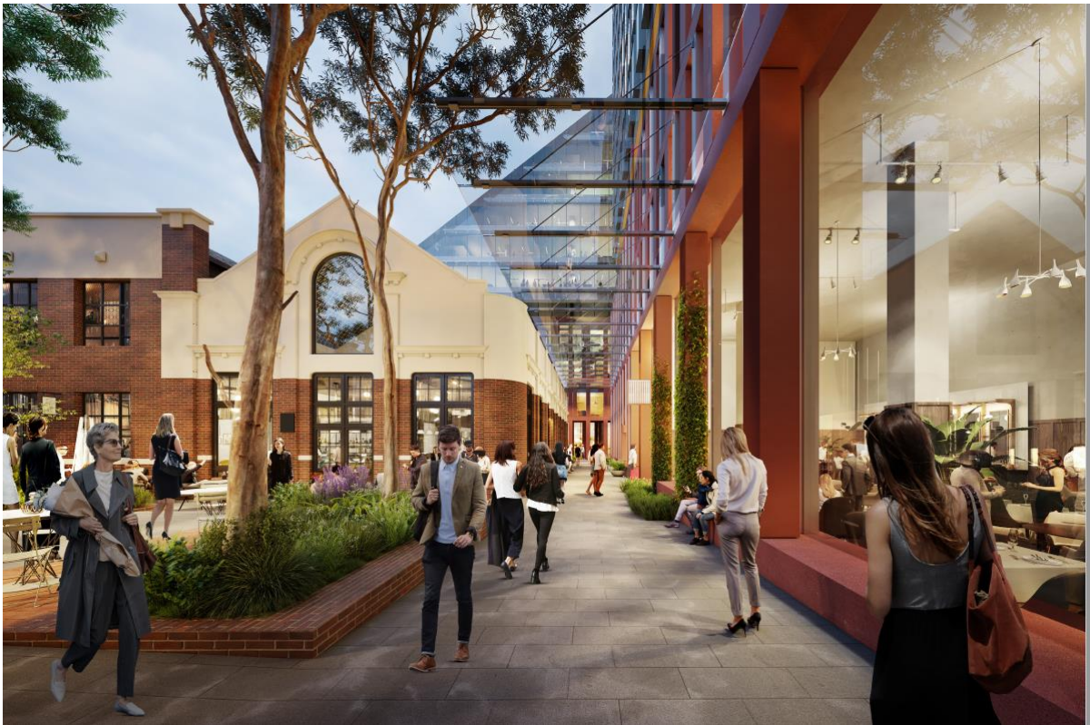
Figure 38: Looking west down Hotham Place towards Building C (Building B to the right and red head green to the left) Source: Denton Corker Marshall
