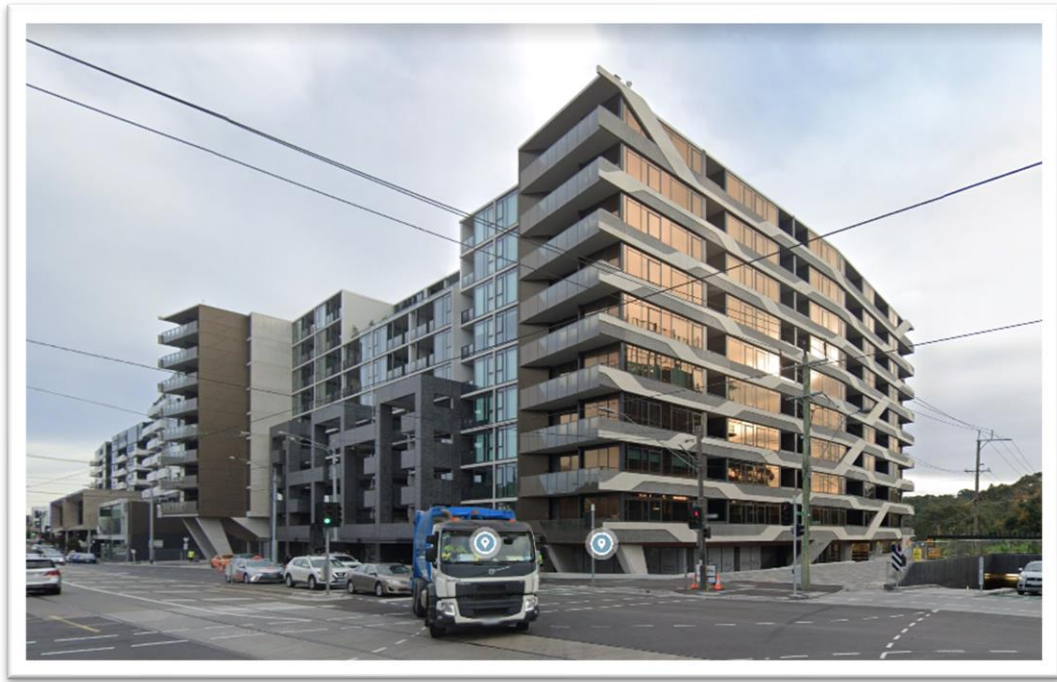
Figure 15: Built form to the north-west. Source: Planning Officer Report, Council Meeting 14 March 2023.
