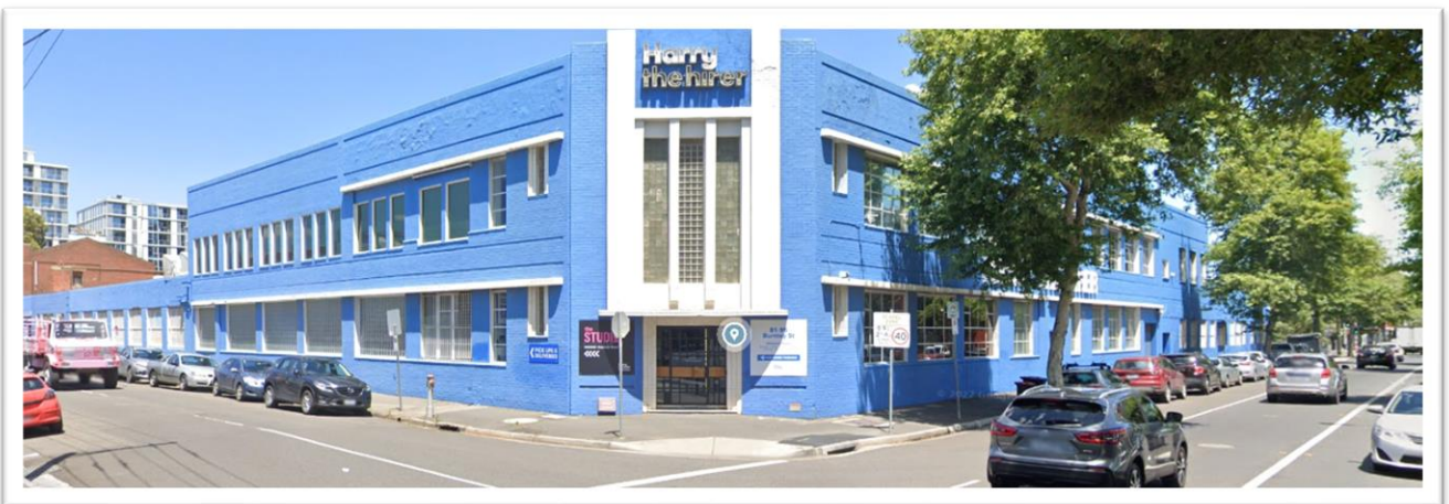
Figure 9: Russell Manufacturing Co. building (81-95 Burnley Street). Source: Landscape Plan (TCL 2023)
