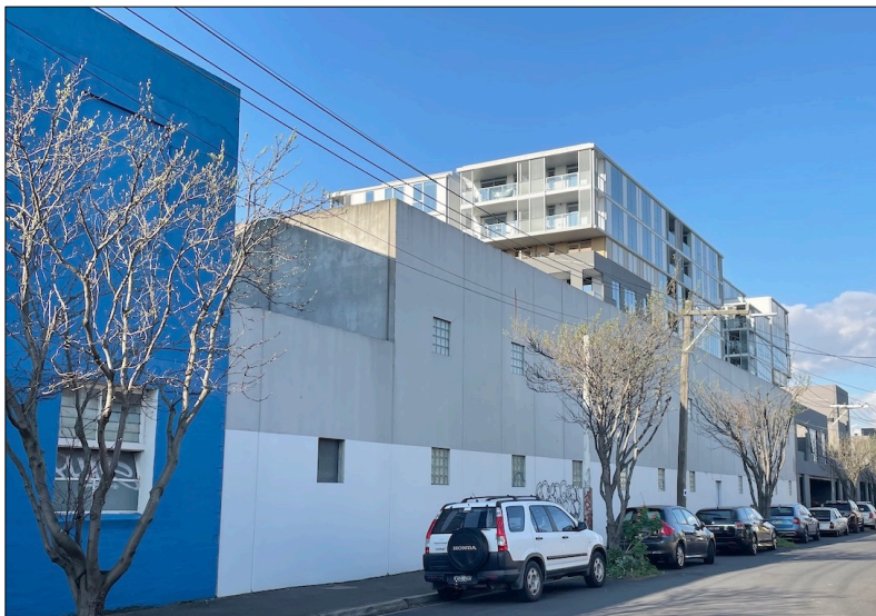
Figure 11 The Appleton Street frontage to the subject site showing modern tilt up concrete building with multi-storey development on the adjacent site in the background.
