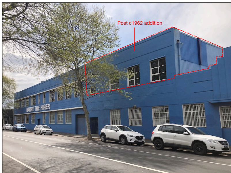
Figure 9 The Burnley Street façade.
