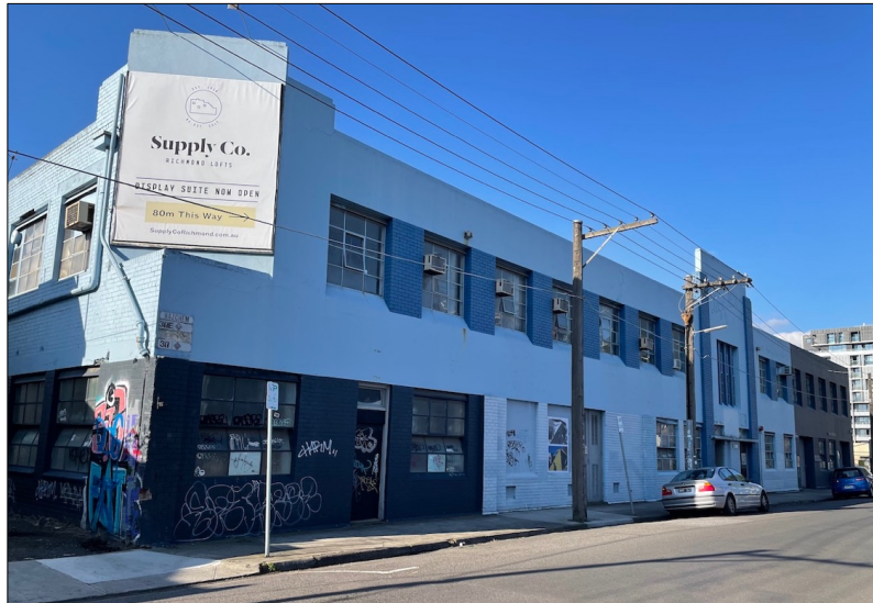
Figure 15 Double-storey interwar former factories on the north side of Doonside Street, opposite the subject site.
