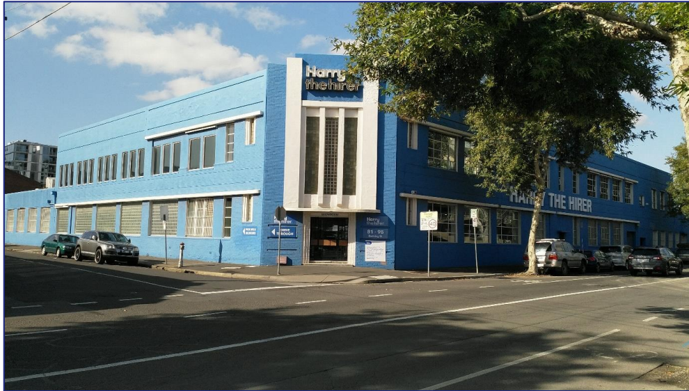
Figure 1: Subject Site – Burnley Street/Doonside Street corner
