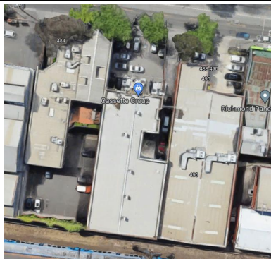
Figure 9: No. 488 - 490 Swan Street, Richmond – Aerial view (Image extracted from Google – Image Capture September 2022).
