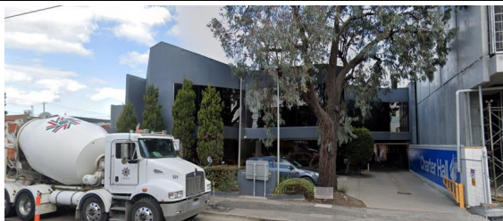
Figure 6: No. 484 Swan Street, Richmond – Street view (Image Google – Image Captured September 2022).
