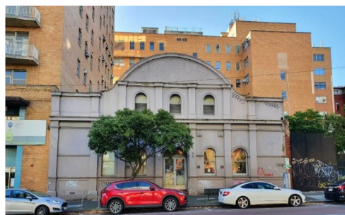
Figure 12 – Brennan Hall viewed from Victoria Parade (Source: Planning Officer photo, May 2021).
