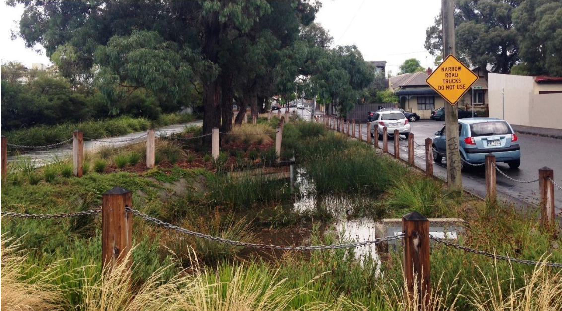
Apperly St Sediment trap
