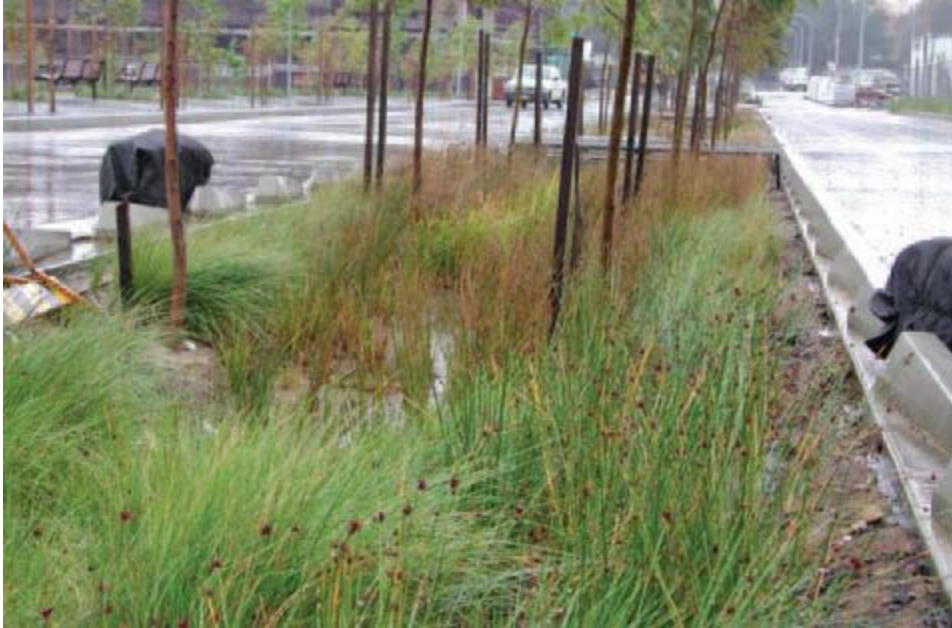
Centre median vegetated swale – landscape feature, stormwater treatment and some local detention.
