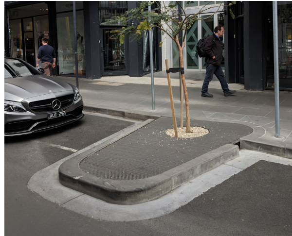
2. Grated tree pit
