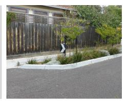
Trees can be located immediately upstream of standard kerb inlets to ensure runoff enters tree pit before entering stormwater network
