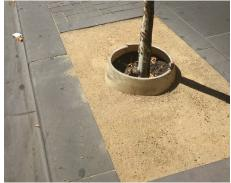
Porous asphalt, No fines concrete
