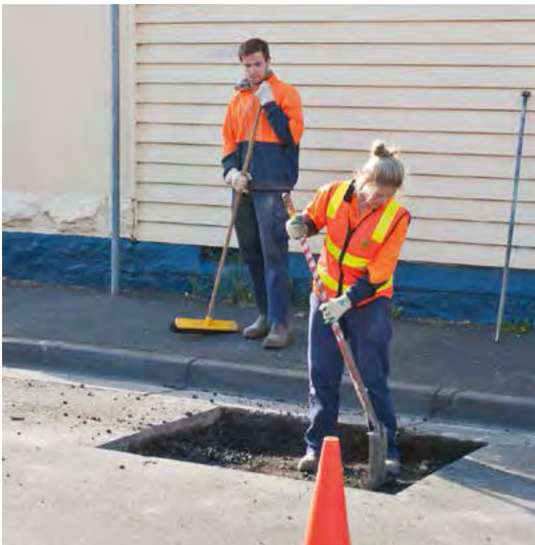
Left: Making room for another street tree.
